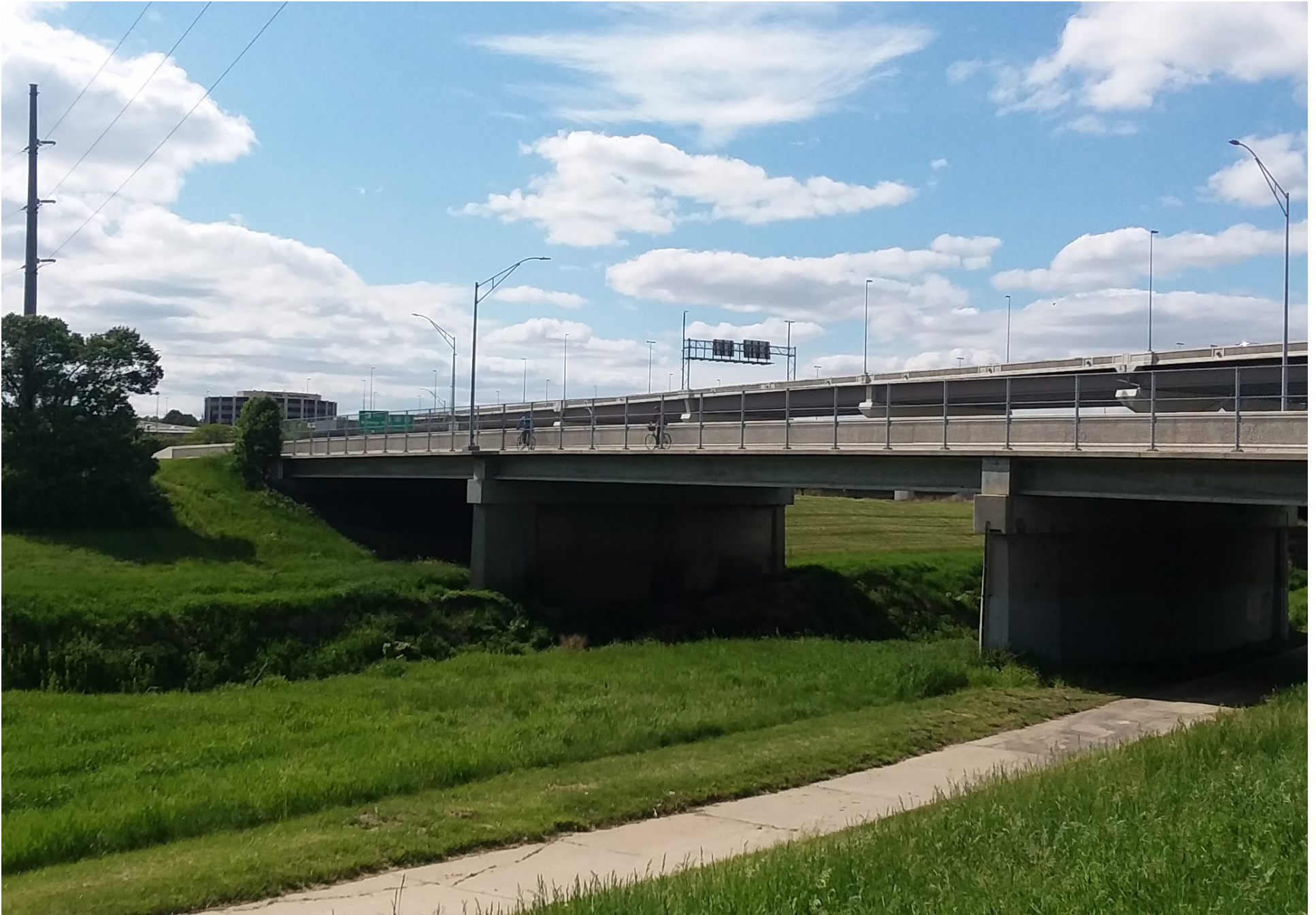
W Dodge Frontage Road Bridge
