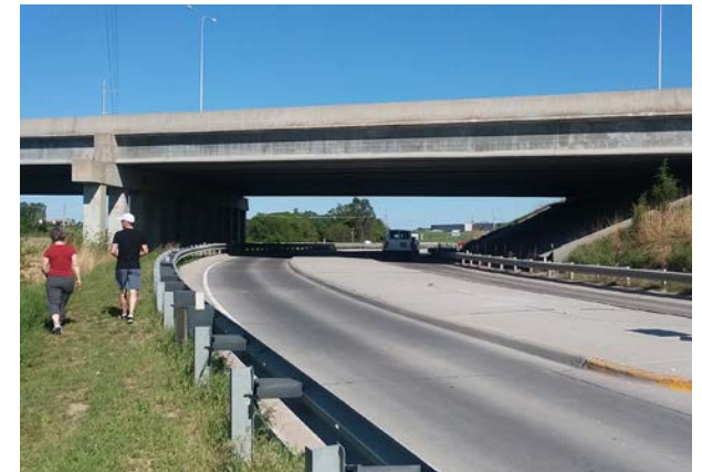
Bridge Underpass, Giles Rd.
