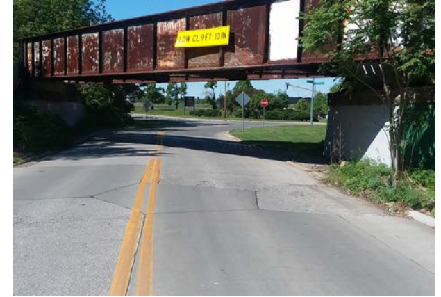
Narrow Railroad Bridge Underpass, Florence Blvd.
