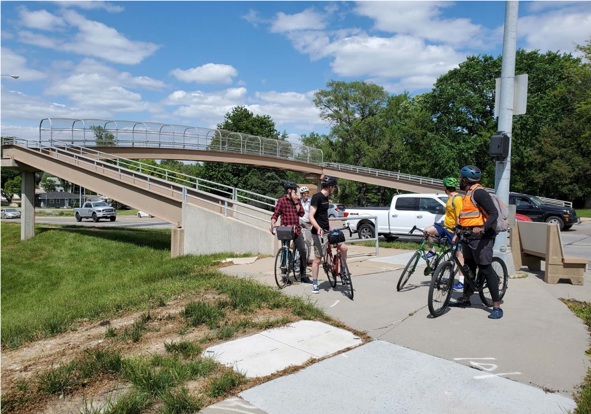
90th Street Pedestrian Bridge
