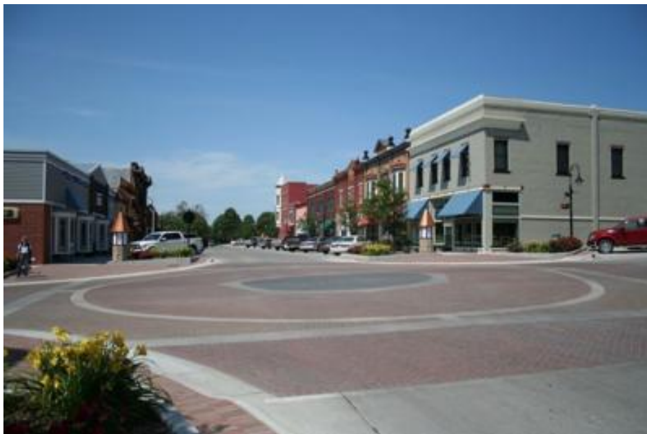
Figure 2.1: Downtown Avoca has seen reinvestment in their downtown, including numerous streetscape improvements.
