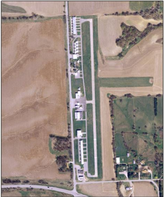
Figure 8-12: Aerial Photograph of the North Omaha Airport
