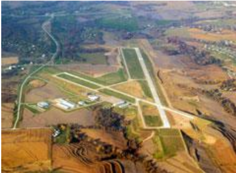
Figure 8-11: Aerial Photograph of the Council Bluffs Airport
