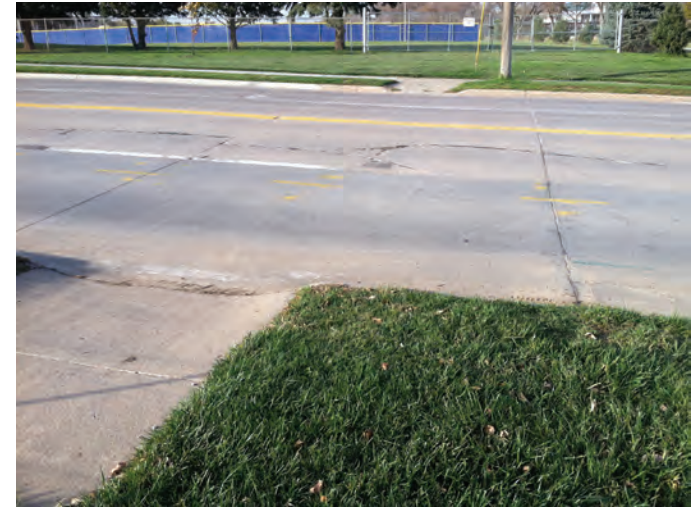
The mid-block crossing does not include street markings, signage or signals alerting drivers and pedestrians of a crossing point.
