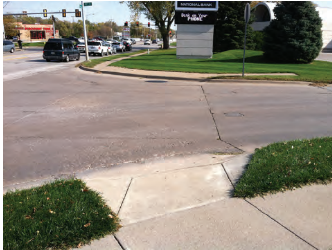
While a curb ramp is provided on the near side of the street, the lack of a ramp on the far side prohibits accessible crossing.
