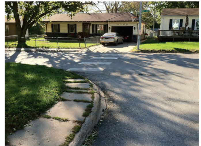
The near sidewalk needs widening, repair, extension and a curb ramp to accommodate crossing.
