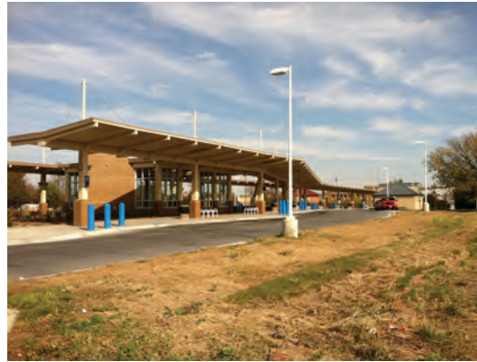
Figure 32: Photos of the recently-renovated North Omaha Transit Center
