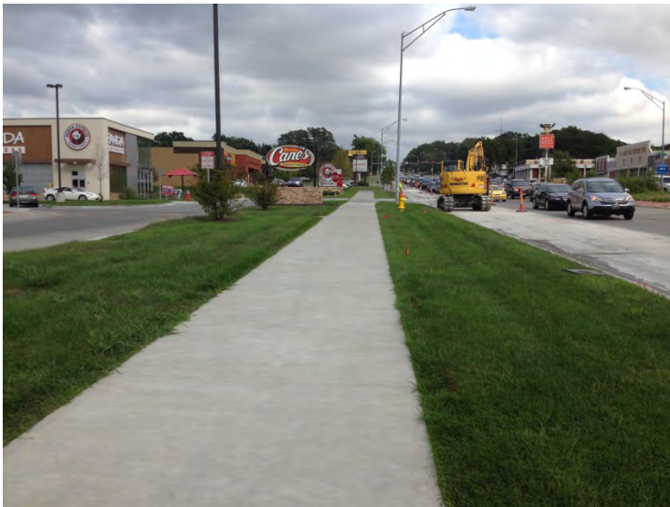
New sidewalk on the north side of Dodge is an (slight) improvement to
