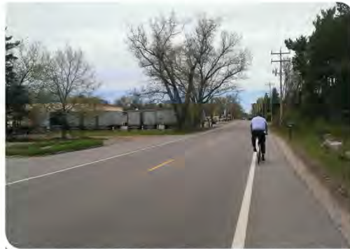
Wide paved shoulders reduce run-off-road crashes, improve roadway maintenance, and can provide space for bicyclists.
