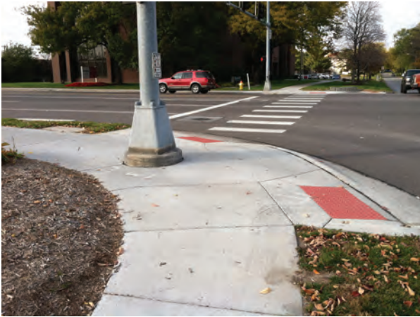
The traffic signal pole is aligned to hinder movement along the sidewalk and without proper setback from the curb ramps.
