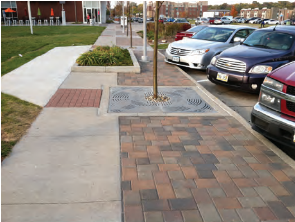
The low planter obstructs the sidewalk.
