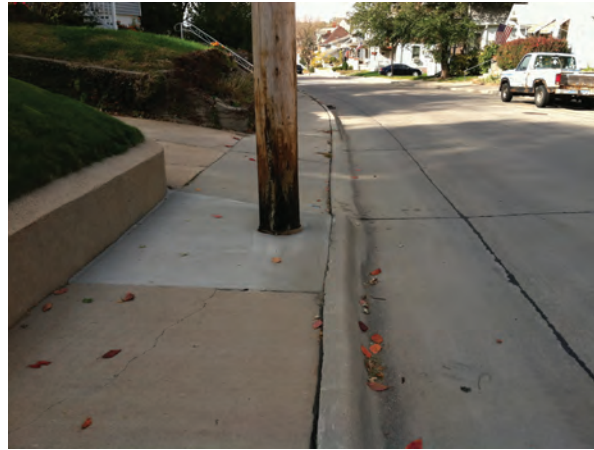
The street light pole is located on the sidewalk and obstructs accessible clearance along the path.
