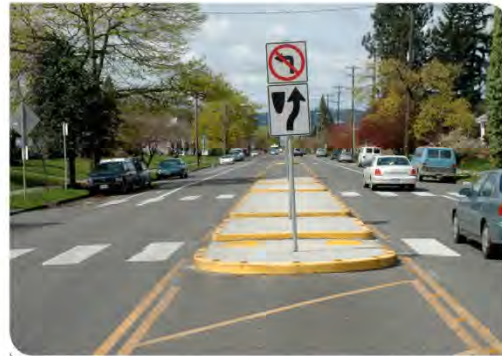
This crossing island doubles as a partial diverter. Curb ramps are “cut through,” allowing pedestrians to remain at-grade.
