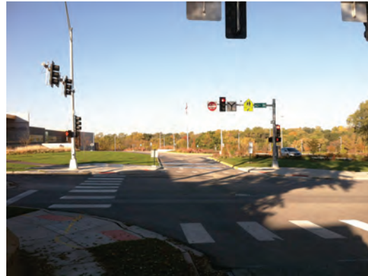
Figure 28: Traffic lights and signals provided with access-prohibited signage for vehicles (left). Landscaped medians, street trees and crosswalk markings (right)
