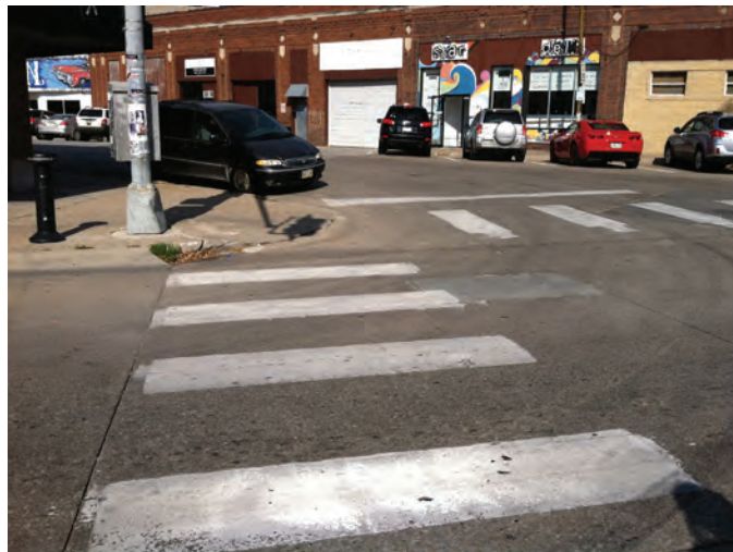
The alignment of the crosswalks is not advantageous as they do not meet the sidewalk at a proper setback from the cross street.
