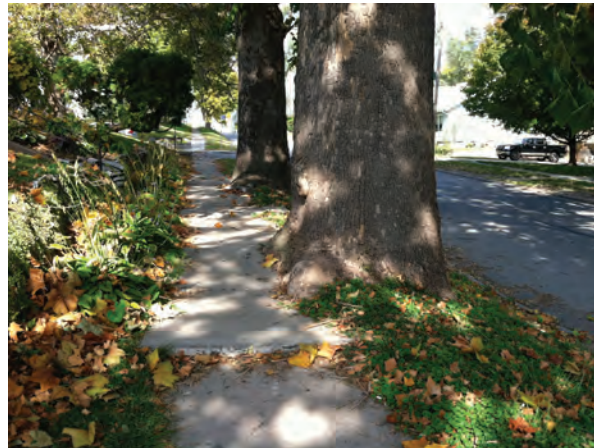
The street trees' trunks have grown into the sidewalk while their roots have raised a portion of the concrete, creating a tripping hazard for pedestrians.
