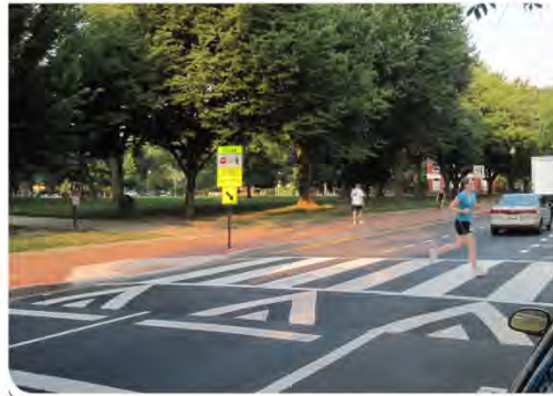
Raised crosswalks have traffic-calming effects. This crosswalk crosses two travel lanes, a bike lane, and a parking lane.
