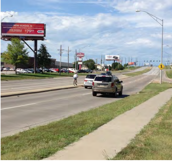
Cyclist trying to cross 132 nd mid-block because there were no sidewalks on the west side of the street
