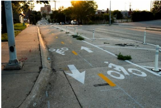
Figure 4: Two-Way Cycle Track on Harney Street
