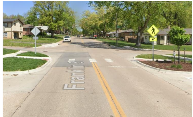
Figure 6: Curb Bump-outs on Franklin Street
