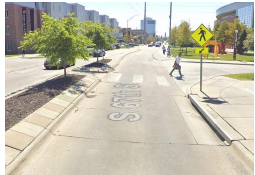
Figure 5: Protected Crossing with Pedestrian Refuge on South 67th Street
