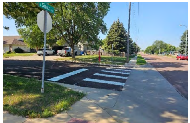
Figure 4: Continental Crosswalk with Curb Ramps
