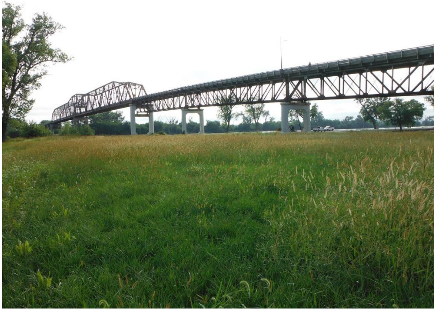
Photograph 3. View southeast toward the Bellevue Bridge. Bellevue Bridge is a continuous truss bridge over the Missouri River connecting Mills County, Iowa and Sarpy County, Nebraska near the city of Bellevue, Nebraska.
