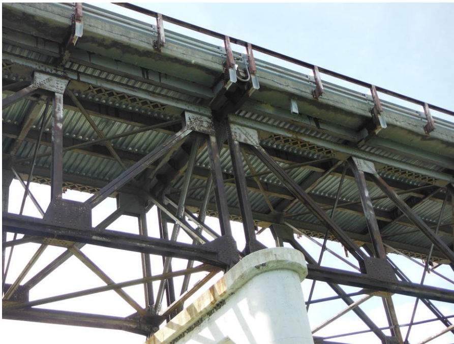
Photograph 4. View toward the bridge support substructure, which are painted. Paint on the materials used during the time of the bridge's construction may have contained lead-based materials. A lead inspection may be needed if paint removal or disposal is necessary.
