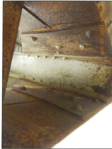
Span 3 L6L7 Lt plate deterioration at L7
