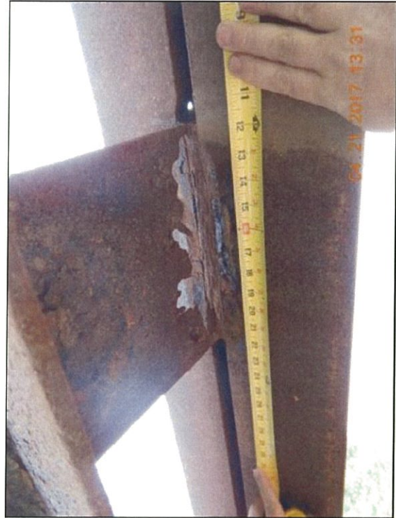
Span 1 L1L2 Lt bottom exterior angle hole below middle batten plate
