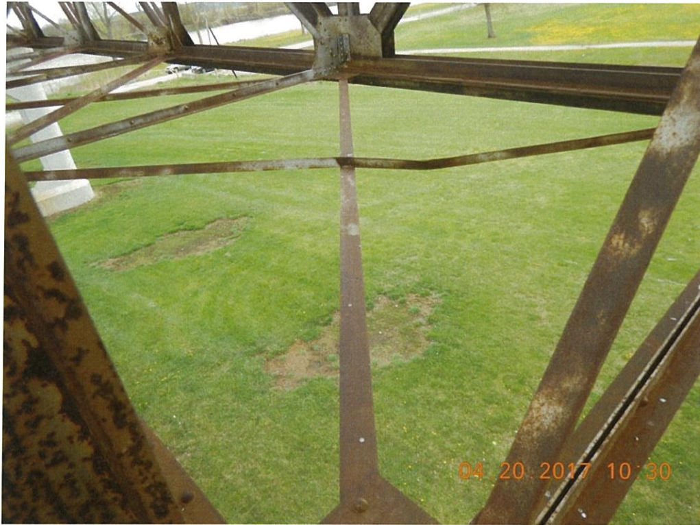
Photo 65: Deck truss lower lateral bracing is bent at Span 2 Bay 5.
