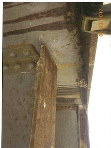
Span 5 Floorbeam 5 bottom flange bird debris
