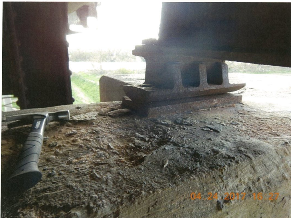
Photo 110: Both anchor bolts of Span 9 Girder 1 are sheared at the top of the slot at the Pier 8 bearing.
