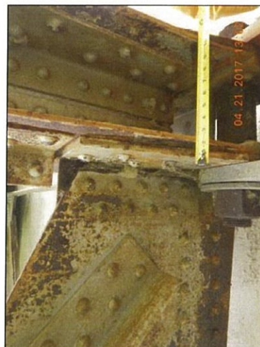
Span 1 L0 Lt bottom interior packrust
