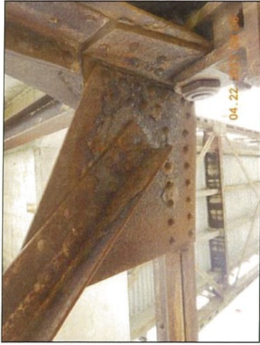
Span 4 L10 Rt horizontal gusset plate deterioration on bottom
