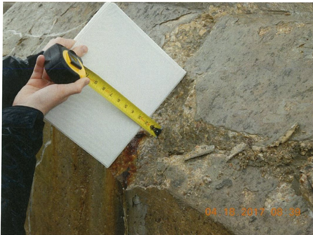
Photo 129: The top of the Pier 8 bottom wall is scaling which is creating spalls around some of the cracks; larger spalls are present at the southwest corner and east faces of the wall. Close up of largest spall on east face shown.
