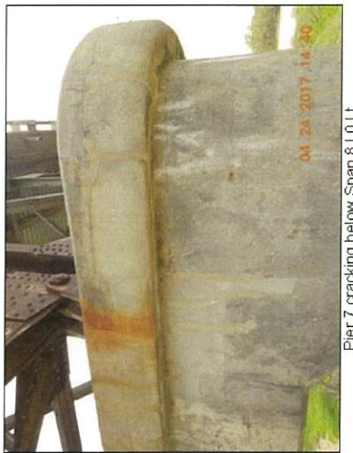
Pier 7 cracking below Span 8 L0 Lt
