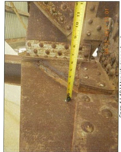
Span 4 L10 Lt top interior packrust
