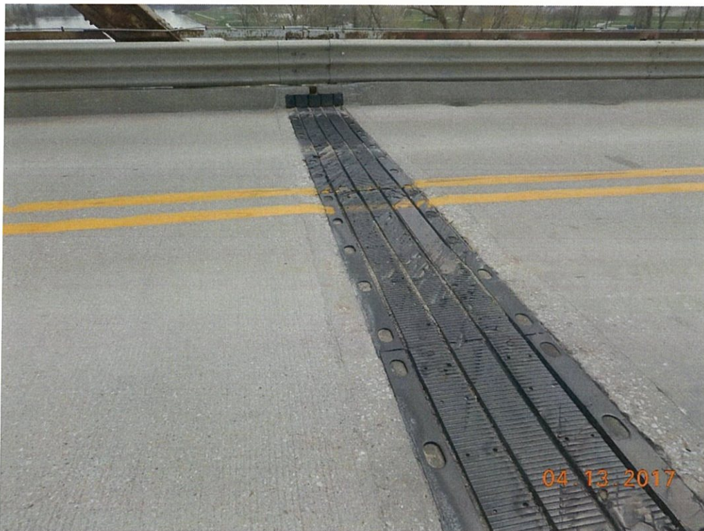
Photo 16: Both of the transflex joints have plow damage consisting of surface damage of the molded rubber and minor spalling of the adjacent concrete.
