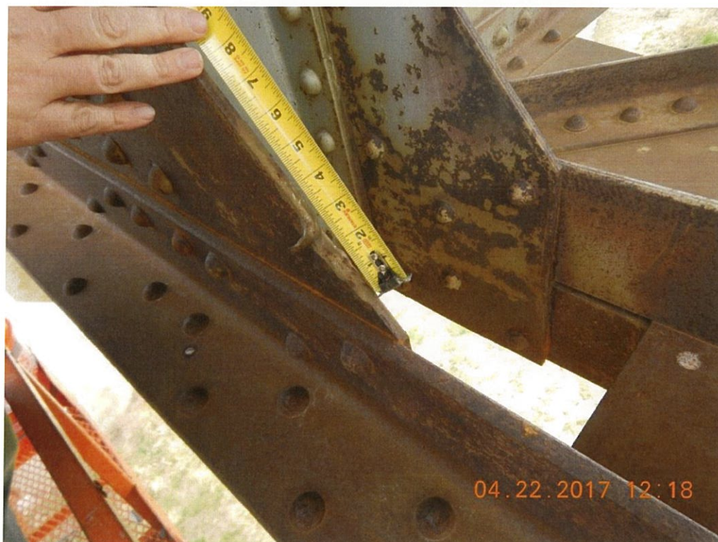
Photo 50: The Span 4 L7 Lt. exterior gusset plate has a minor tear.
