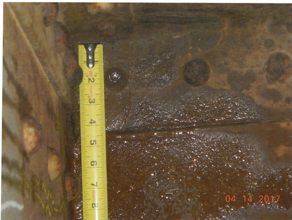
Photo 76: The packrust has broken rivets in several locations of the thru truss lower chords. Span 6 L6'L7' Lt. at L6' shown.
