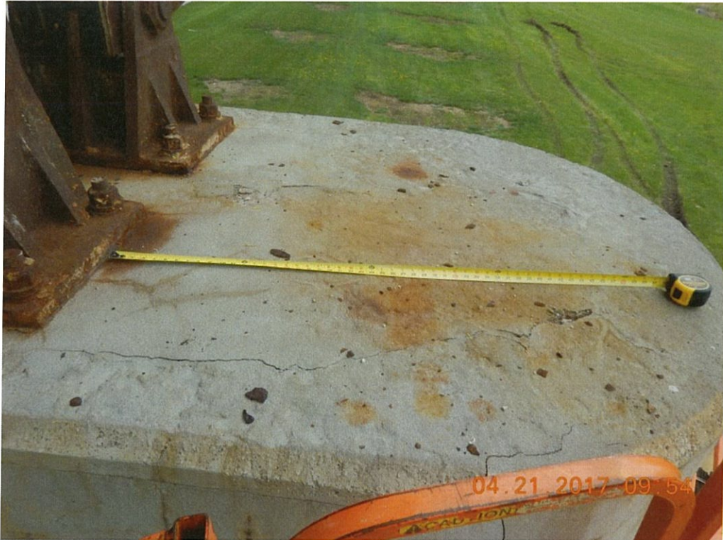
Photo 119: The top of the Pier 1 cap has minor sealant coat deterioration with plain sand underneath it near the center; similar at the south end with cracks forming - shown.
