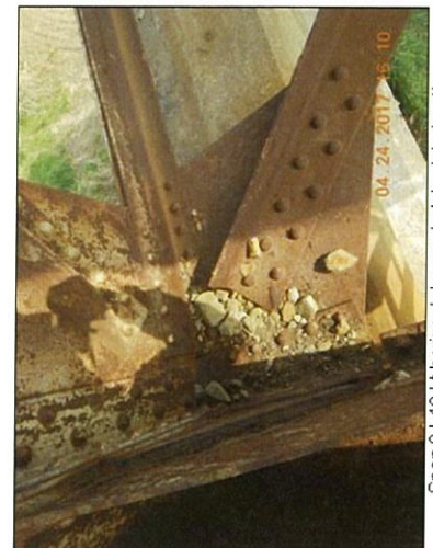
Span 8 L10 Lt horizontal gusset plate deterioration
