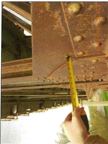
Span 8 L0 Rt top exterior packrust
