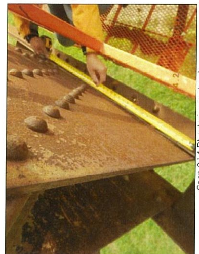
Span 8 L1 Rt exterior packrust
