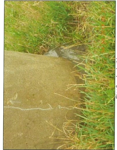
Pier 8 water buildup
