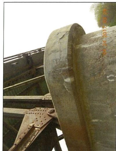
Pier 7 South end West face of cap deterioration
