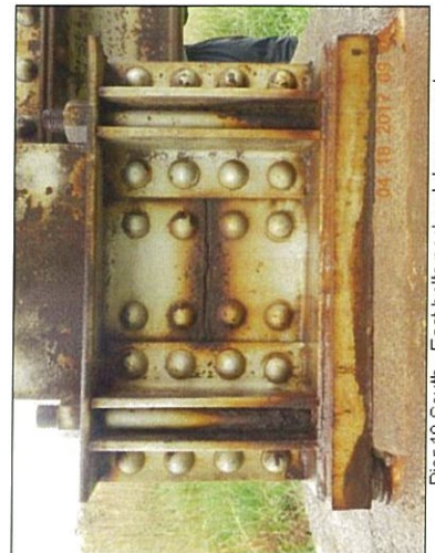
Pier 10 South - East bolts packrust, typ on west
