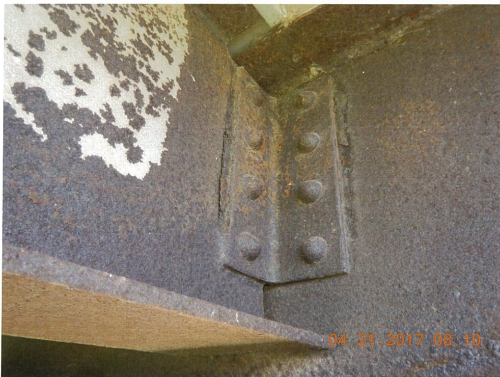
Photo 58: Minor packrust has developed between the deck truss floorbeam web and exterior stringer connection angle at some locations throughout. Span 2 Stringer 4 at Floorbeam 8 shown.
