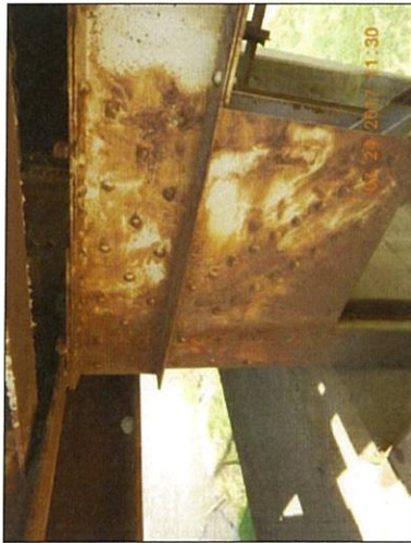
Span 7 U0 Rt exterior deterioration
