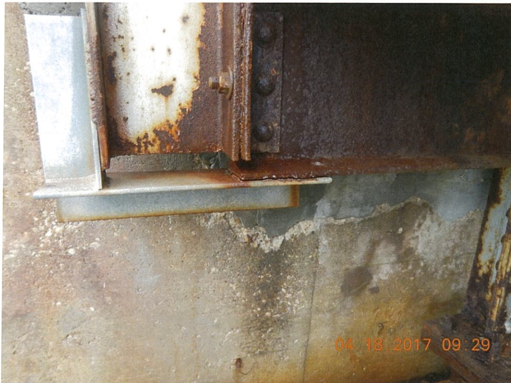
Photo 17: The bottom connection weld of the northeast rail at Abutment 2 is cracked at the beam; the rails are bolted into the deck and connected to the beam with bolts and angles.
