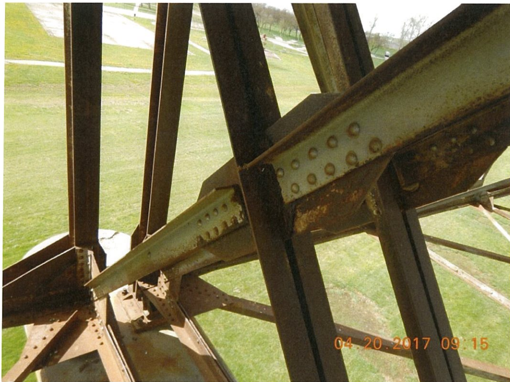
Photo 63: Packrust is developing at the center of the deck truss bracing; the worst is typically in the vertical plane bracing at the ends of the spans. Span 3 L0 end shown.
