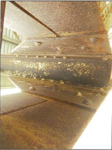
Span 3 L6L7 Lt at L7 packrust and loss
