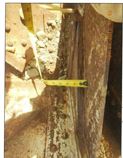
Span 8 L10 Lt top interior packrust
