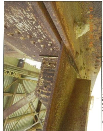
Span 3 L2 Rt horizontal gusset plate packrust on bottom
