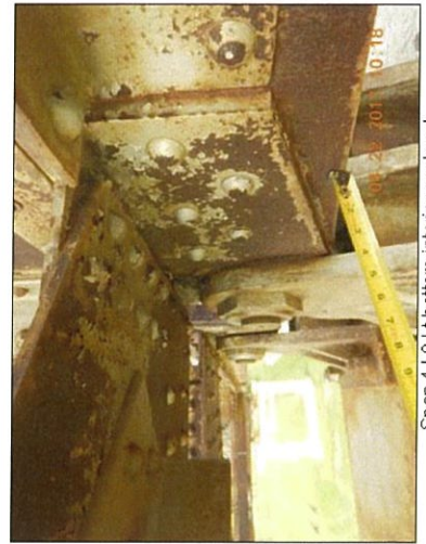
Span 4 L0 Lt bottom interior packrust
