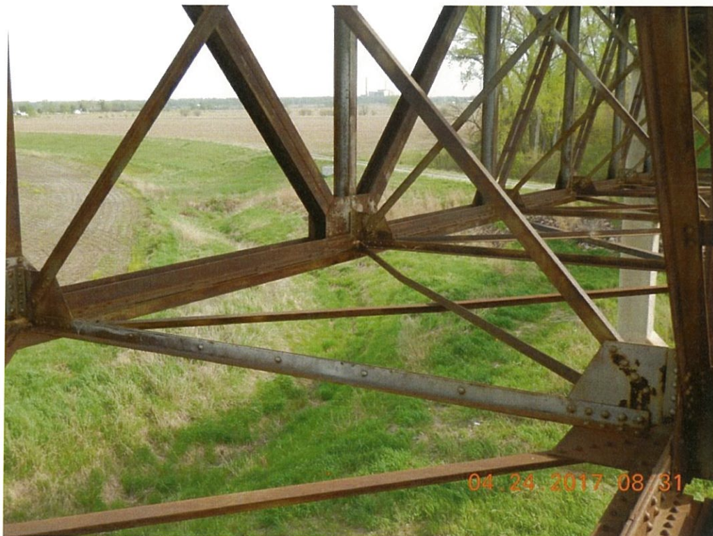
Photo 70: Deck truss lower lateral bracing is bent at Span 8 Bay 5.
