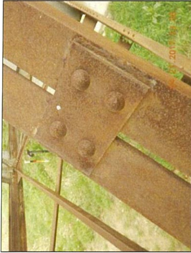
Span 1 U1L2 Lt batten plate deterioration
