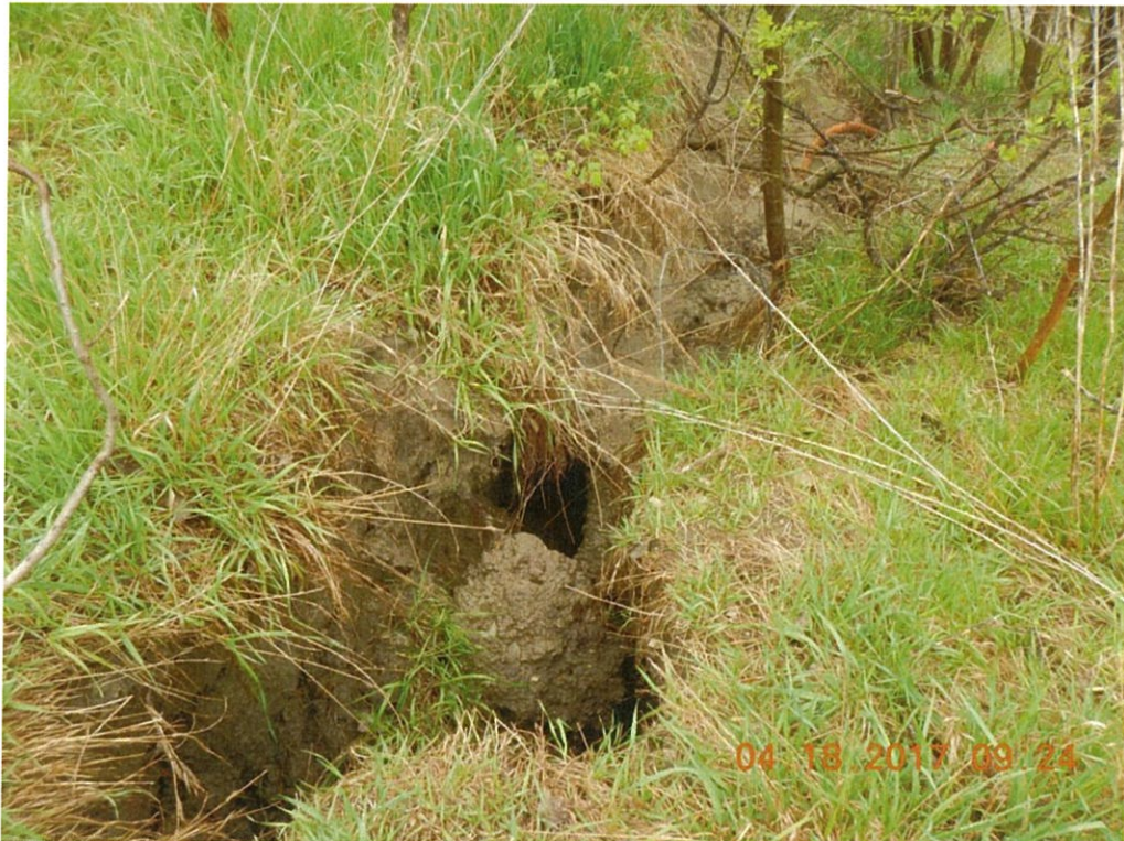
Photo 134: The undermining at the northeast corner of the east approach has previously created a 2' deep embankment erosion channel. The channel is now between 4' and 5' deep.
