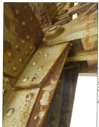
Span 7 L10 Lt bottom interior packrust
