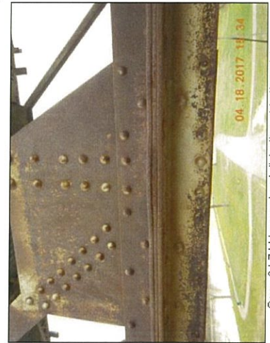
Span 3 L7 Lt lower chord distortion at batten plates
