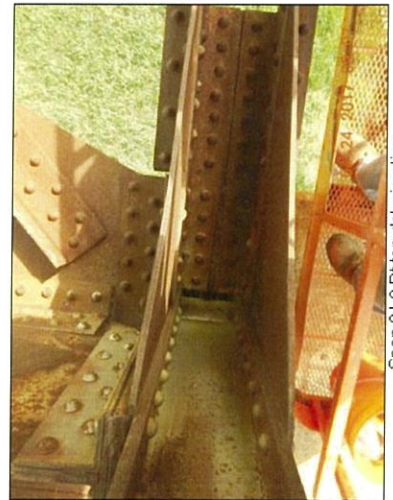
Span 8 L0 Rt top deterioration
