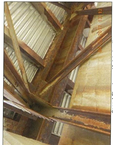
Span 4 Floorbeam 10 deterioration
