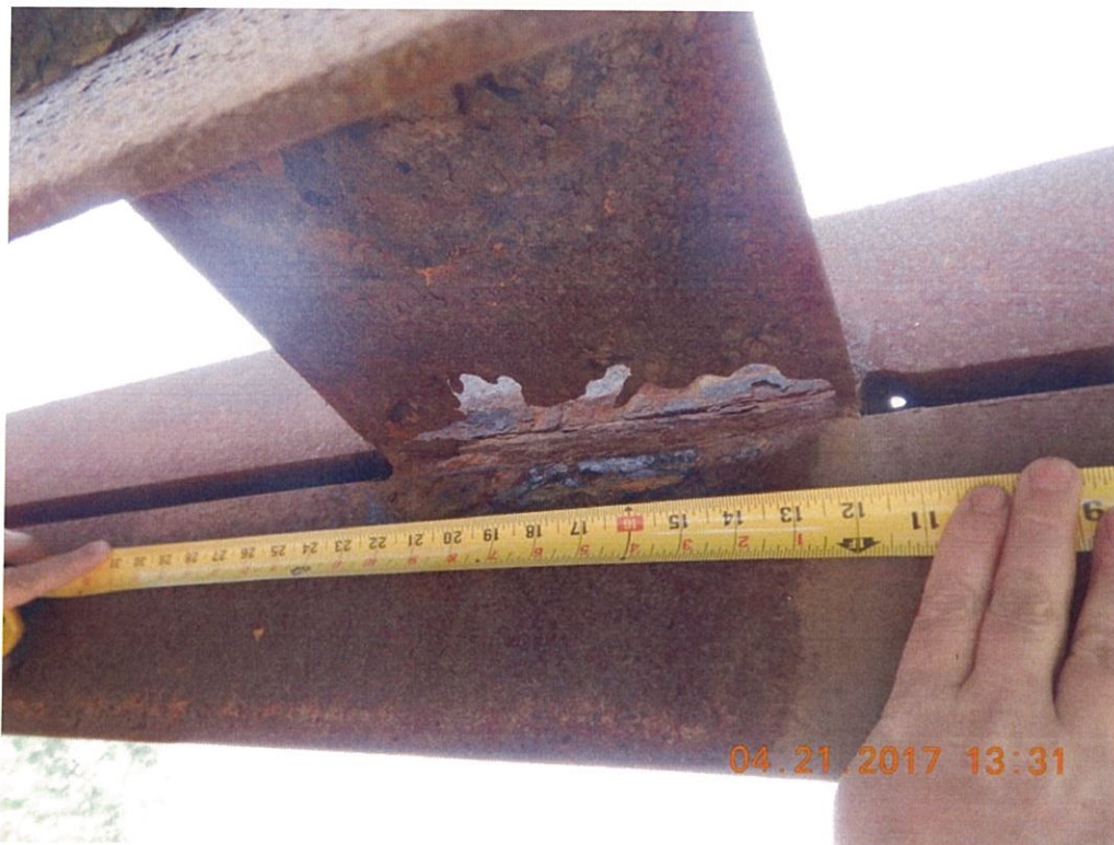
Photo 26: The worst case of the deck truss lower chord loss is at the middle batten plate of Span 1 L1L2 Lt. Complete section loss in the exterior angle for approx. 5" in length and 1" in depth.
