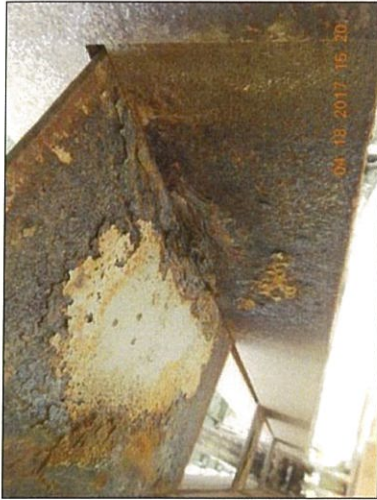
Span 3 L9L10 Lt batten and lower chord deterioration near L9
