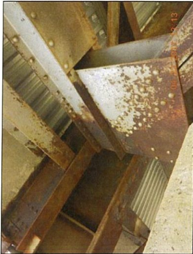
Span 4 U10 Lt exterior deterioration
