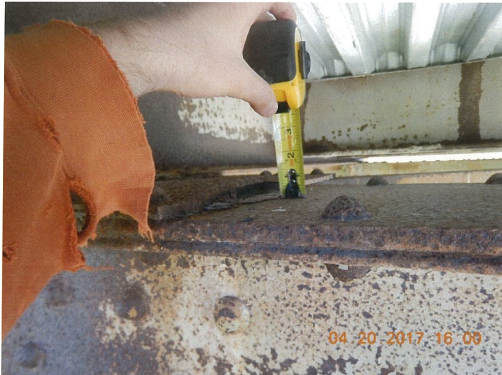
Photo 39: Heavier packrust up to 1" is typical at the deck truss upper chord cover plates below the floorbeam where only two rivets are present instead of four. Span 3 U3 Rt. shown.
