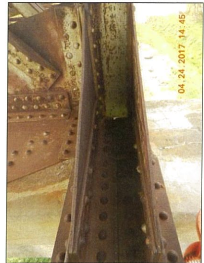
Span 8 L0 Lt top deterioration
