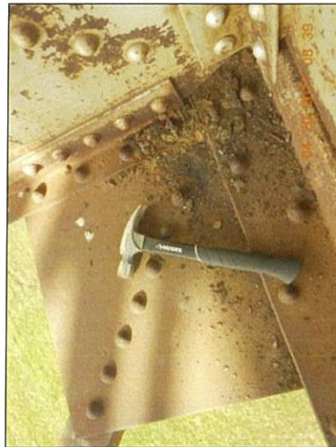
Span 3 L2 Lt horizontal gusset plate deterioration
