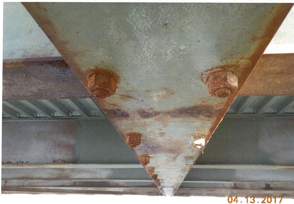
Photo 87: The thru truss lower lateral bracing gusset plates have corrosion and packrust; the L1' and L2' have significant section loss with holes forming. Span 6 L1' Lt. shown.
