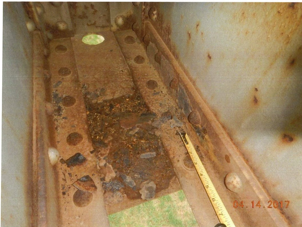
Photo 78: Span 6 L3' Rt. has flaking corrosion of the exterior bottom angle; when removed pitting is up to 1/8" deep in the vertical leg of the angle.
