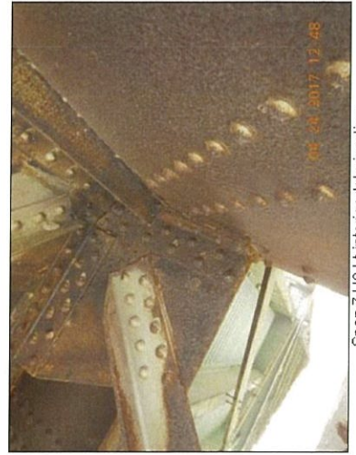
Span 7 U0 Lt interior deterioration
