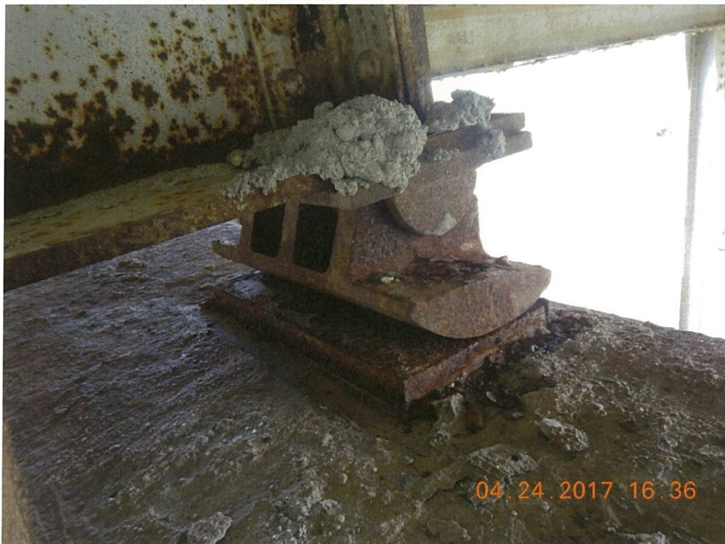
Photo 112: Both anchor bolts at Span 9 Girder 3 are sheared at the top of the slot at the Pier 8 bearing.
