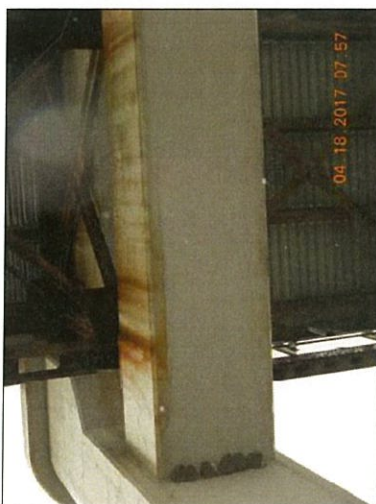
Pier 4 bottom of strut cracking
