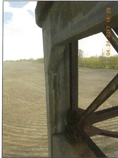
Pier 8 south interior face deterioration
