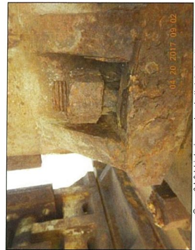
Span 3 L0 Lt interior anchor bolt deterioration
