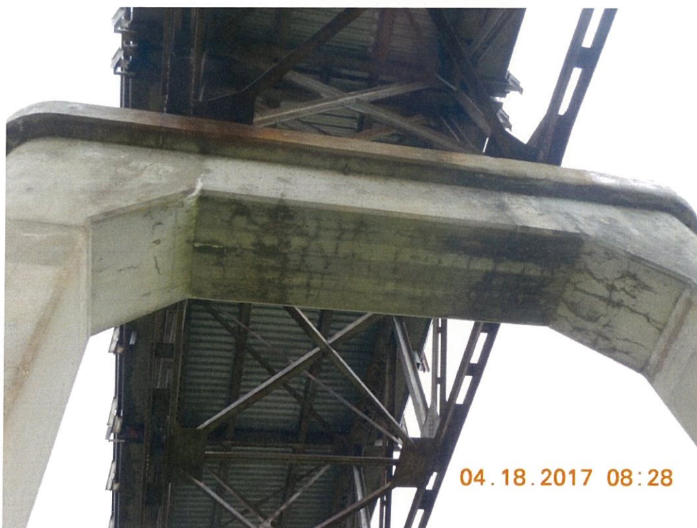
Photo 126: Efflorescence is present at the bottom corners of the Pier 7 cap. It is also present at the top ends of the cap and the east face of the bottom wall.
