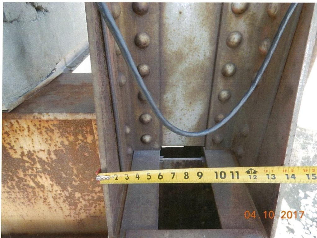
Photo 74: Packrust is present at most lower gusset plate connections of the thru truss spans.
