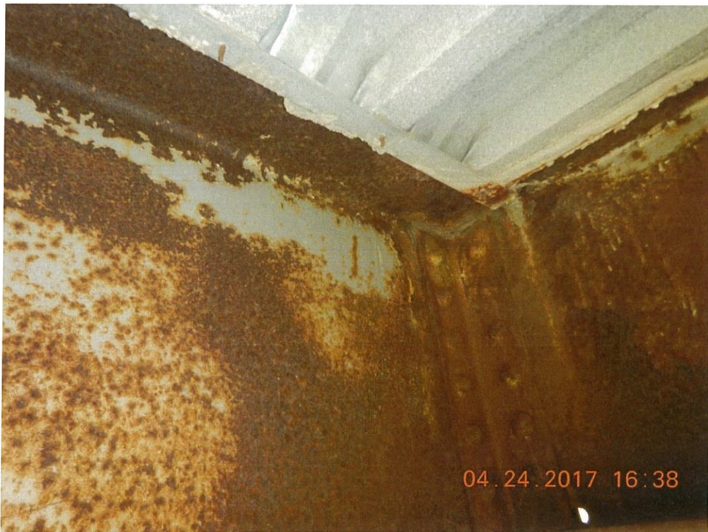
Photo 100: The leaking joints at above the ends of the girders have caused heavy rust with some section loss in the girder webs. Girder 4 interior face at Pier 8 shown.
