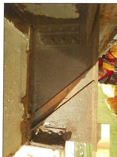
Span 4 Floorbeam 2 Rt stiffened and hole
