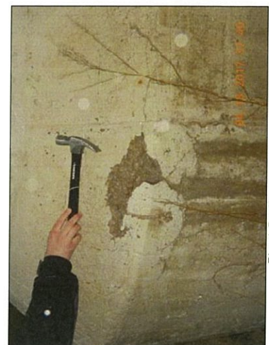
Pier 1 Southeast spall at bottom
