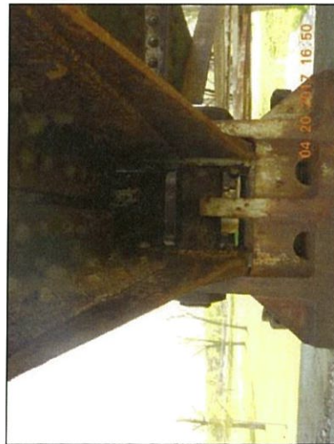
Span 3 L0 Rt bottom plates bowed inward
