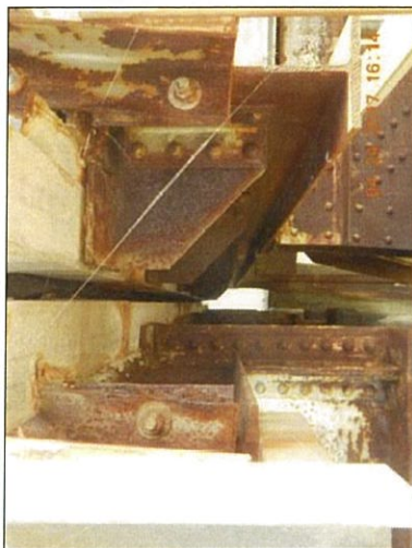
Span 8 Floorbeam 0 Lt deterioration below deck joint
