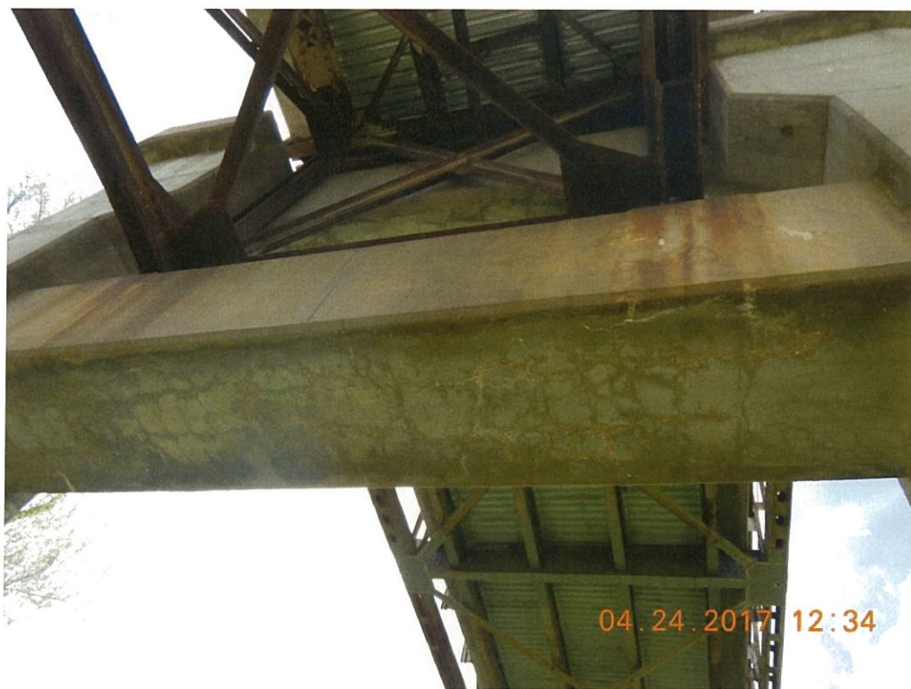
Photo 125: Minor efflorescence on the Pier 6, Span 7 cap.
