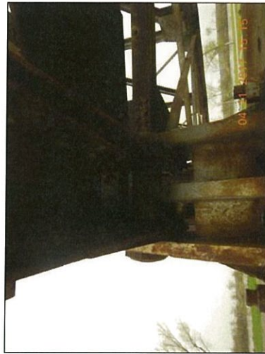
Span 1 L10 Lt gusset plates bent inward
