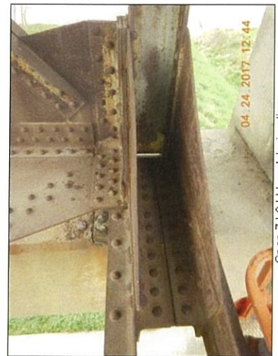
Span 7 L0 Lt top deterioration
