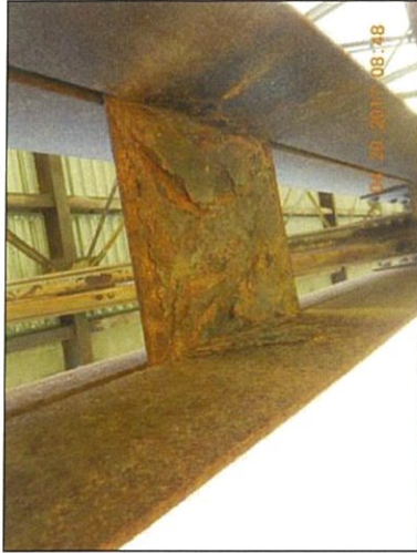
Span 3 L1L2 Lt 2nd batten plate deterioration
