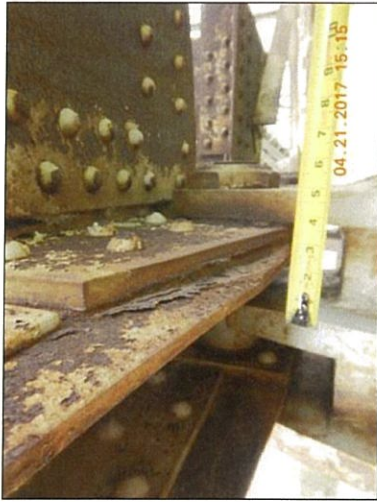
Span 1 L10 Lt bottom interior packrust
