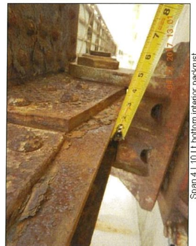
Span 4 L10 Lt bottom interior packrust (2)
