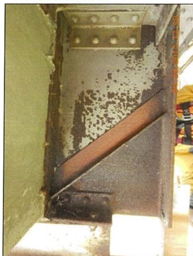
Span 7 Floorbeam 1 Lt stiffened and hole
