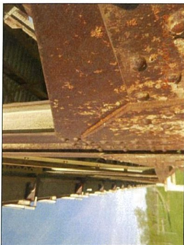
Span 4 L0 Rt top exterior packrust
