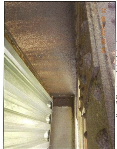
Span 3 Floorbeam 2 Lt deterioration
