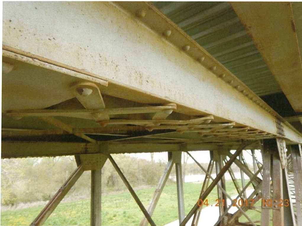
Photo 47: Small dents are present at some locations throughout the deck truss. These dents were most likely created during construction. Span 1 U7U8 Rt. lacing near L7 shown.
