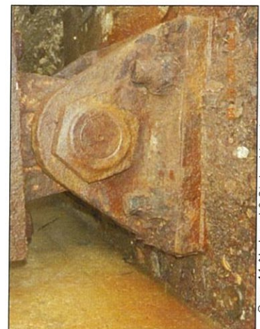
Span 11 Abutment 2 Girder 1 bearing looking North - interior nuts and bolts deterioration
