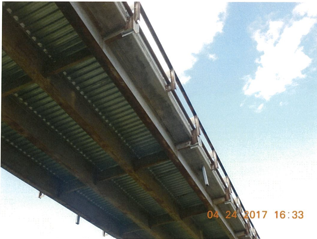
Photo 9: Transverse cracking with efflorescence is present randomly throughout the overhangs of Spans 9 through 11. South overhang of Span 9 shown.
