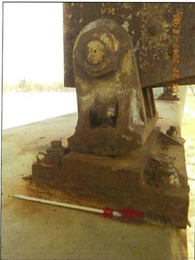
Span 4 L10 Lt rocker shifted east from exterior
