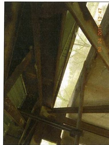
Span 7 Floorbeam 0 interior deterioration (3)
