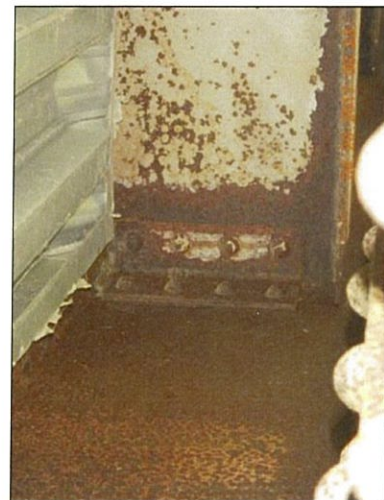
Span 3 Floorbeam 4 Stringer 2 exterior packrust
