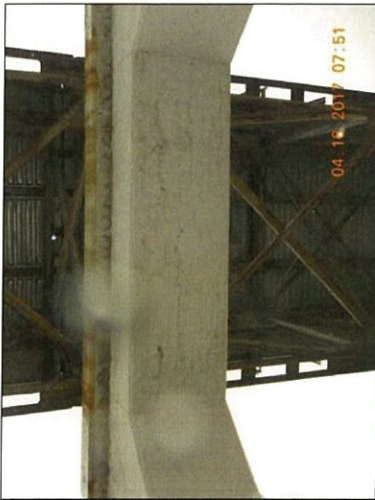
Pier 3 cracking on bottom of strut
