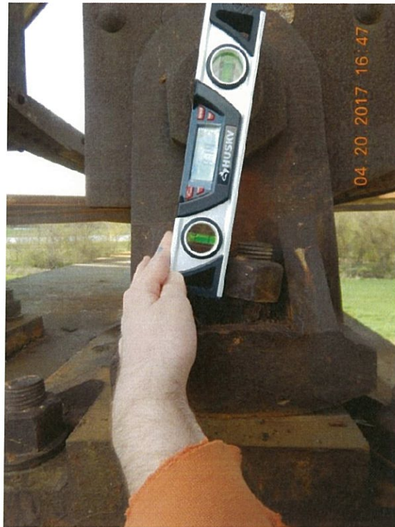
Photo 106: The deck truss anchor bolts at expansion bearings have delamination in the threads between the nut and the bearing plate; the slots are filled with debris causing some of the bolts to bend. Span 3 L0 Rt. exterior bolt shown.
