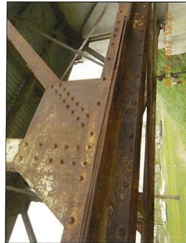
Span 1 L2 Lt exterior heavy deterioration
