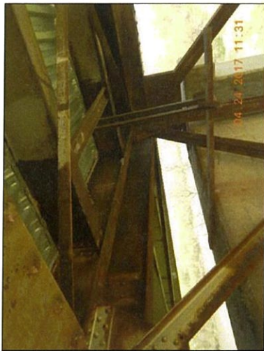
Span 7 bracket at Floorbeam 0
