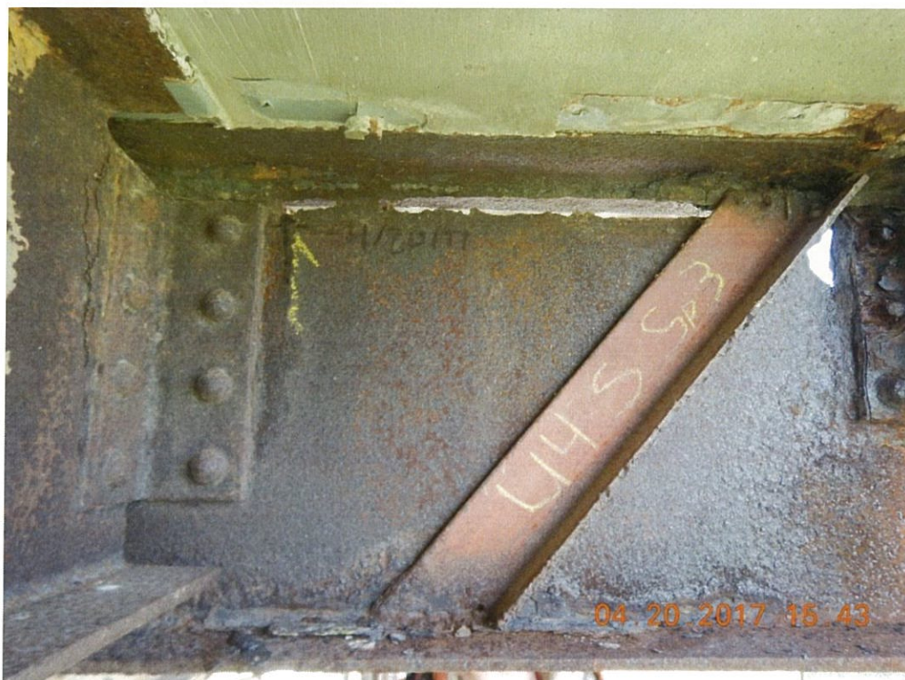
Photo 60: Most of the locations shown in Photo 59 have been retrofitted with steel angles to strengthen the weakened web. Span 3 Floorbeam 4 Rt. shown. This location has the worst section loss with extended growth towards the stringer clip angle since last being marked.
