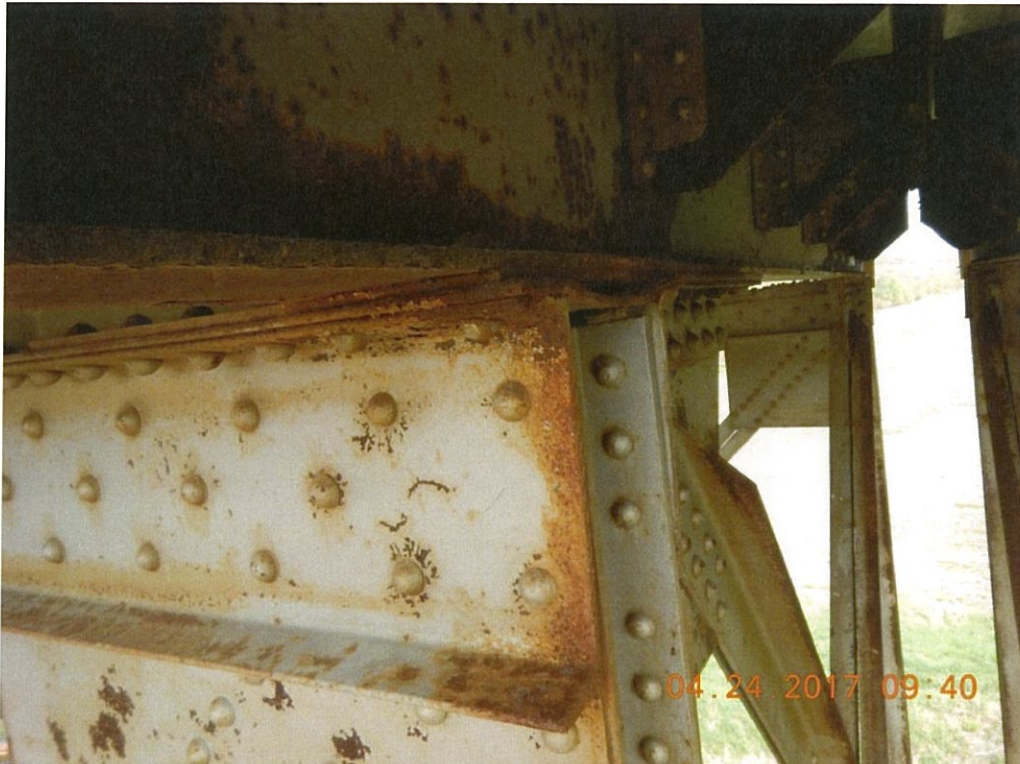
Photo 37: Minor packrust up to 1/4" is typical at the deck truss upper connections below the deck joints. Span 7 U0 Lt. end shown.
