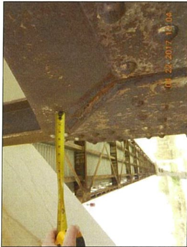
Span 4 L10 Lt top exterior packrust
