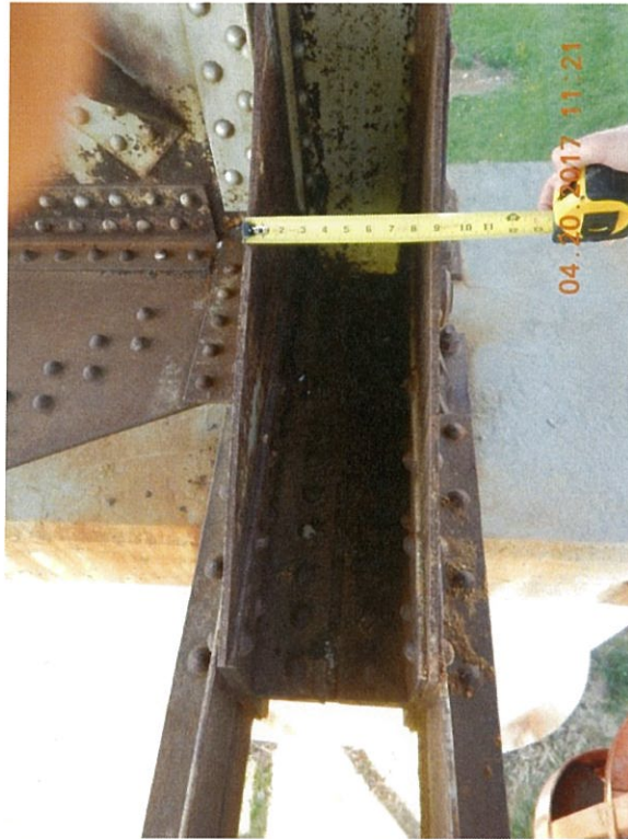
Photo 43: The lower chord gusset plates at the deck truss bearings are typically bowed inward at the top. Span 2 L0 Lt. shown.
