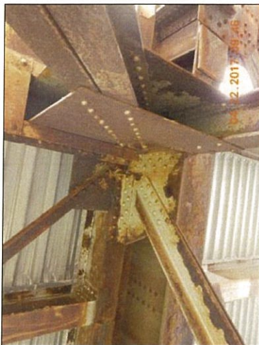
Span 4 U10 Rt interior deterioration
