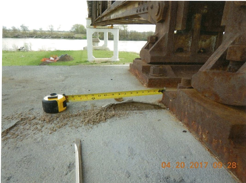
Photo 121: The top of the Pier 2 cap has sealant coat deterioration with sand and aggregate underneath it at one location on the north.
