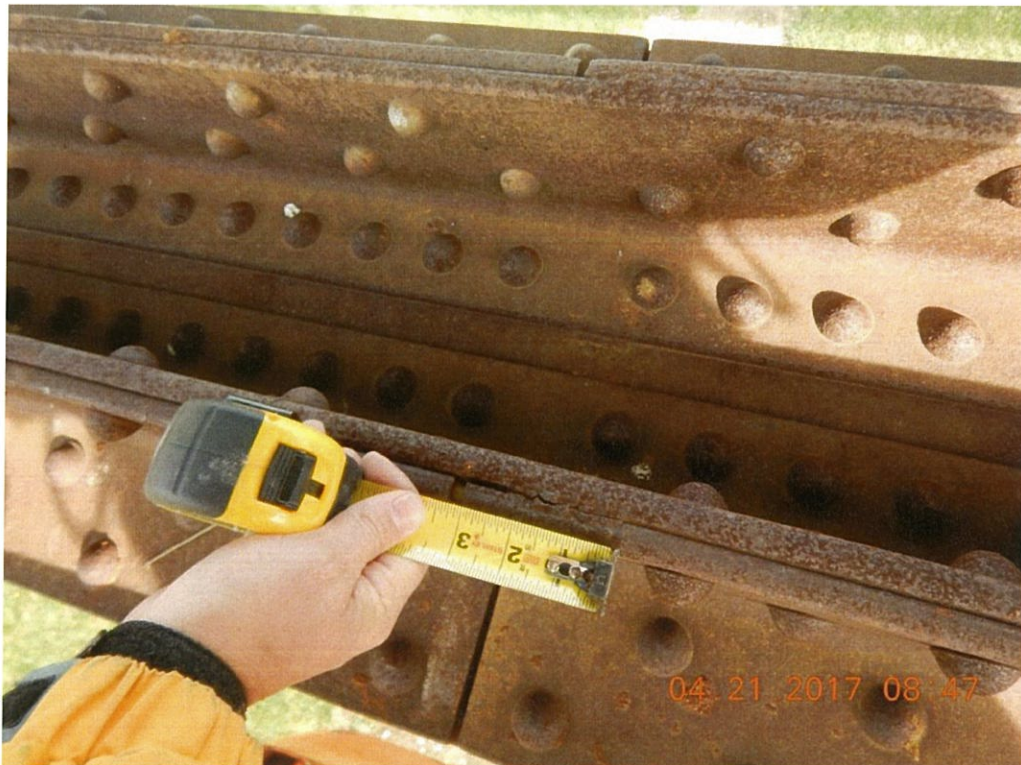
Photo 52: The riveted splice connections in the deck truss lower chords have tack welds placed during construction. Cracks found through welds at some locations. Span 2 L3L4 Rt. shown.
