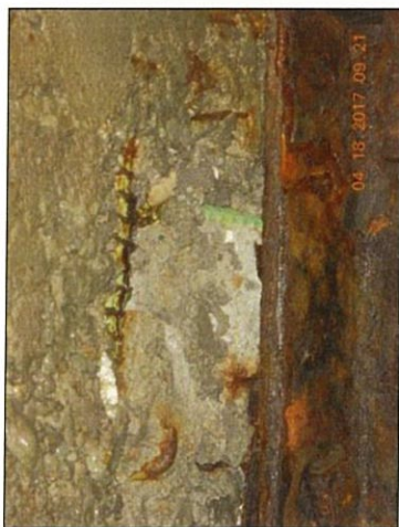
Span 11 Abutment 2 South deck corner poor consolidation with exposed rebar
