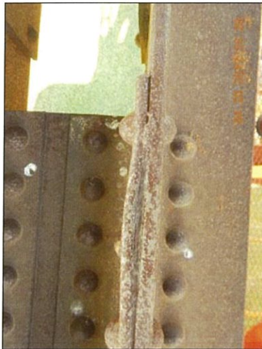
Span 3 L1L2 Rt splice tack weld crack
