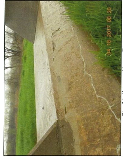
Pier 6 bottom cracking on East
