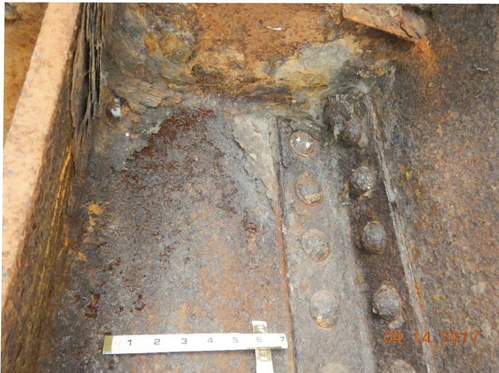
Photo 93: Thru truss floorbeam corrosion shown in Span 5 at Floorbeam 0 below the joint.
