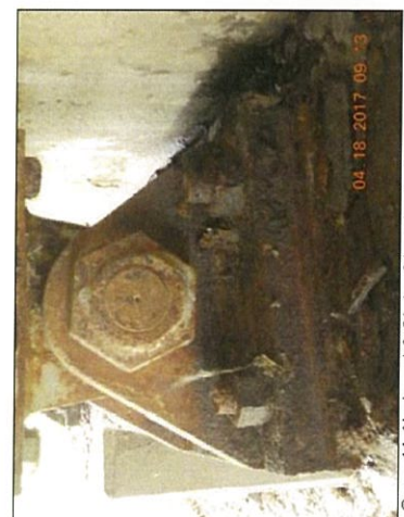
Span 11 Abutment 2 Girder 2 bearing looking North - nuts and bolts deterioration
