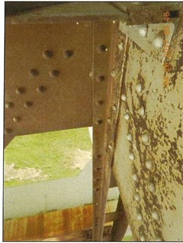
Span 2 L9 Lt interior packrust at top of lower chords
