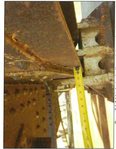
Span 3 L0 Lt interior bottom plate packrust
