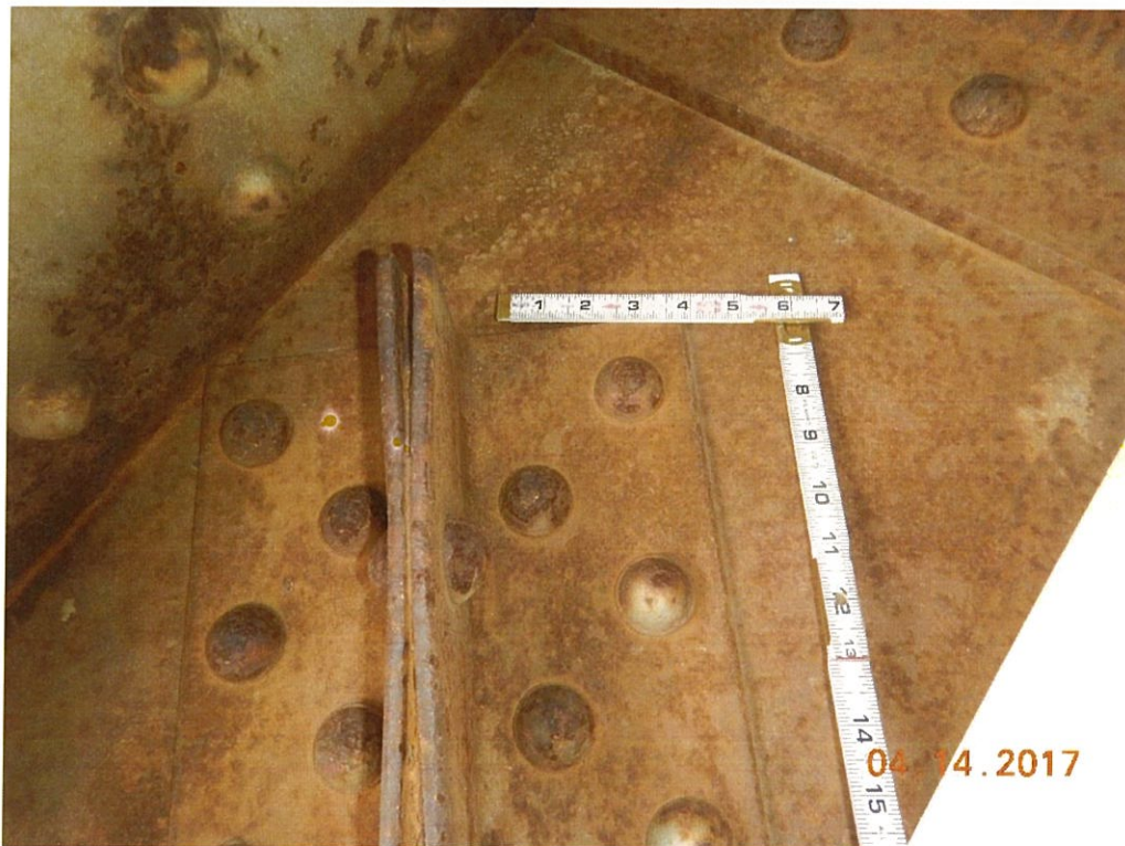
Photo 86: Areas of heavy corrosion and packrust are located at ends of the thru truss lower lateral bracing angles near the gusset plate connections.
