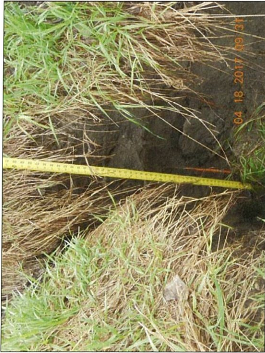
East approach erosion ditch on North measurement
