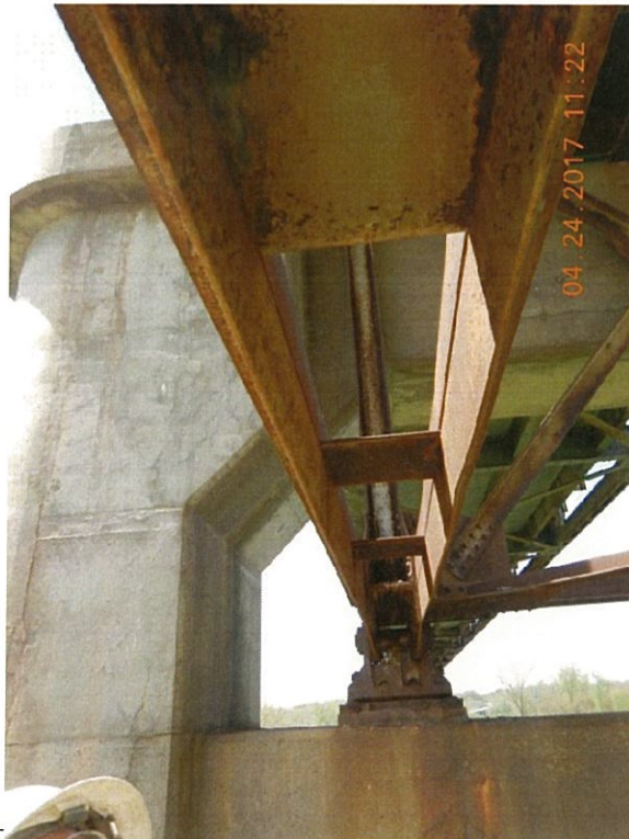
Photo 42: The vertical angles of the deck truss lower chords from L0 to L2 and L8 to L10 were typically bowed outward with the interior leg of Span 7 L0L1 Rt. distorting in a wave pattern.
