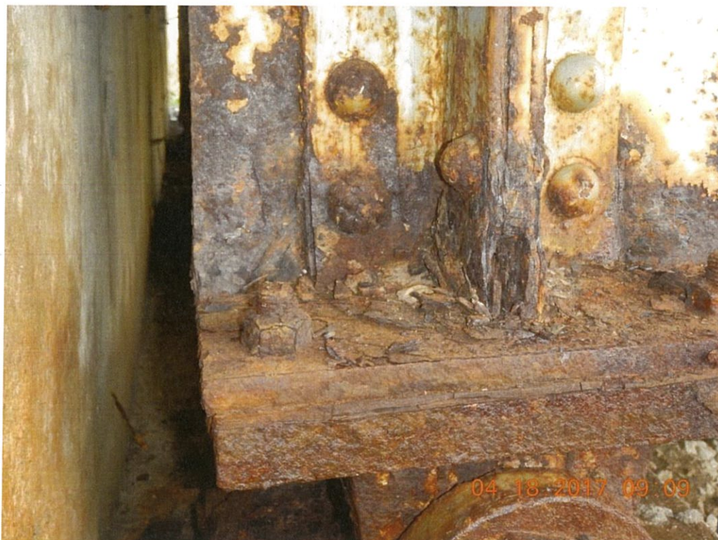
Photo 102: The leaking joints at above the ends of the girders have caused heavy rust with some section loss in the girder webs. Girder 1 exterior face at Abutment 2 shown.
