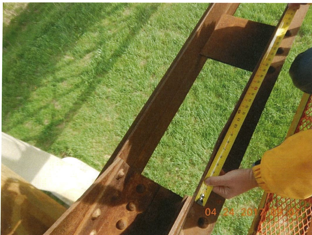
Photo 49: Small dents are present at some locations throughout the deck truss. These dents were most likely created during construction. Span 8 L0L1 Rt. exterior at L0 shown.
