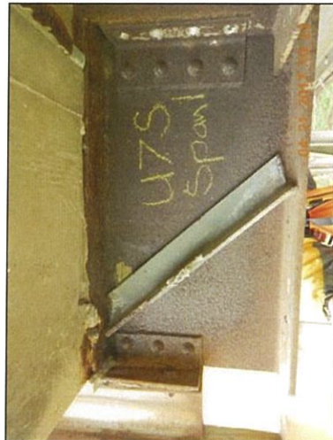
Span 1 Floorbeam 7 Rt stiffened and deterioration
