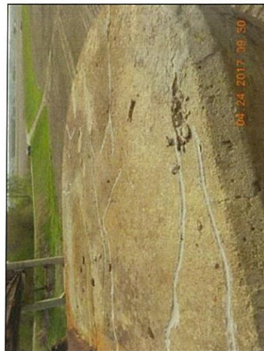
Pier 6 South end cap deterioration
