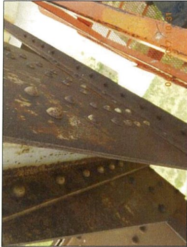
Span 4 L1 Lt exterior packrust
