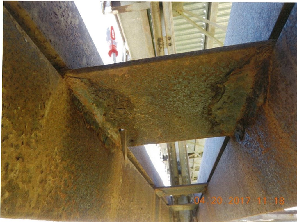
Photo 25: Similar loss in Span 2 L0L1 Lt. west batten plate as shown in Photos 22 and 23.
