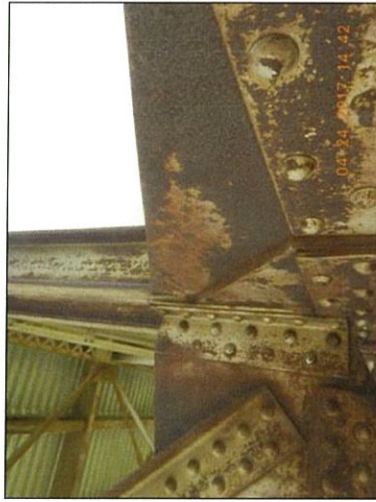
Span 8 L0 Lt top interior packrust
