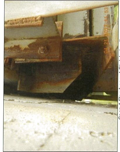
Span 1 Floorbeam 1 Rt deterioration
