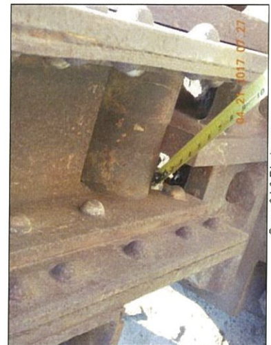
Span 3 L0 Rt pin wear
