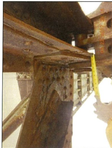
Span 4 L10 Rt bottom interior packrust
