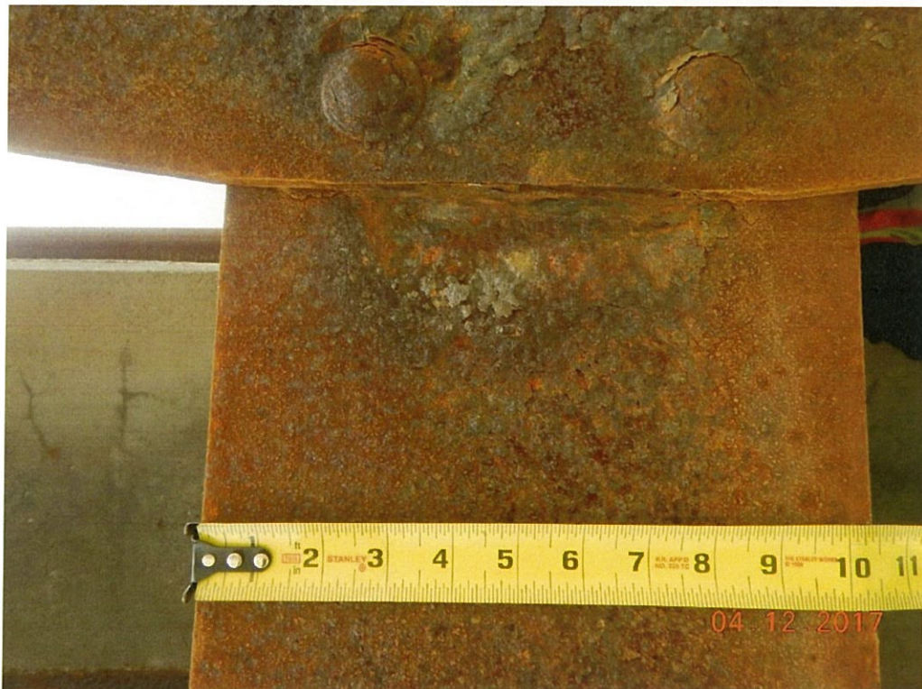
Photo 90: Many of the remaining, un-strengthened, floorbeams have significant section loss of the flanges, webs, and rivets. Section loss at an isolated area of the underside of the bottom flanges at the beam ends to gusset plate connection.
