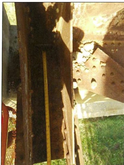
Span 8 L10 Lt top deterioration
