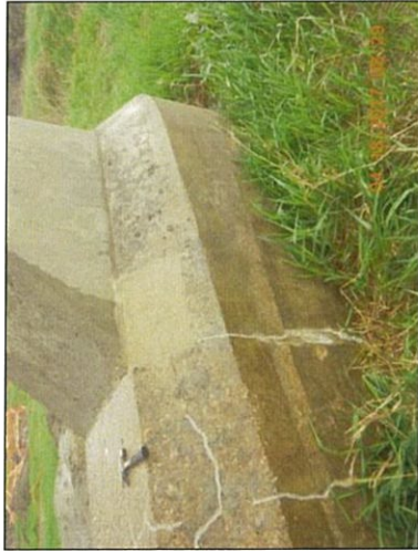
Pier 7 bottom efflorescence at Northeast
