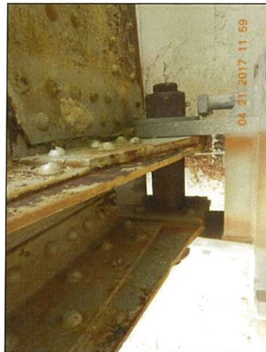
Span 1 L0 Rt bottom interior packrust
