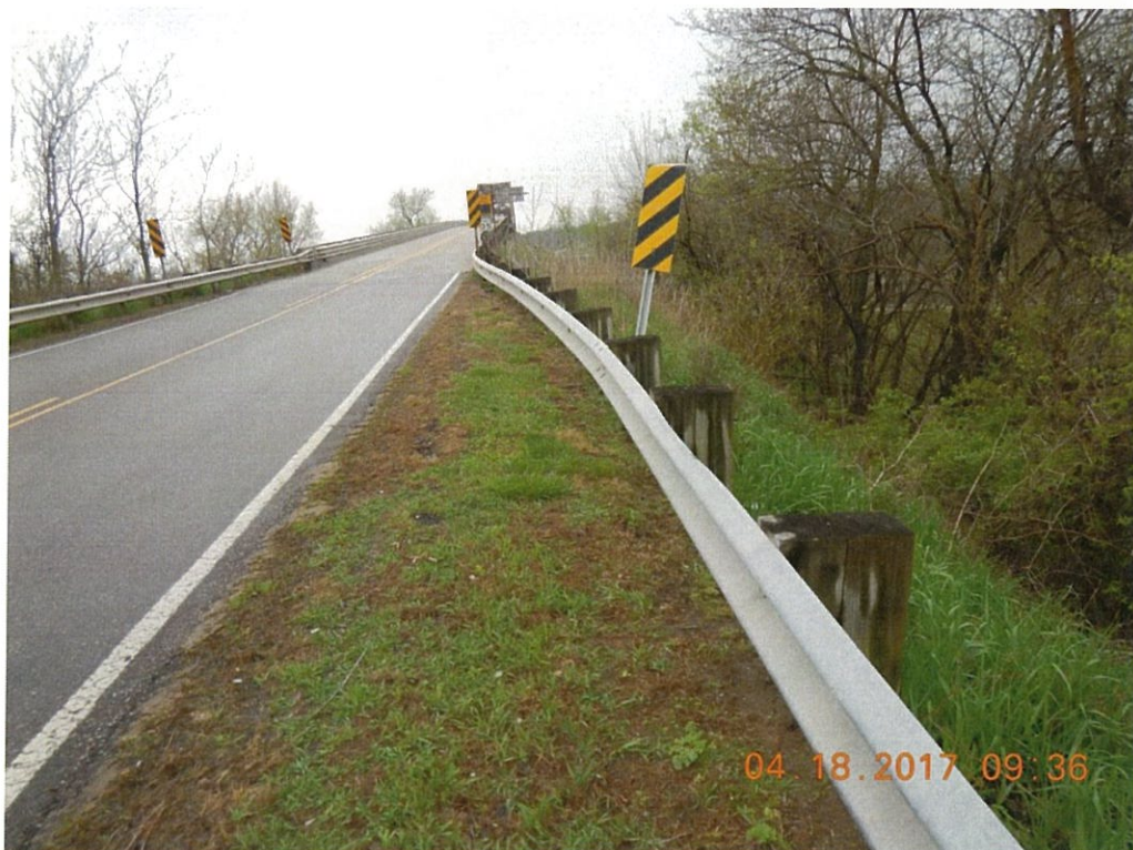
Photo 18: The northeast approach rail center has minor impact damage. One of the northeast delineators has minor misalignment and deformation.
