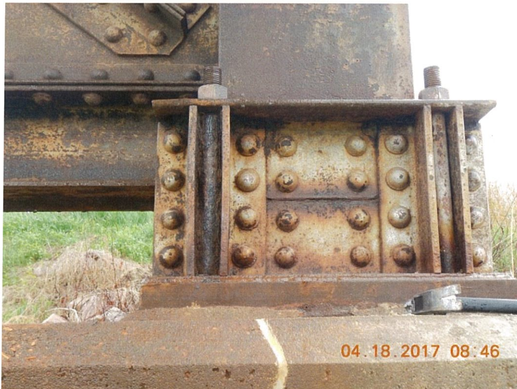
Photo 132: Heavy packrust has developed between the Pier 9 steel column anchor bolts and their stiffeners; there is section loss on some bolts. West bolts at the south column shown.
