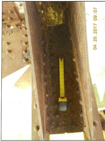
Span 3 L0 Lt end plate deterioration with rivets severely deteriorated on exterior side
