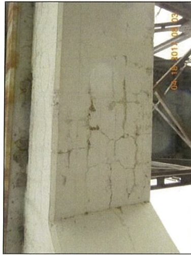
Pier 1 bottom of strut cracking closeup
