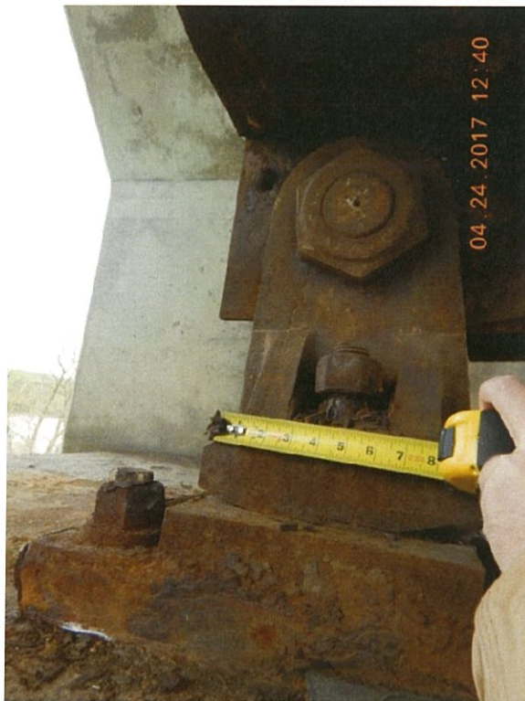
Photo 109: The deck truss expansion bearing anchor bolts have delamination in the threads between the nut and the bearing; the debris from this is filling up the slots. Span 7 L0 Lt. interior shown.
