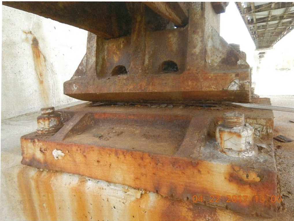
Photo 108: Packrust is developing below the deck truss expansion bearing rockers creating minor debris. Span 4 L10 Lt. shown.
