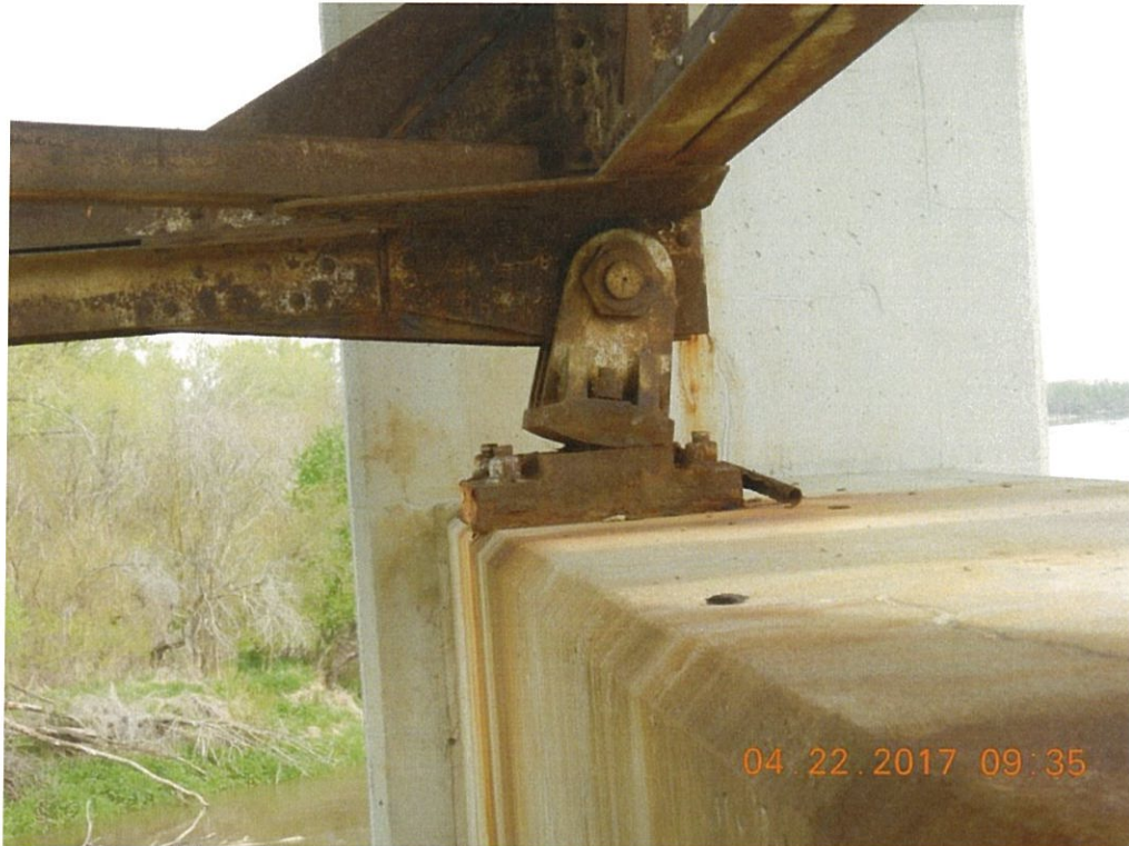
Photo 107: All of the deck truss expansion bearings appear to be over rotated. Span 4 L10 Lt. shown.
