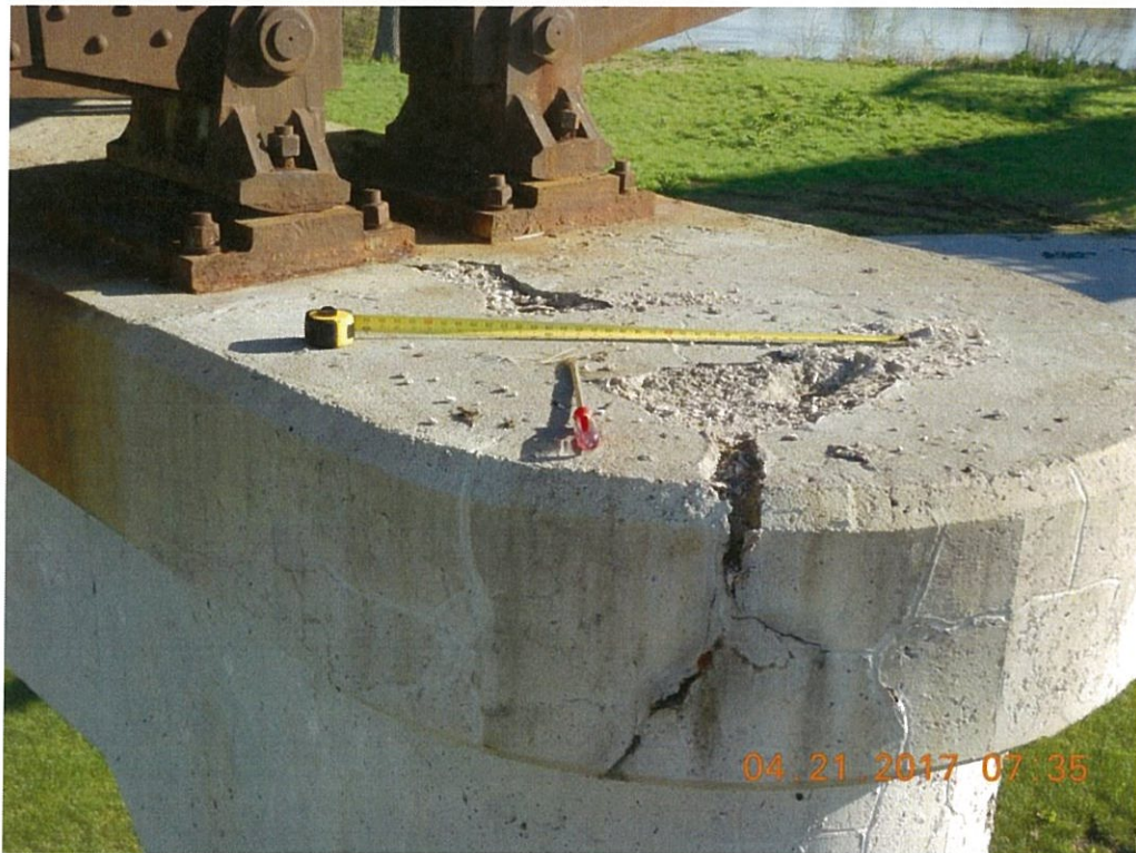
Photo 120: The top of the Pier 2 cap has sealant coat deterioration with sand and aggregate underneath it at two locations on the south.
