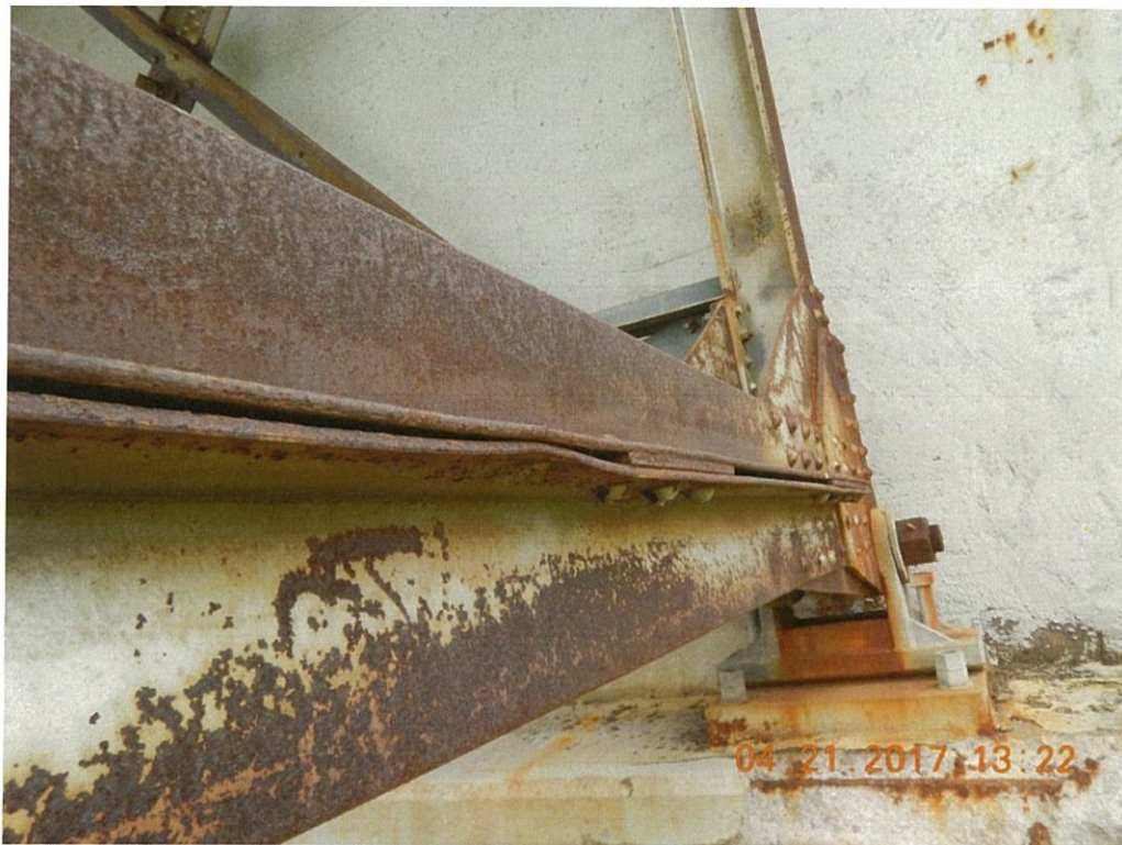
Photo 46: Small dents are present at some locations throughout the deck truss. These dents were most likely created during construction. Span 1 L0L1 Lt. exterior near L0 shown.
