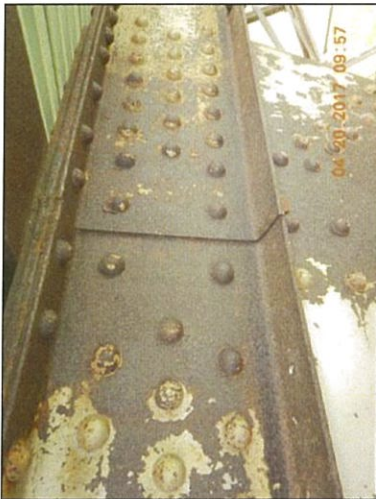
Span 2 U8 Lt exterior upper channels not lined up
