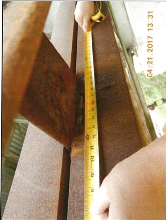
Span 1 L1L2 Lt bottom interior angle hole below middle batten plate
