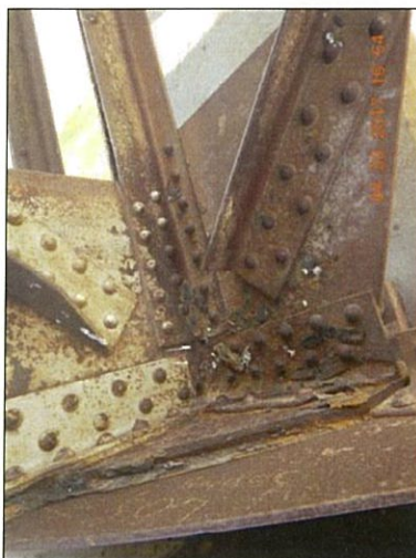
Span 3 L0 Rt horizontal gusset plate deterioration
