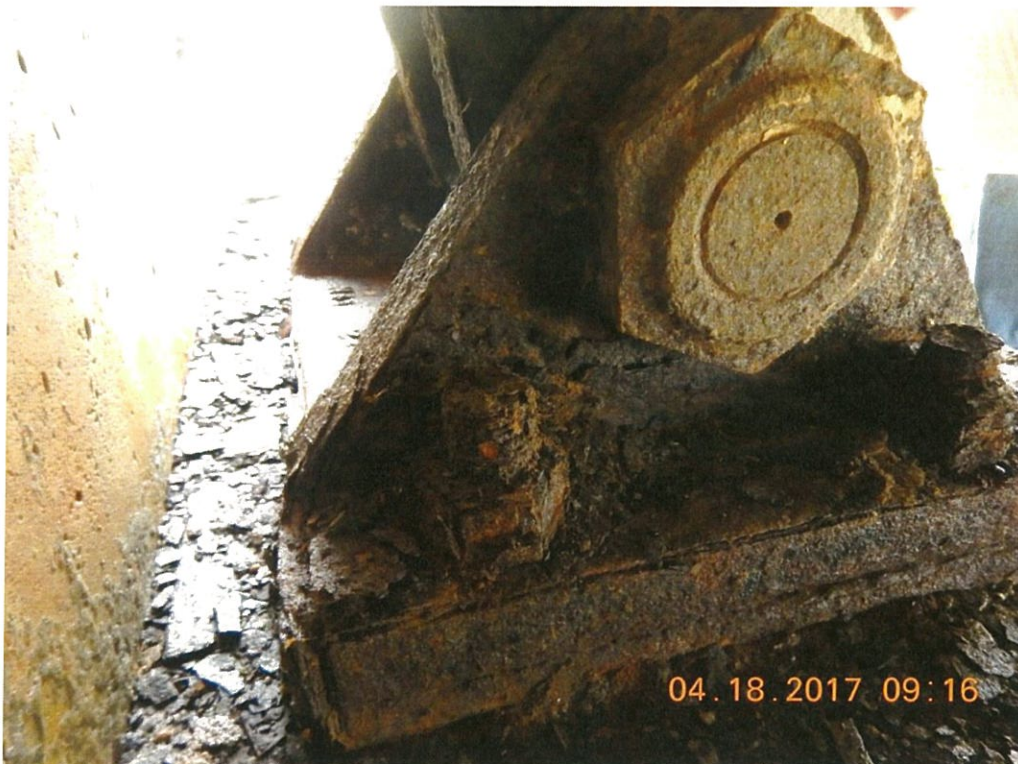
Photo 114: The north bolts at Abutment 2 for Span 11 Girder 4 are starting to deteriorated in a similar manner as shown in Photo 113. This is typical at all four bolts of Girders 1 and 2.
