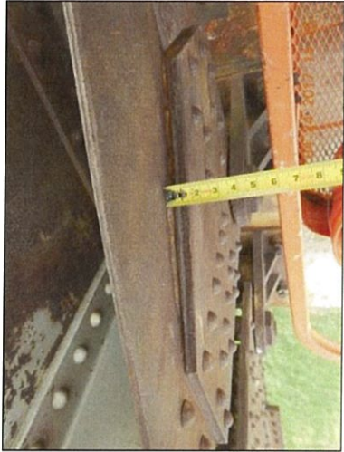
Span 7 L10 Lt top exterior packrust
