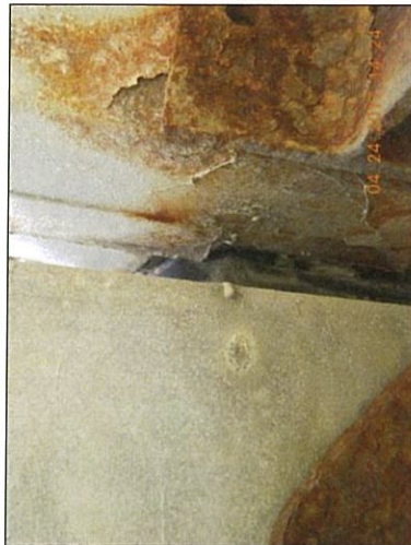
Pier 7 deck joint holes on north end
