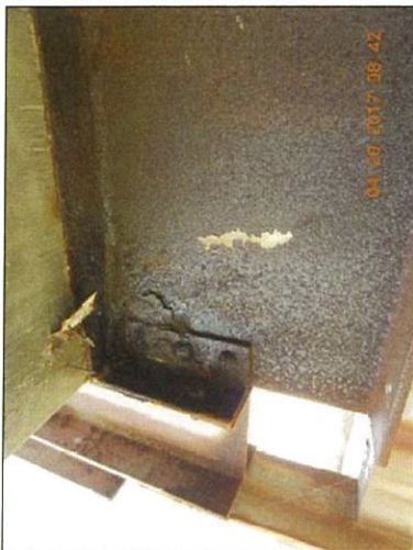
Span 3 Floorbeam 2 Lt web deterioration
