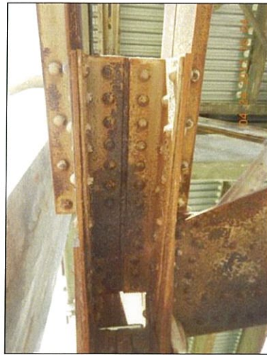
Span 8 L10 Lt bottom deterioration
