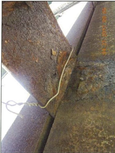
Span 2 L1L2 Rt middle batten plate deterioration
