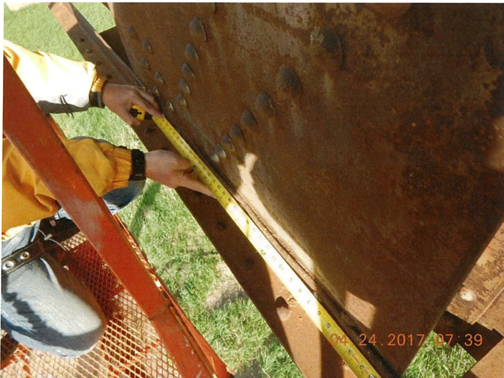
Photo 29: Minor packrust up to 1/4" is typical at the members coming into the deck truss lower connection gusset plates, excluding end connections. Span 8 L9 Rt. exterior shown.
