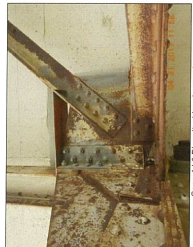
Span 1 L0 Rt vertical bracing angles
