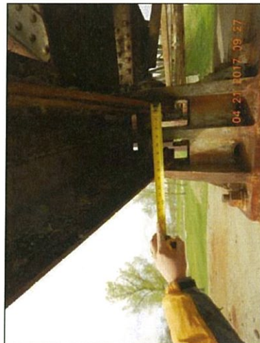
Span 2 L0 Rt gusset plates bent inward
