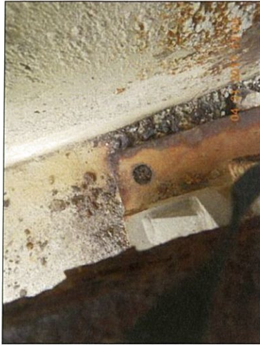
Span 1 L0 Lt interior-back bolt not installed - typ Rt
