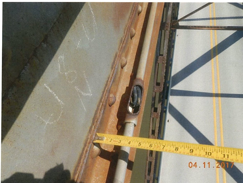
Photo 137: There is a missing conduit junction box cover on top of the Pier 4 cap at the north end and in Span 5 along the inside of U8U9 Lt. – shown.
