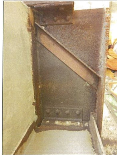
Span 8 Floorbeam 6 Rt stiffened and hole
