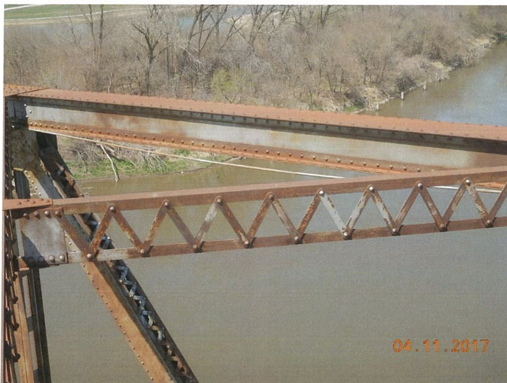
Photo 138: The conduit in Span 5 is unsupported along the inside U7U8 Lt.
