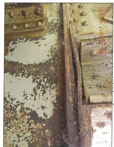
Span 3 U0 Lt end packrust
