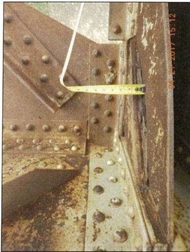
Span 1 L10 Lt top interior packrust
