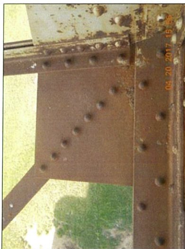
Span 3 L3 Rt horizontal gusset plate deterioration
