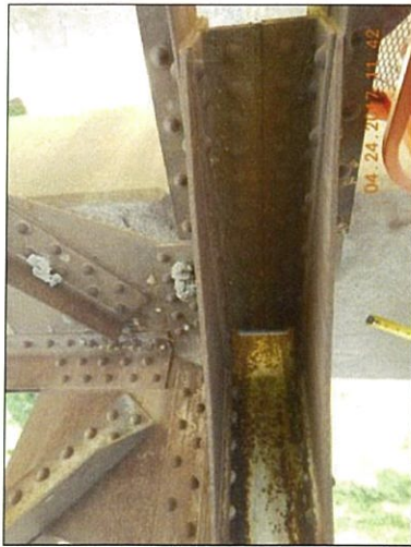
Span 7 L0 Rt top deterioration
