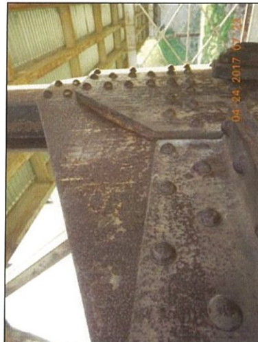
Span 8 L10 Rt top exterior packrust
