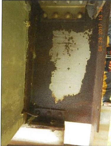
Span 7 Floorbeam 4 Lt hole
