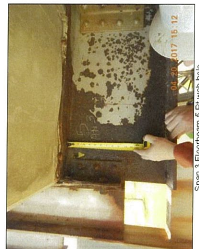
Span 3 Floorbeam 4 Stringer 4 deterioration
