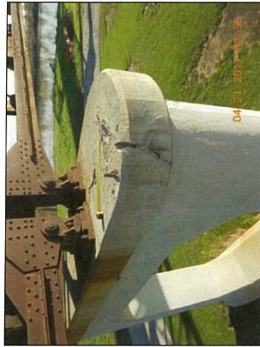
Pier 2 South cap deterioration
