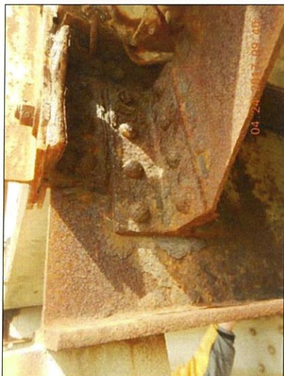
Span 7 Floorbeam 10 Rt deterioration below joint
