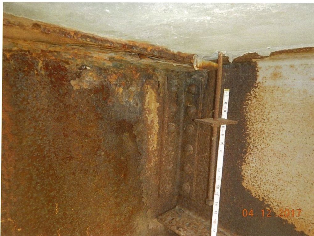
Photo 96: Two locations, Floorbeams L4' and L3', have 1/4" diameter holes in the web near the top flange. Floorbeam L4' shown.
