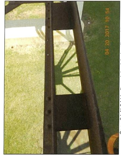
Span 2 L1L2 Lt batten plate deterioration at top
