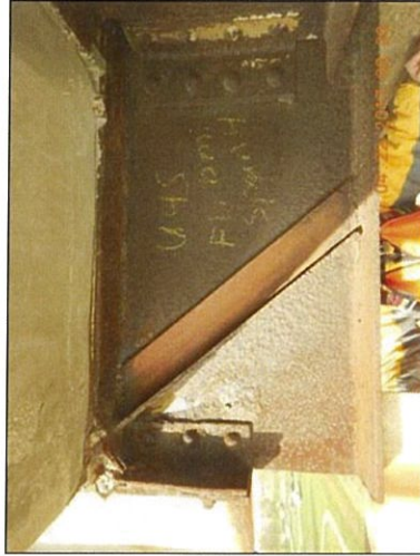
Span 4 Floorbeam 4 Rt stiffened and hole
