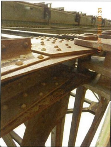
Span 7 L10 Rt bottom exterior packrust
