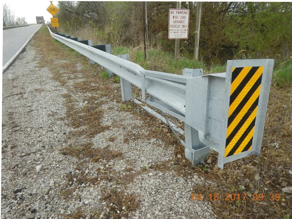
Photo 19: The northeast approach end terminal has minor impact damage.
