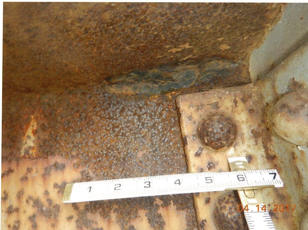
Photo 94: Thru truss floorbeam corrosion shown at Span 5 Floorbeam 2 Lt., web to bottom flange.
