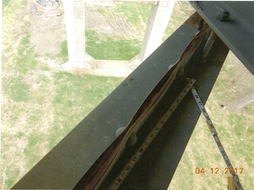
Photo 85: There is heavy packrust buildup between the angles of the thru truss lower lateral bracing.
