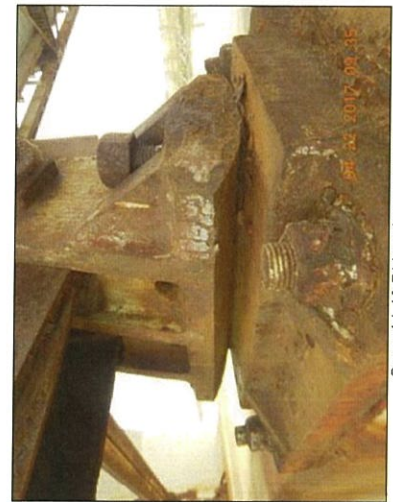
Span 4 L10 Rt bearing packrust
