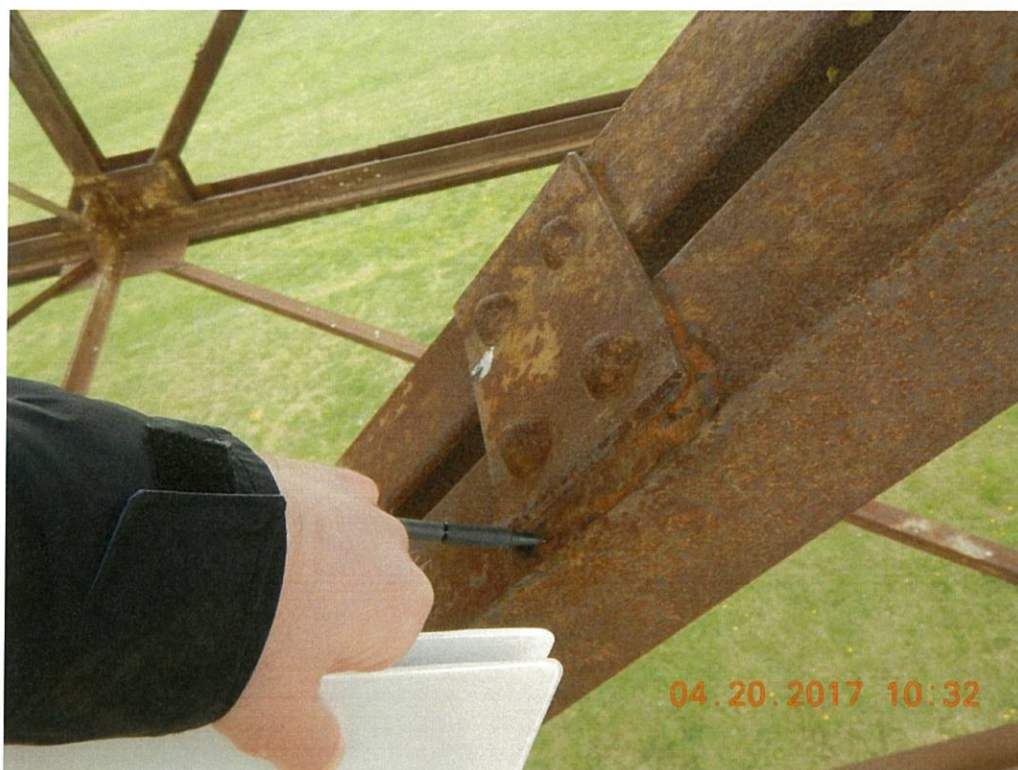
Photo 34: Minor packrust up to 1/4" is typical at the batten plates of the deck truss diagonals consisting of two angles. Span 2 U3L4 Lt. shown.
