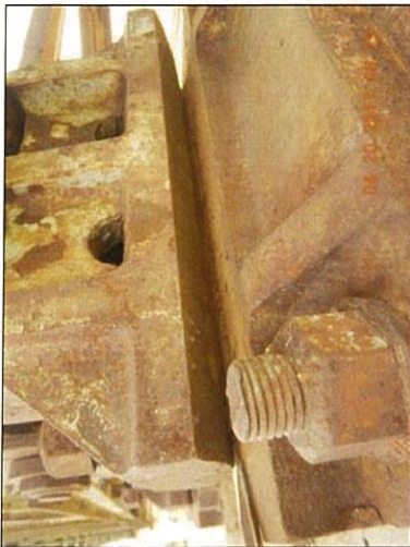
Span 2 L10 Lt minor packrust under bearing
