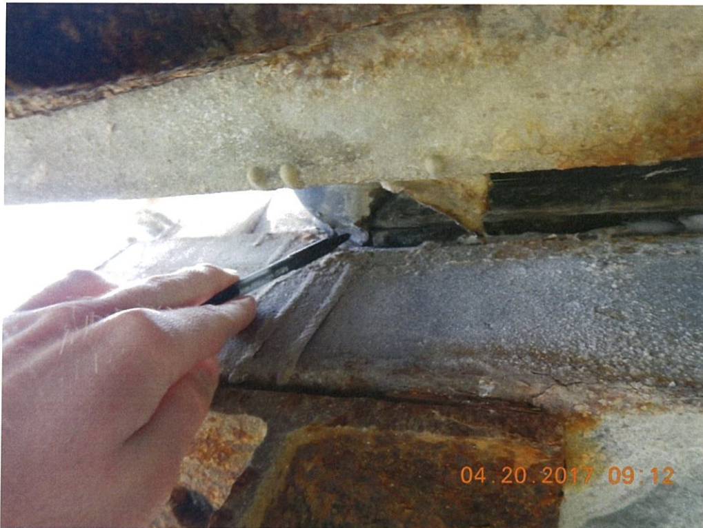
Photo 15: There are typically two small holes in each end of the joint, at all strip seal joints. The north end of the joint above Pier 2 is shown and water is visibly coming out of the hole.
