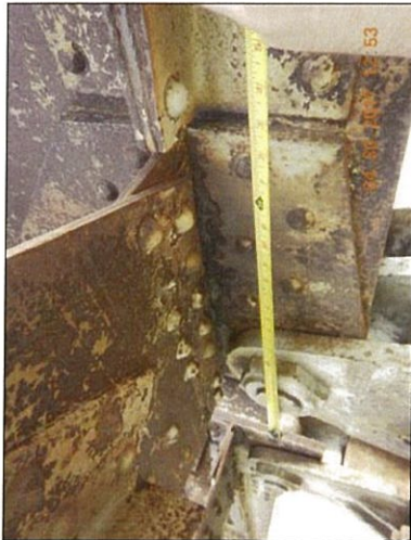
Span 3 L10 Rt bottom horizontal gusset plate packrust
