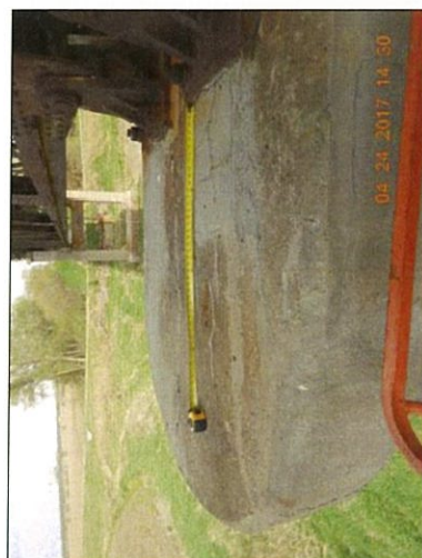
Pier 7 top north deterioration
