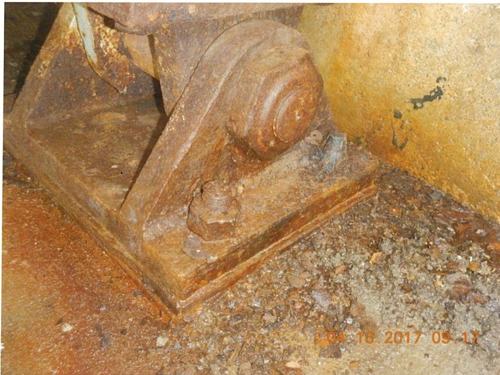
Photo 113: The southeast anchor bolt at Abutment 2 for Span 11 Girder 4 is deteriorated to the point no threads are distinguishable and the nut is almost completely gone.
