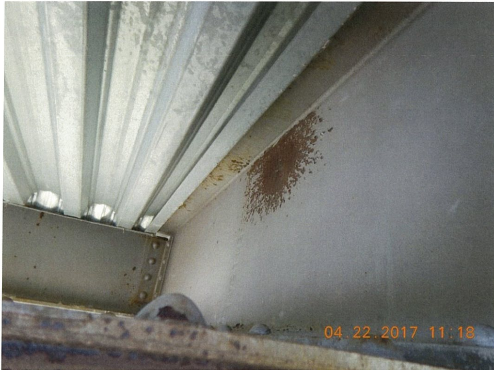
Photo 61: There are larger dimple dents in the deck truss floorbeam webs near the exterior stringers in a few locations. Span 4 Floorbeam 5 Lt. shown.
