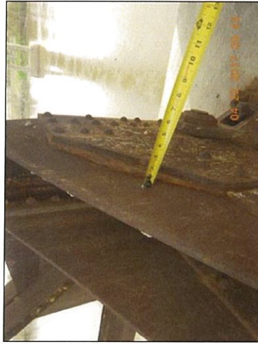
Span 4 L10 Rt top exterior packrust
