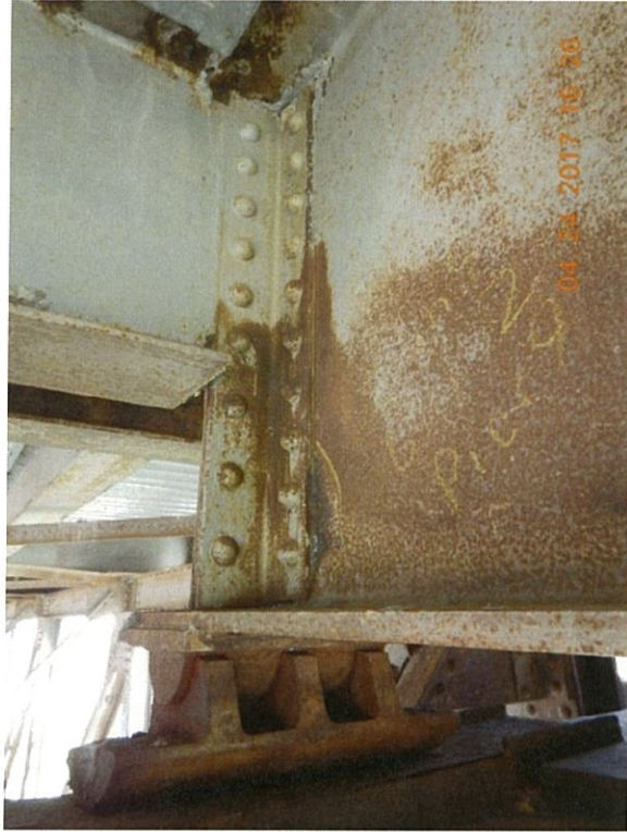
Photo 99: The leaking joints at above the ends of the girders have caused heavy rust with some section loss in the girder webs. Girder 2 interior face at Pier 8 shown.
