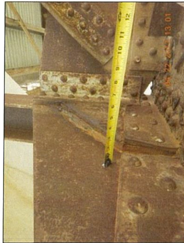
Span 4 L10 Lt top interior packrust (2)
