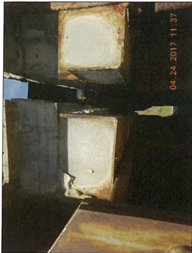
Pier 6 deck joint South end possible leak
