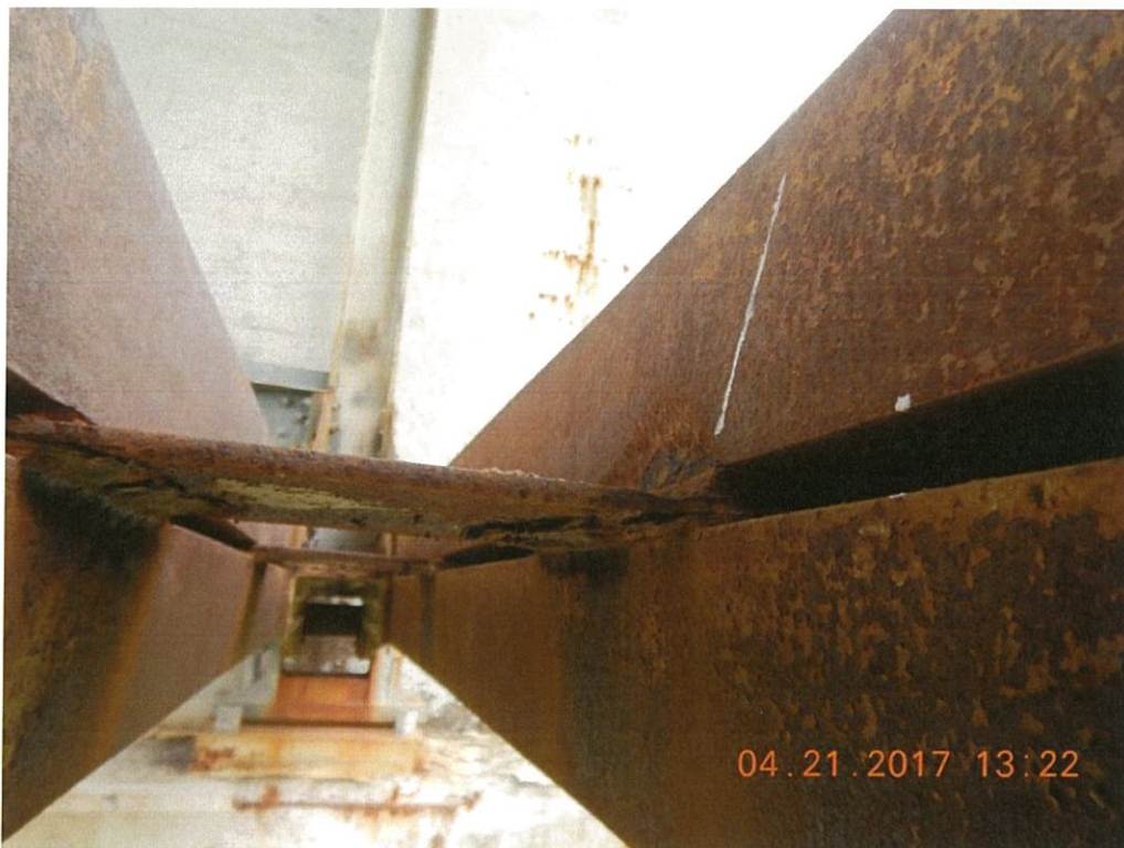
Photo 22: The section loss at the batten plates of the deck truss lower chords is typically on the inside of the lower chord angle above and below the batten plate. Span 1 L0L1 Lt. shown.
