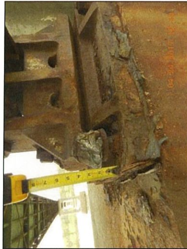
Span 7 L0 Lt front interior nut not down
