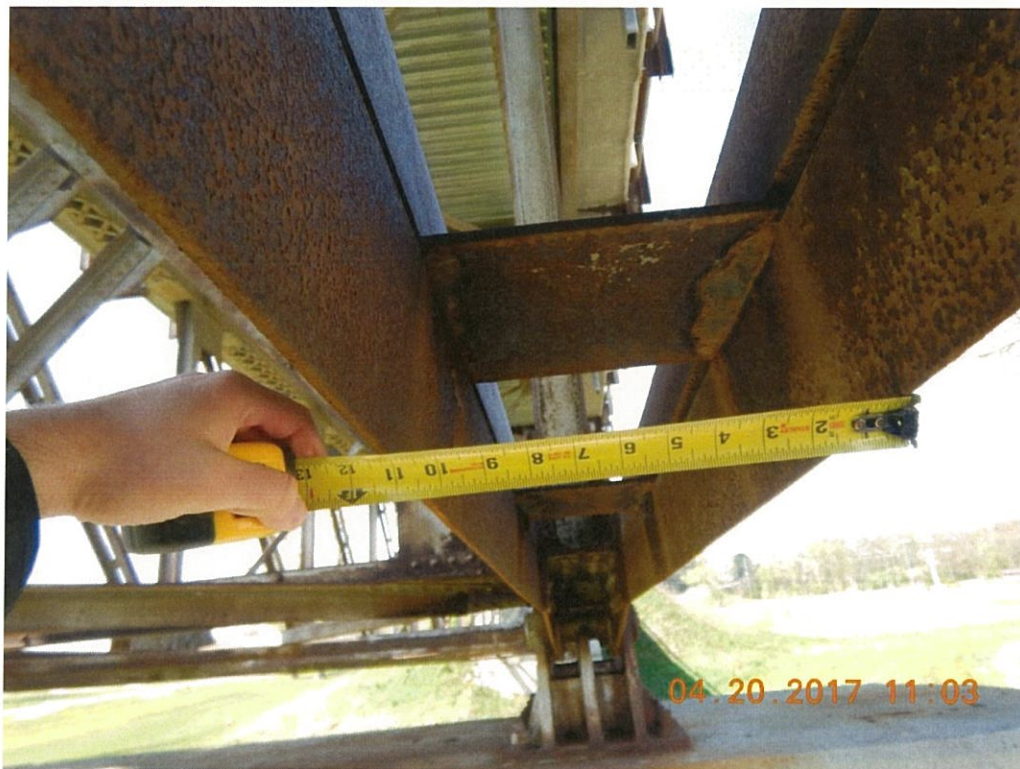
Photo 40: The vertical angles of the deck truss lower chords from L0 to L2 and L8 to L10 were typically bowed outward. Span 2 L0L1 Lt. shown.
