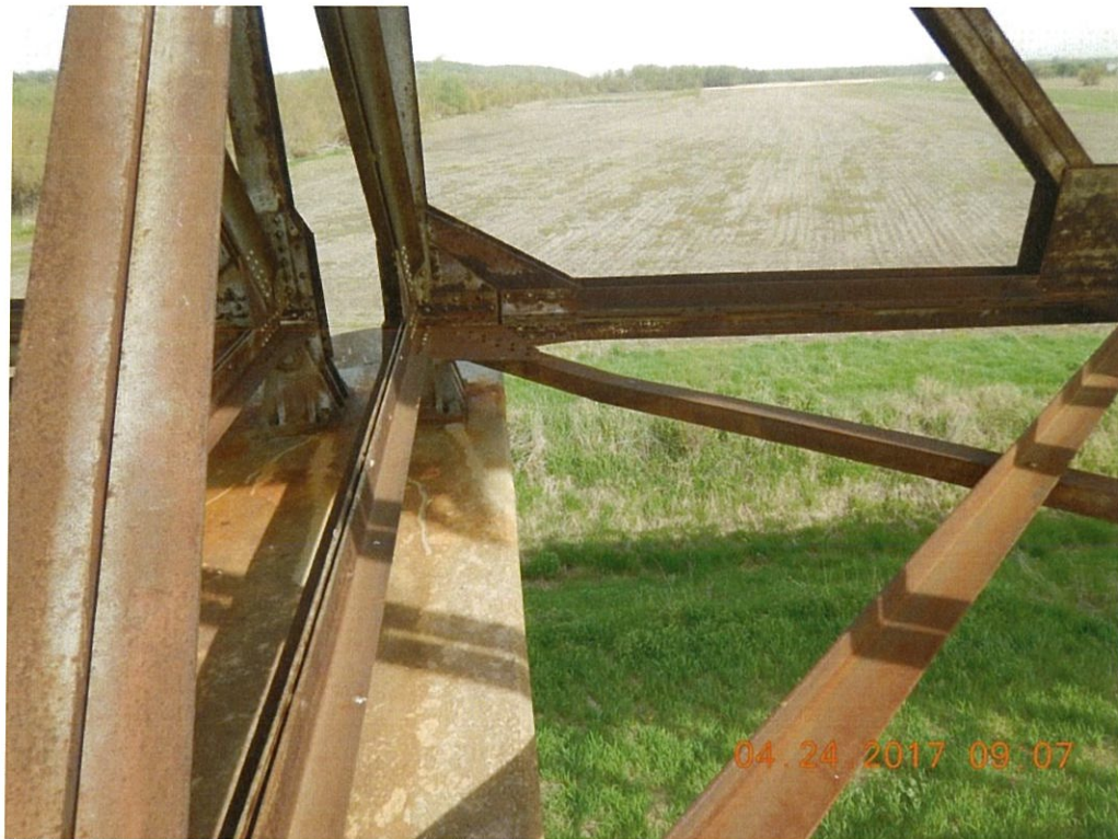
Photo 69: Deck truss lower lateral bracing is bent at Span 8 Bay 1.
