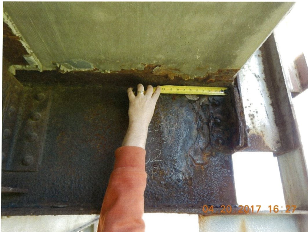
Photo 59: Several of the deck truss floorbeam ends have full penetration section loss varying in size. Span 3 Floorbeam 2 Rt. shown.
