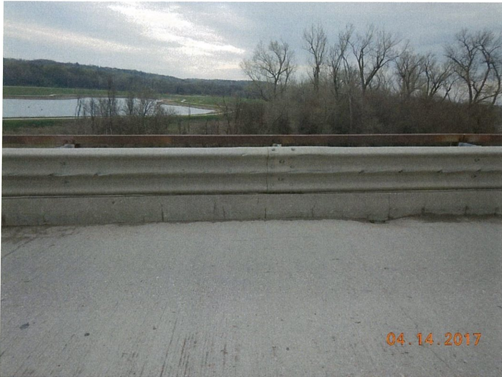
Photo 11: The curbs have hairline vertical cracking with spacing of 2' to 4' throughout their entire length. Minor impact damage is present along both rails with several jagged tears.
