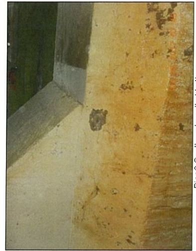
Pier 2 Southeast spall at bottom
