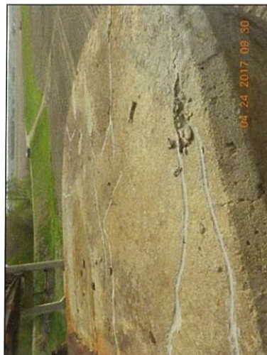
Pier 7 South end cap deterioration
