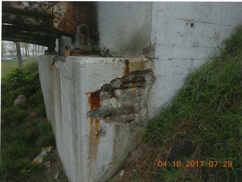
Photo 117: The north vertical face of the Abutment 1 cap is spalled 2" deep for approximately 2' by 2'.
