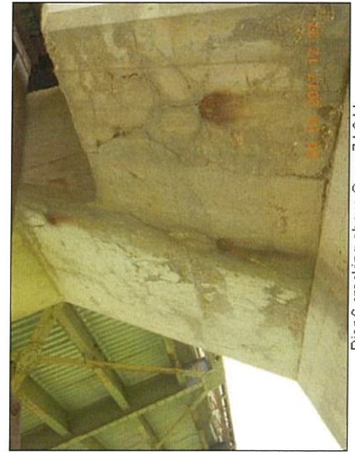
Pier 6 cracking above Span 7 L0 Lt
