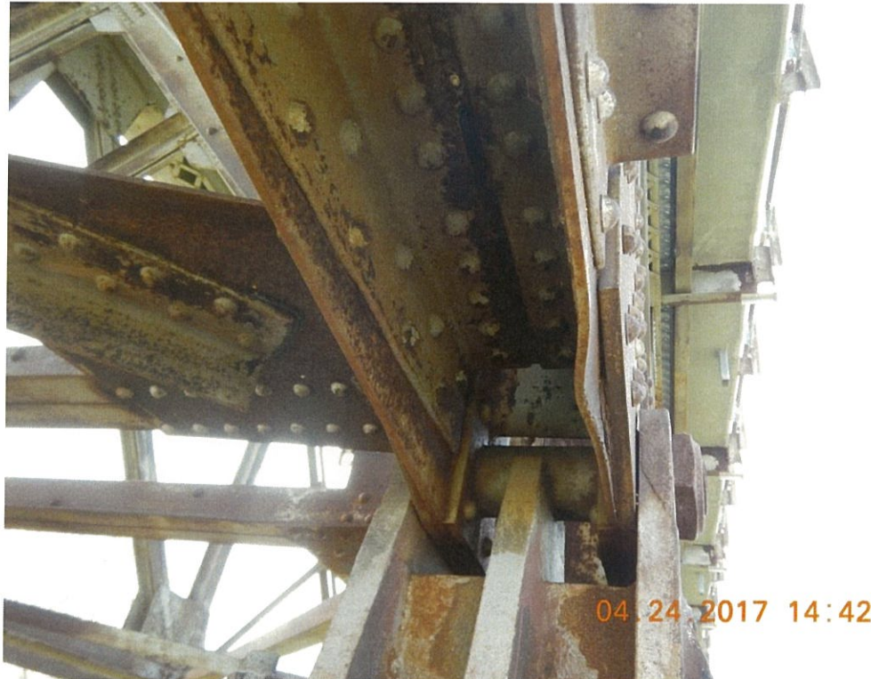
Photo 45: The lower chord gusset plates at the deck truss bearings are typically bowed inward at the bottom. Span 8 L0 Lt. shown, also has a dent on the exterior.
