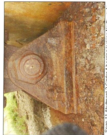
Span 11 Abutment 2 Girder 4 bearing looking North - nuts and bolt deterioration
