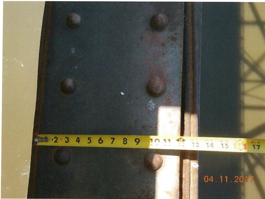
Photo 75: Packrust is present at most lower chords of the thru truss spans.
