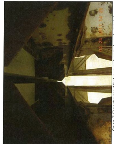
Span 7 Floorbeam 10 deterioration below deck joint
