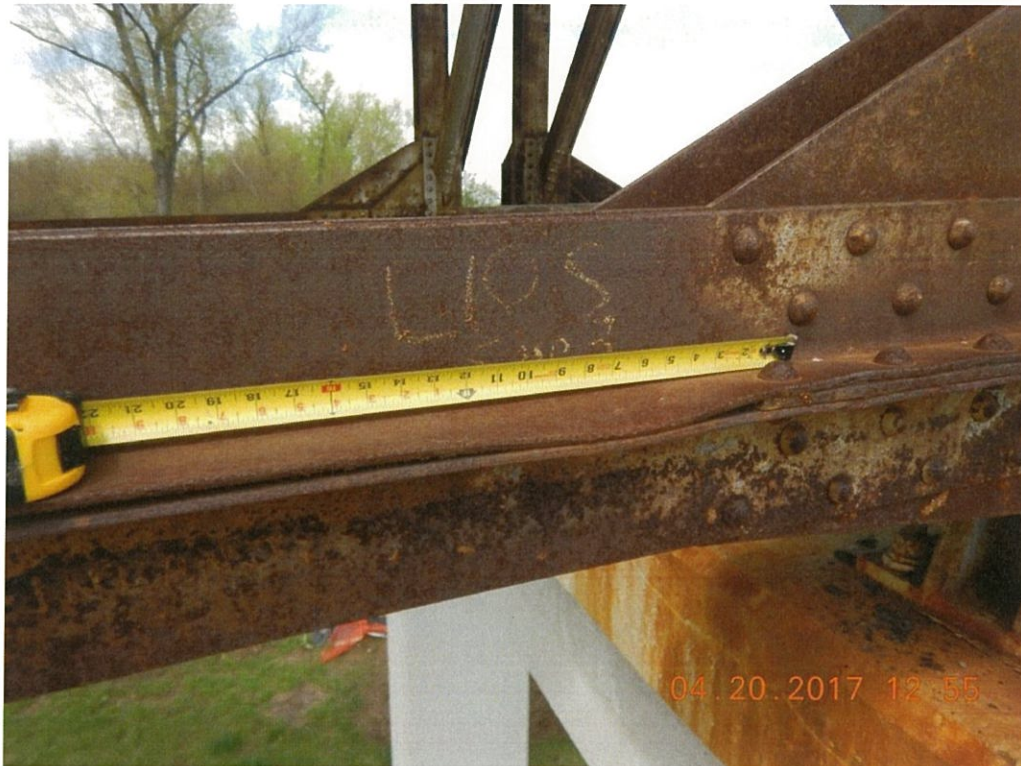
Photo 48: Small dents are present at some locations throughout the deck truss. These dents were most likely created during construction. Span 3 L9L10 Rt. exterior at L10 shown.
