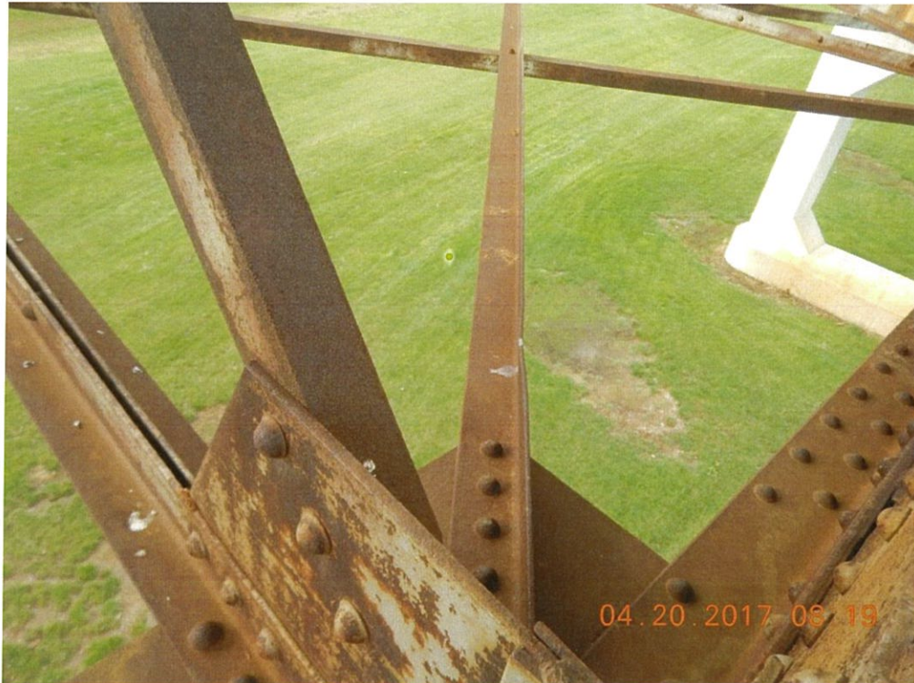
Photo 66: Deck truss lower lateral bracing is bent at Span 3 Bay 4.
