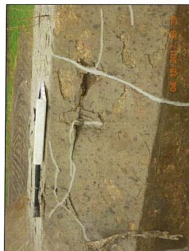
Pier 8 bottom cracking and poor consolidation
