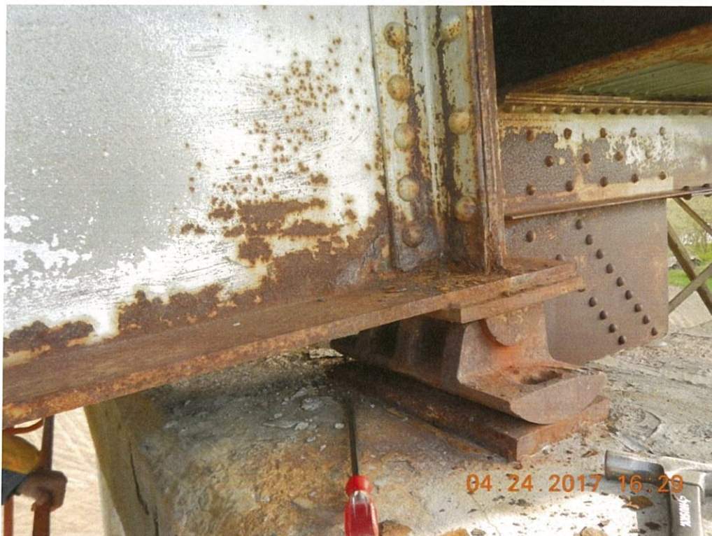
Photo 98: The leaking joints at above the ends of the girders have caused heavy rust with some section loss in the girder webs. Girder 1 exterior face at Pier 8 shown – exterior anchor bolt is sheared off).
