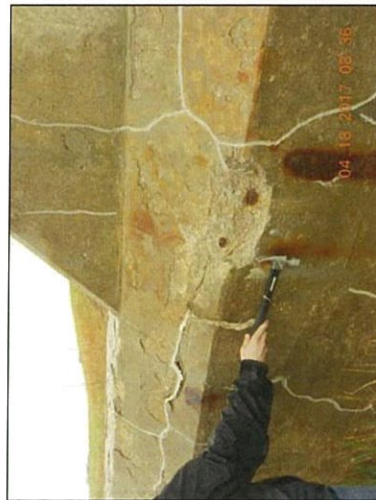
Pier 8 spill at Southwest bottom
