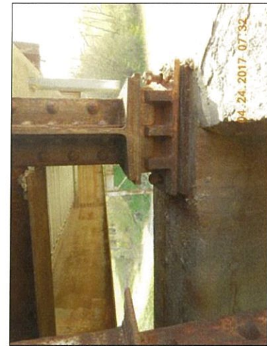
Span 9 Girder 4 bearing at Pier 8 deterioration
