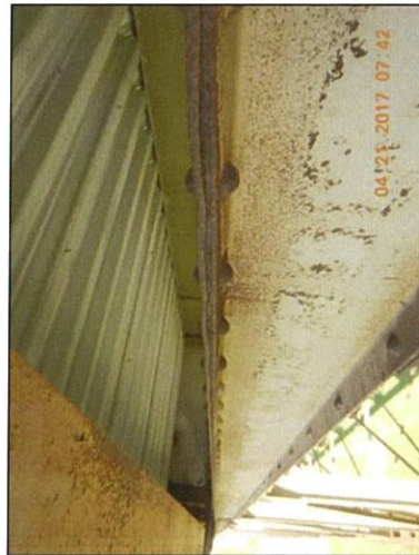
Span 2 U10 Rt typ packrust at upper chord cover plates
