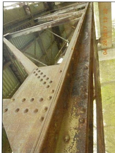
Span 7 L3 Lt exterior deterioration
