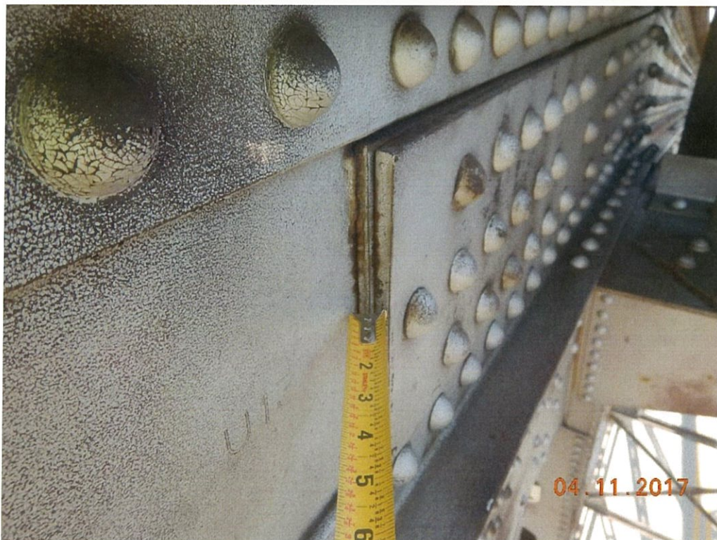
Photo 72: One thru truss upper chord tack weld was found with a crack through the weld with no sign of propagation into the base metal. The cracked tack weld is located at the north splice plate of Span 6 U13' Rt.
