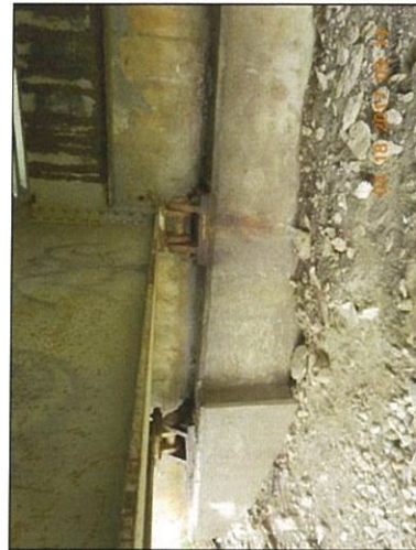
Bearings Abutment 2 Girders 1 and 2
