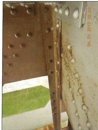
Span 1 L9 Lt interior packrust
