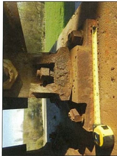
Span 3 L0 Lt interior anchor bolt bent
