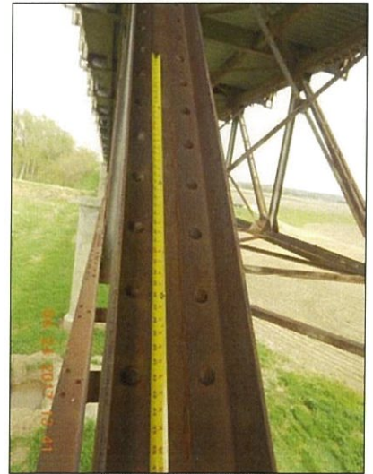
Span 7 U6L5 Lt packrust
