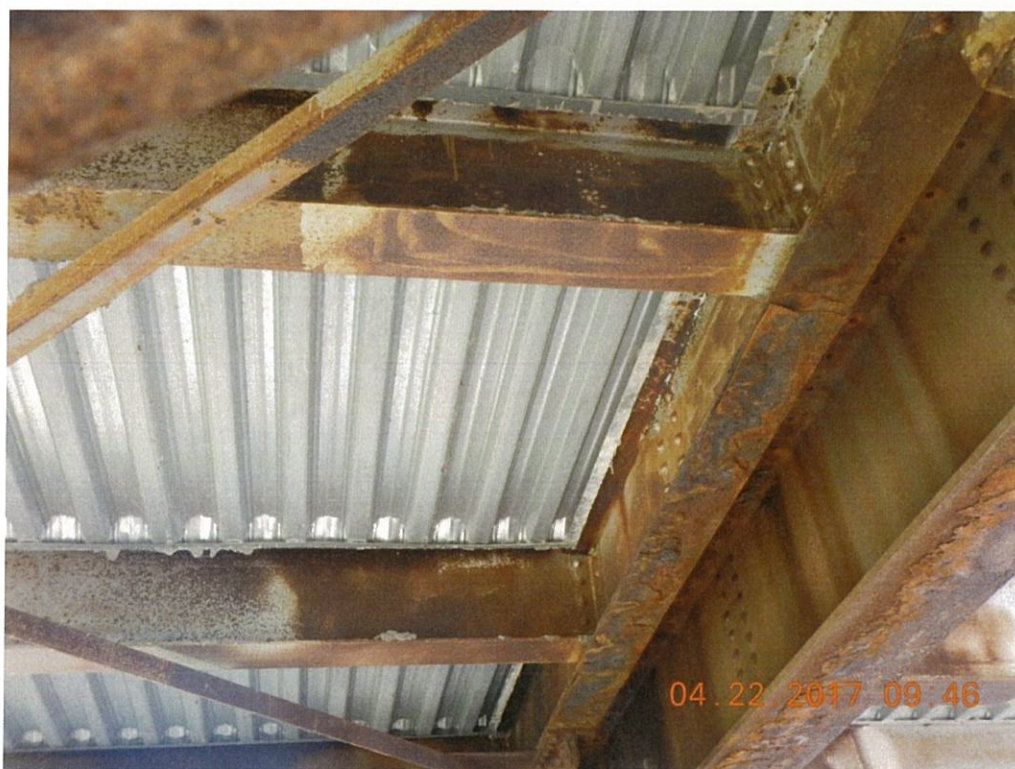
Photo 54: There are areas of delamination in the deck truss floorbeam faces below the deck joints. Span 4 Floorbeam 10 shown.
