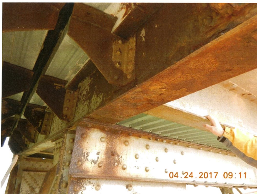
Photo 56: There are areas of delamination in the deck truss floorbeam faces below the deck joints. Span 8 Floorbeam 0 Rt. end shown.
