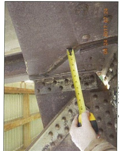
Span 8 L10 Rt top interior packrust
