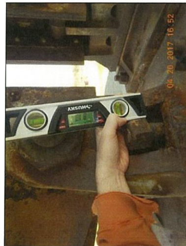
Span 3 L0 Rt interior anchor bolt bent
