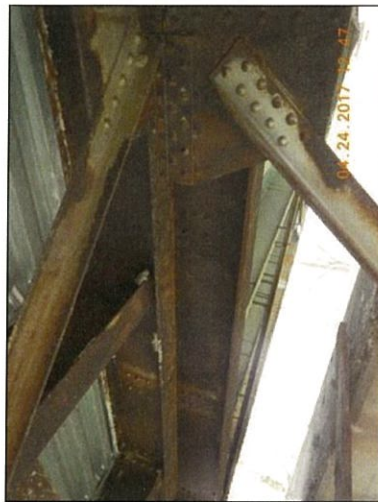
Span 7 Floorbeam 0 interior deterioration (2)
