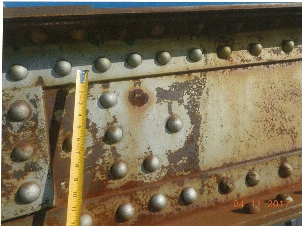
Photo 73: One rivet head is missing on the exterior face at Span 5 U1 Rt.
