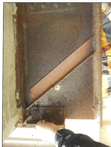
Span 3 Floorbeam 8 Rt stiffened and deterioration
