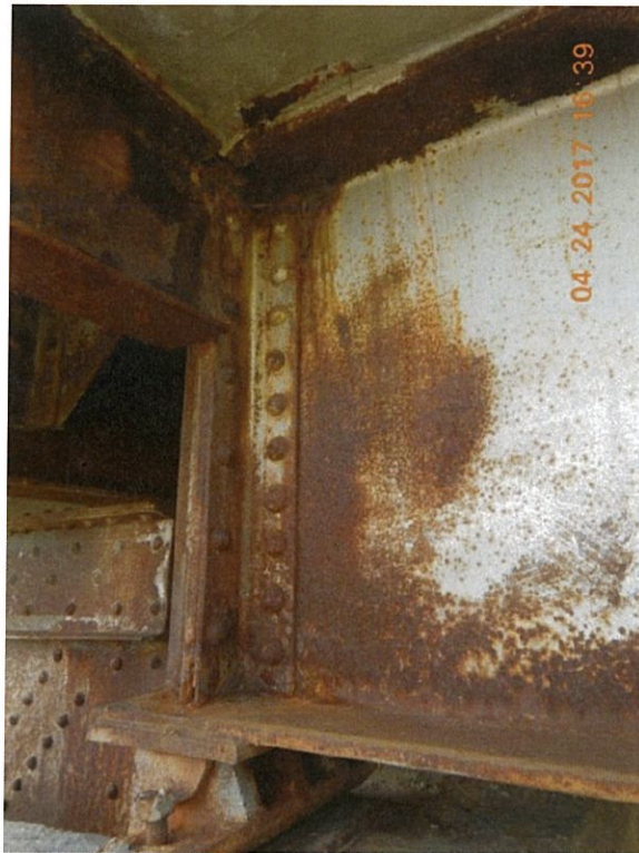
Photo 101: The leaking joints at above the ends of the girders have caused heavy rust with some section loss in the girder webs. Girder 4 exterior face at Pier 8 shown.
