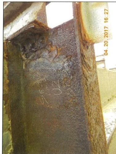
Span 3 Floorbeam 2 Rt deterioration
