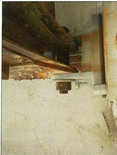
Span 1 L0 Rt bottom exterior packrust
