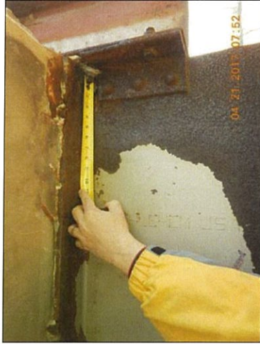
Span 2 Floorbeam 9 Rt hole
