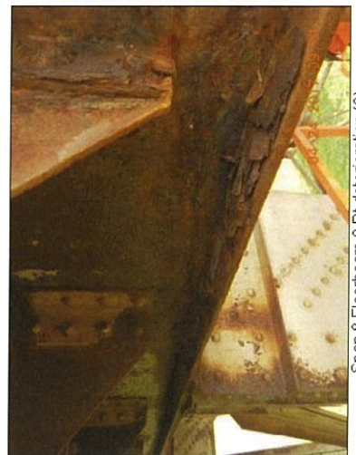
Span 8 Floorbeam 0 Rt deterioration (2)
