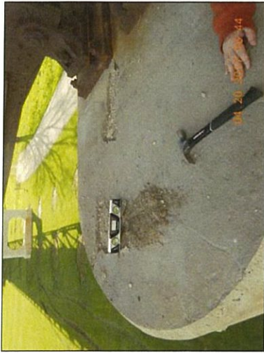
Pier 2 South cap deterioration closeup
