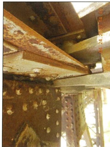
Span 8 L0 Lt bottom interior packrust
