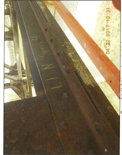
Span 3 L1L2 Lt packrust at L1
