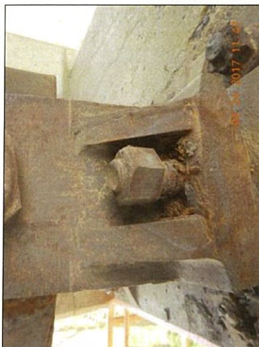
Span 7 L0 Rt interior anchor bolt deterioration
