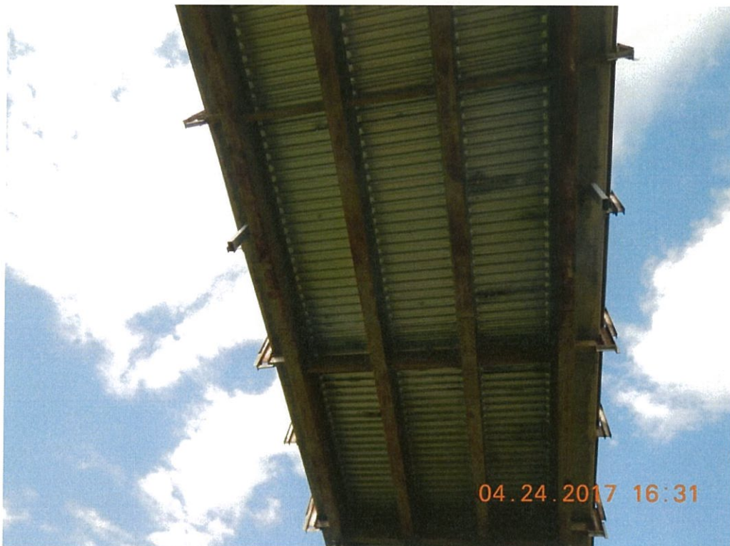
Photo 10: A few seam locations of the stay-in-place decking in Spans 9 through 11 are showing rust. Span 9 shown.
