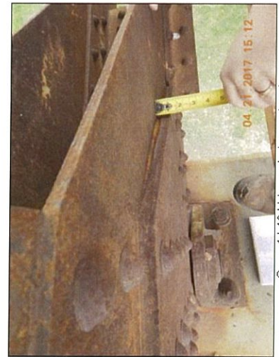
Span 1 L10 Lt top exterior packrust
