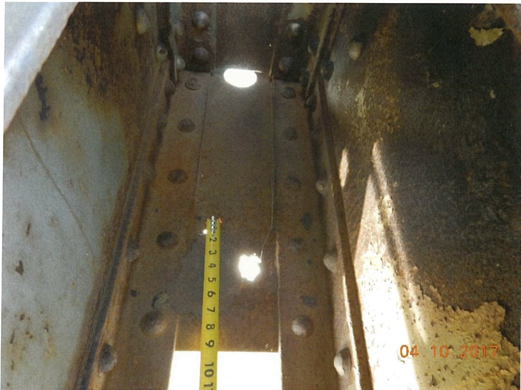
Photo 87: The thru truss lower lateral bracing gusset plates have corrosion and packrust; the L1' and L2' have significant section loss with holes forming. Span 6 L1' Lt. shown.
