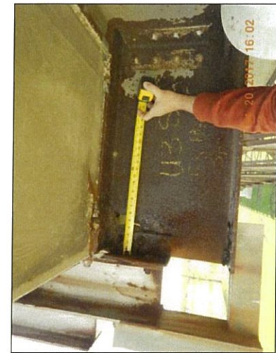
Span 3 Floorbeam 3 Rt deterioration
