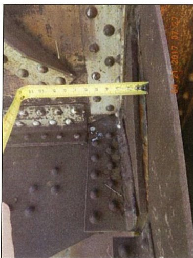
Span 3 L10 Rt top interior packrust (2)
