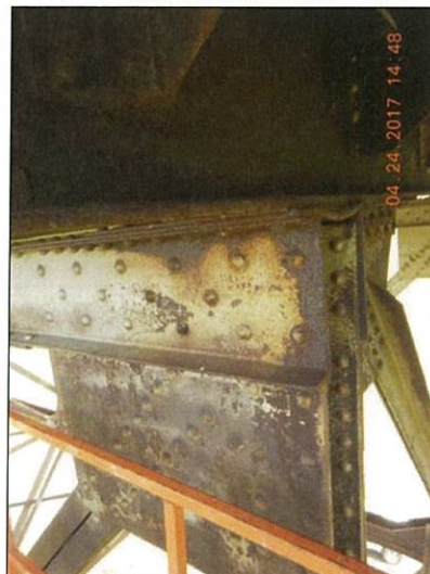
Span 8 U0 Lt exterior deterioration
