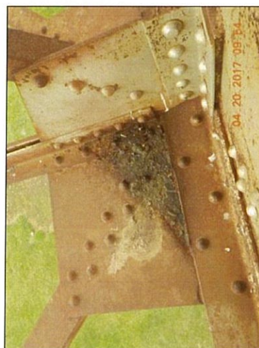
Span 2 L8 Lt horizontal gusset plate deterioration
