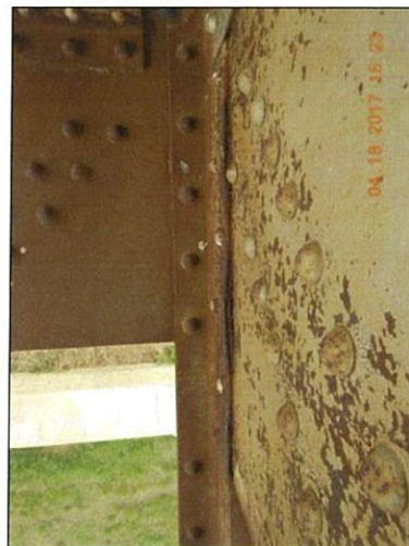
Span 3 L9 Lt interior packrust
