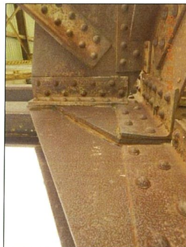
Span 2 L10 Lt top interior plate packrust and deterioration
