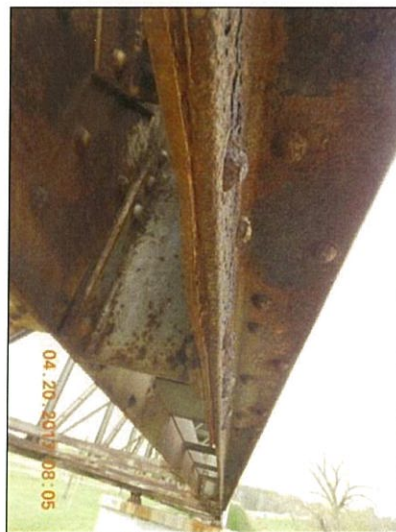
Span 3 L4 Lt bottom packrust
