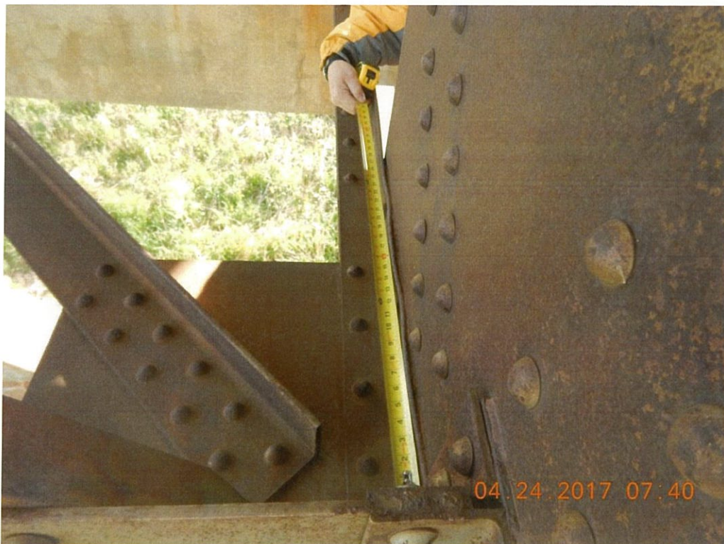
Photo 30: Minor packrust up to 1/4" is typical at the members coming into the deck truss lower connection gusset plates, excluding the end connections. Span 8 L9 Rt. interior shown.
