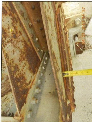
Span 1 L0 Rt top exterior packrust
