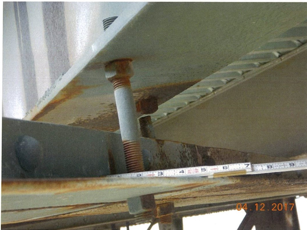
Photo 82: Some of the thru truss lower lateral bracing hanger bolts used to minimize vibrations of the bracing are sheared off.
