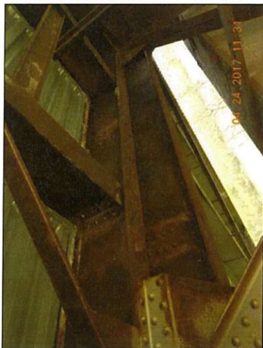
Span 7 Floorbeam 0 interior deterioration
