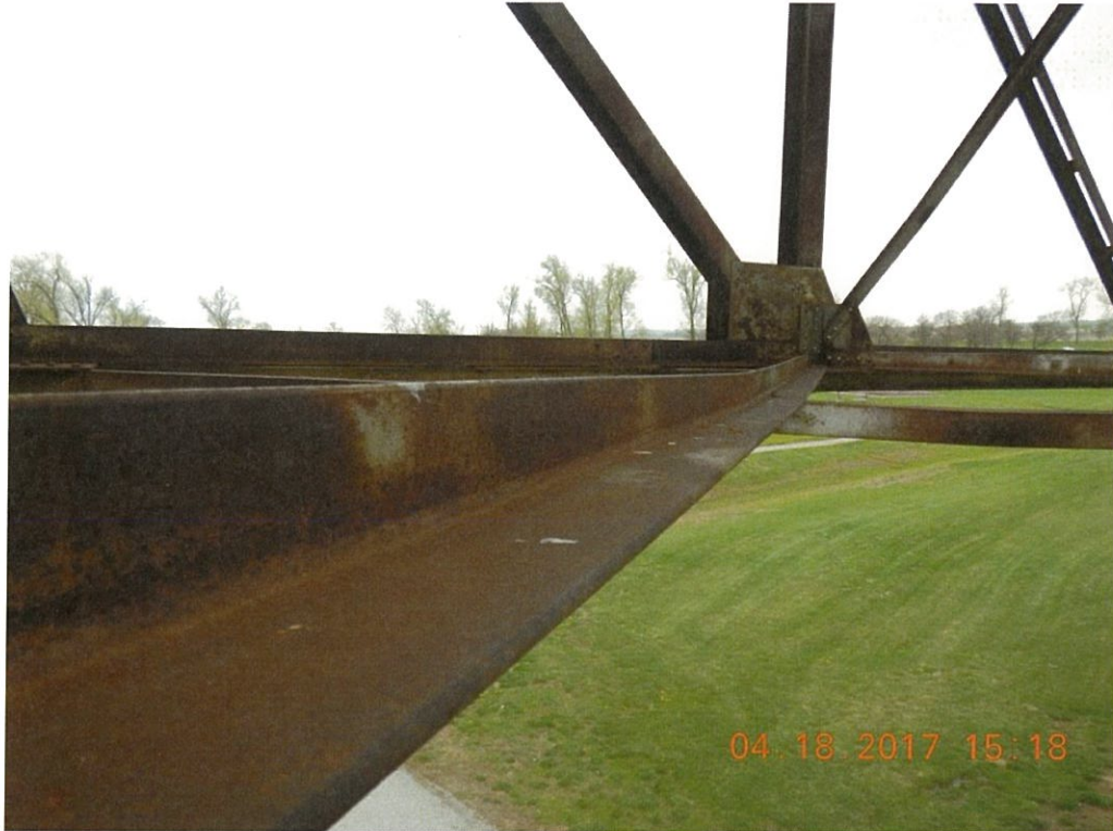
Photo 67: Deck truss lower lateral bracing is bent at Span 3 Bay 9.
