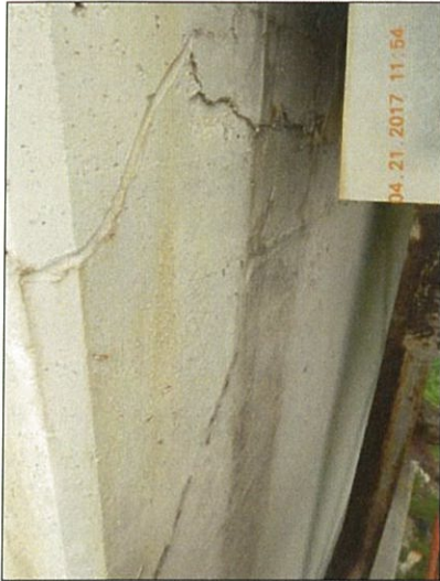
Abutment 1 South water marks from joint leakage
