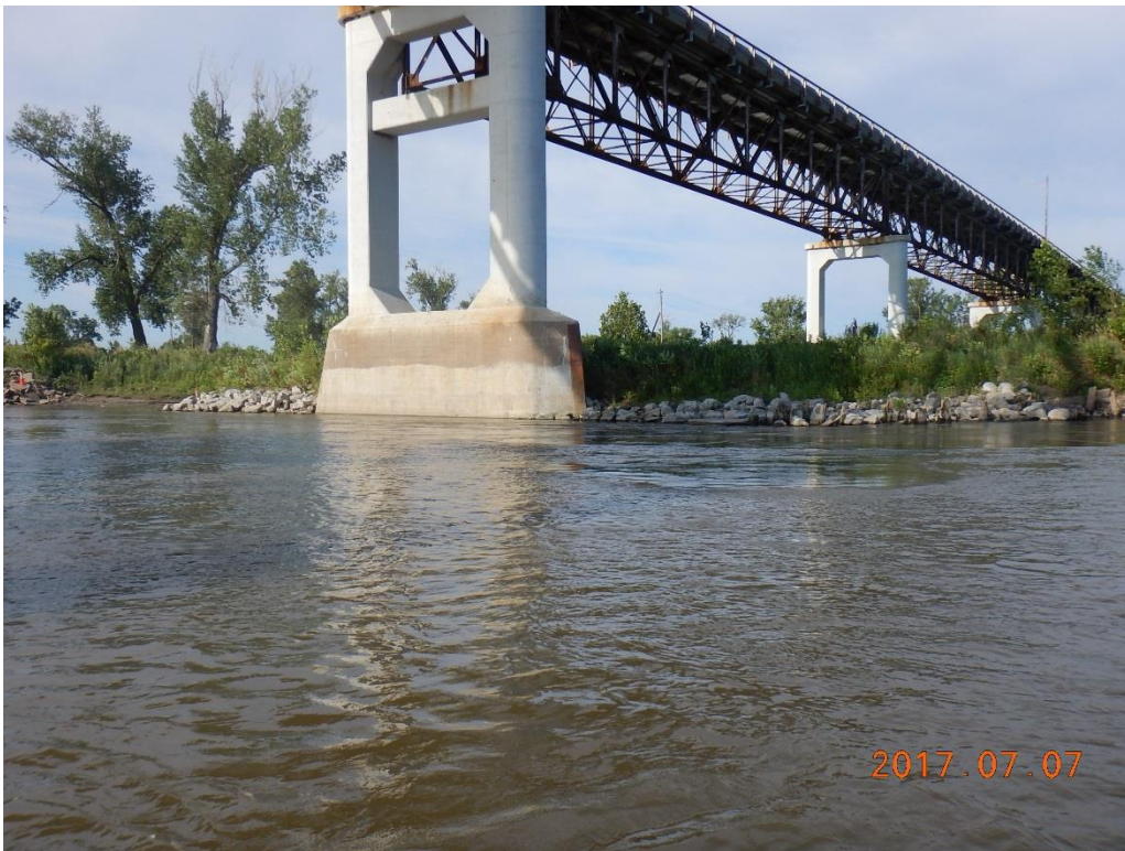
Pier 4 – Riprap Placed to Repair Scour
