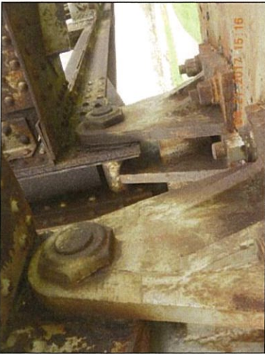
Span 2 L0 Lt interior pin packrust
