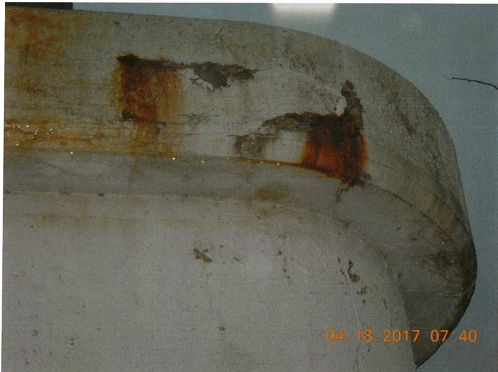
Photo 118: Spalling with heavy rust staining on the vertical face of the Pier 1 cap at the north and south ends. Northeast corner shown.
