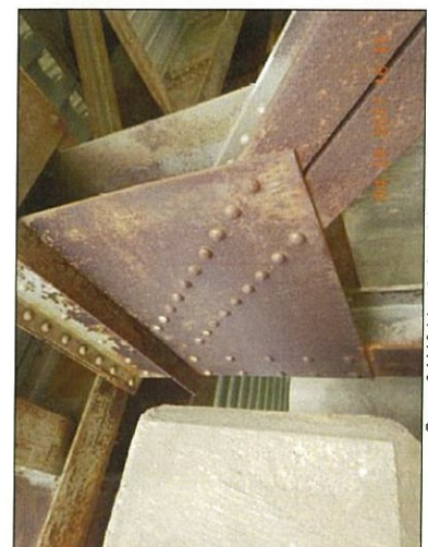
Span 8 U10 Lt exterior deterioration
