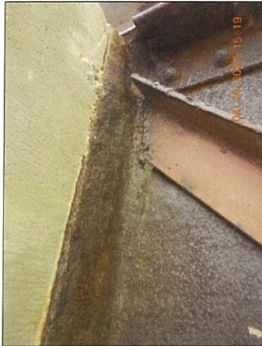
Span 8 Floorbeam 4 Lt top stiffened weld crack on East
