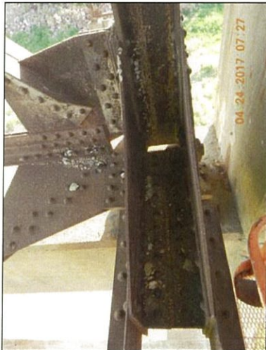
Span 8 L10 Rt top deterioration
