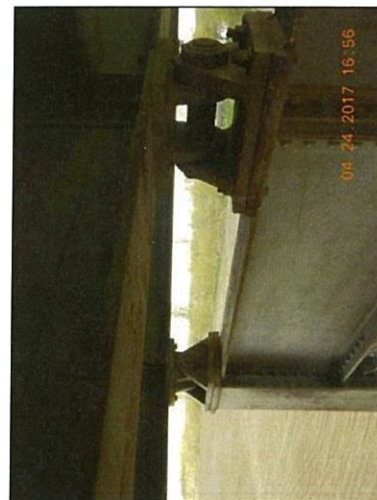
Bearings Pier 9 Girders 3 and 4
