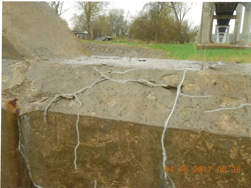
Photo 128: The top of the Pier 8 bottom wall is scaling which is creating spalls around some of the cracks; larger spalls are present at the southwest corner and east faces of the wall. East face shown.
