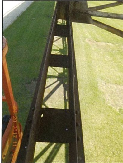
Span 2 L0L1 Lt batten plate deterioration from top
