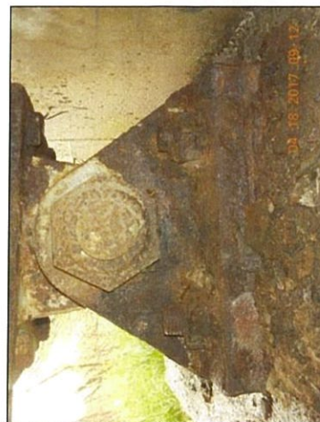
Span 11 Abutment 2 Girder 1 bearing looking North - interior nuts and bolts deterioration
