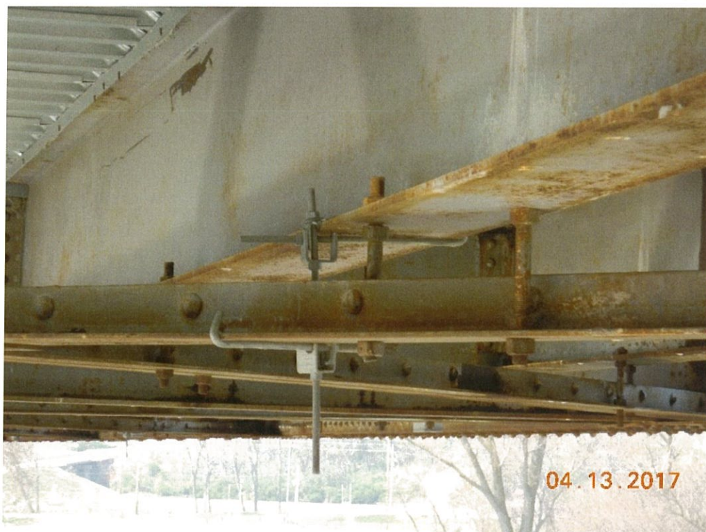
Photo 83: New thru truss lower lateral bracing hanger rods have previously been installed at some locations near Pier 5 and appear to be functioning as intended.
