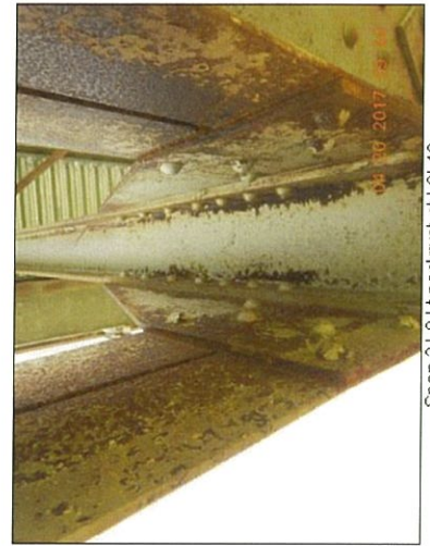
Span 2 L9 Lt packrust at L9L10
