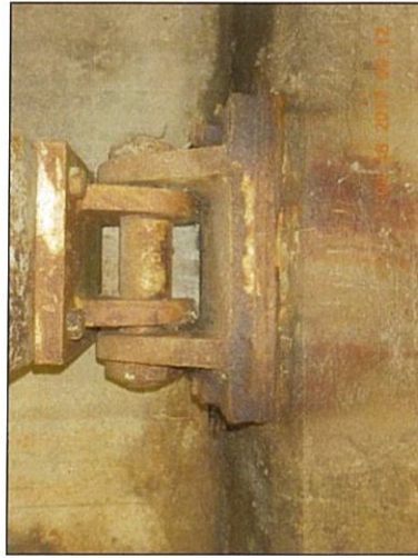
Span 11 Abutment 2 Girder 2 bearing
