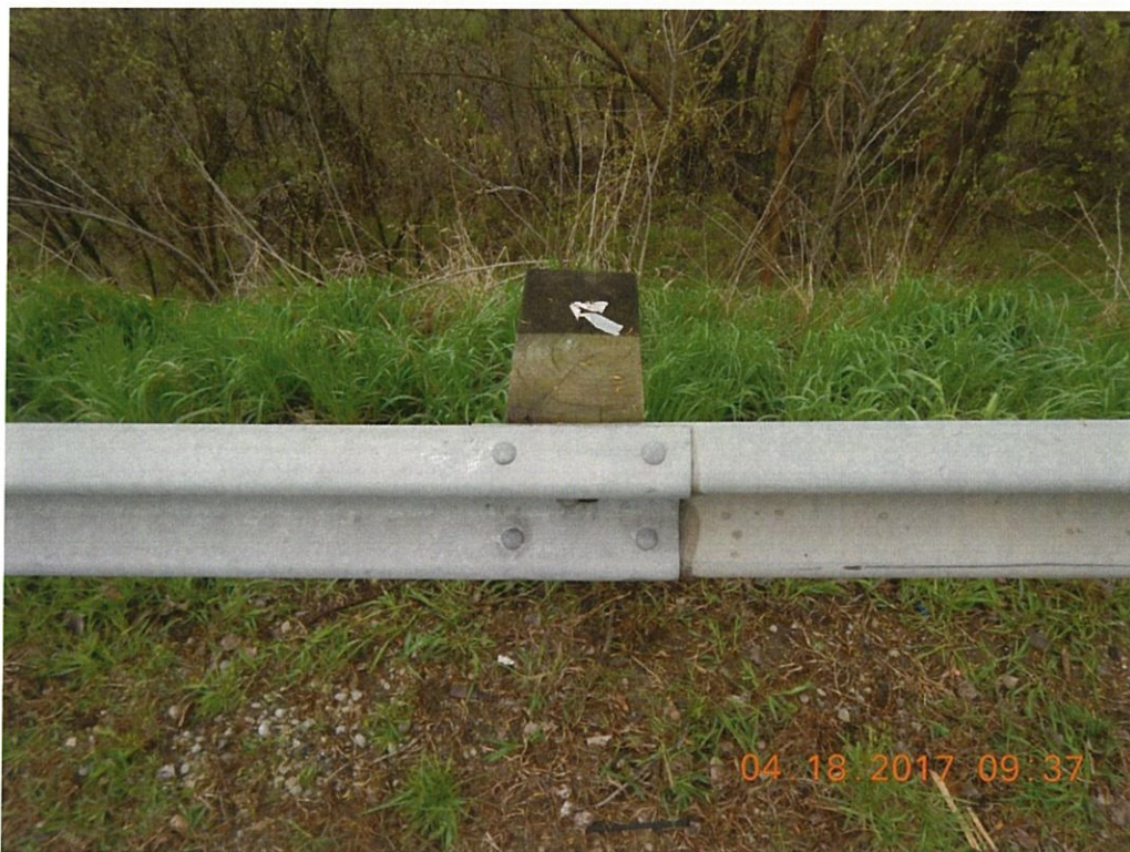
Photo 20: There are locations of improper rail splice lapping in both east approach rails.
