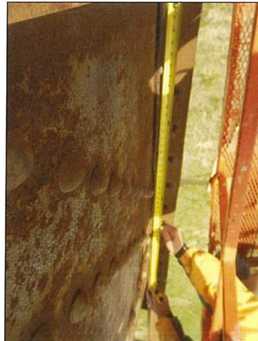
Span 4 L9 Rt exterior packrust
