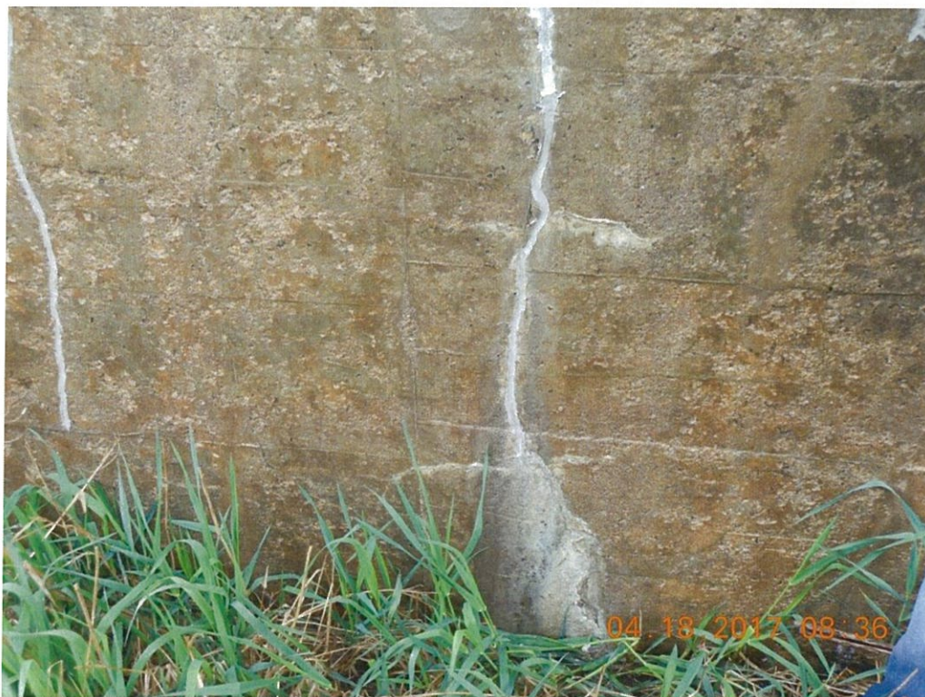
Photo 130: Efflorescence is present at the west face of the Pier 8 bottom wall.
