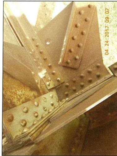
Span 8 L0 Rt horizontal gusset plate deterioration
