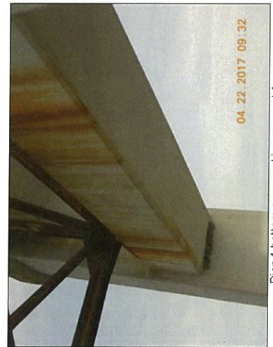
Pier 4 bottom cap cracking on west face
