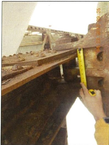
Span 4 L10 Rt bottom exterior packrust
