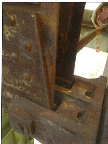
Span 7 L0 Rt bottom exterior packrust
