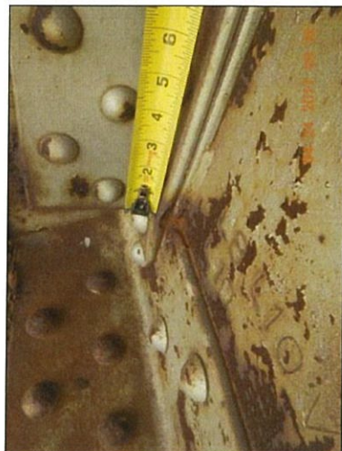
Span 7 L10 Rt top interior deterioration
