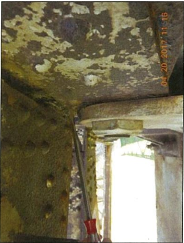
Span 2 L0 Lt bottom of horizontal gusset plate packrust
