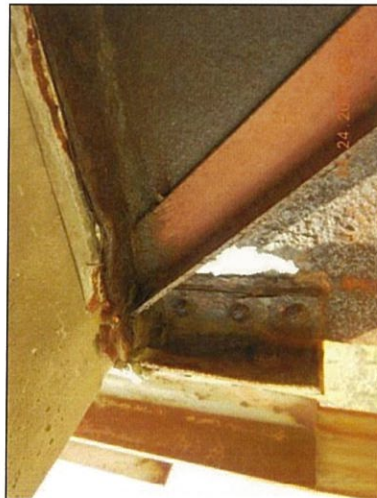
Span 7 Floorbeam 8 Rt top flange loss
