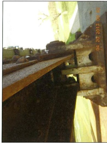
Span 3 L0 Lt exterior bottom plate packrust
