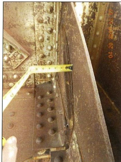
Span 3 L10 Rt top interior packrust
