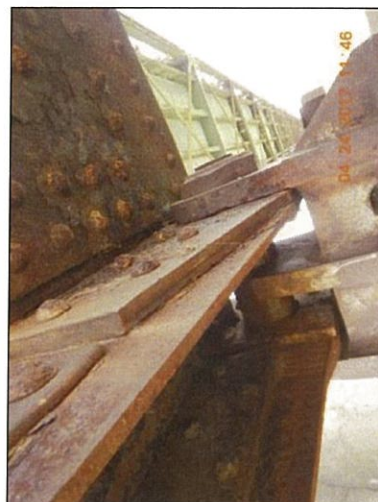
Span 7 L0 Rt bottom interior packrust
