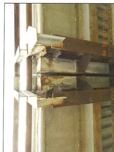
Span 3 U10 Rt deterioration below deck joint
