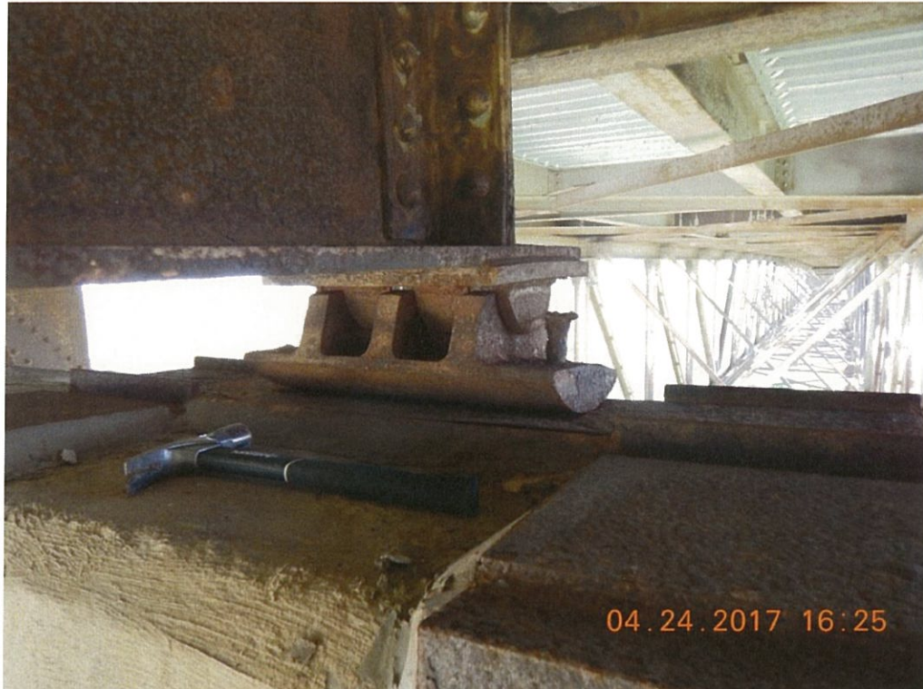
Photo 111: The south anchor bolt at Span 9 Girder 2 is missing at the Pier 8 bearing and the north has no nut.
