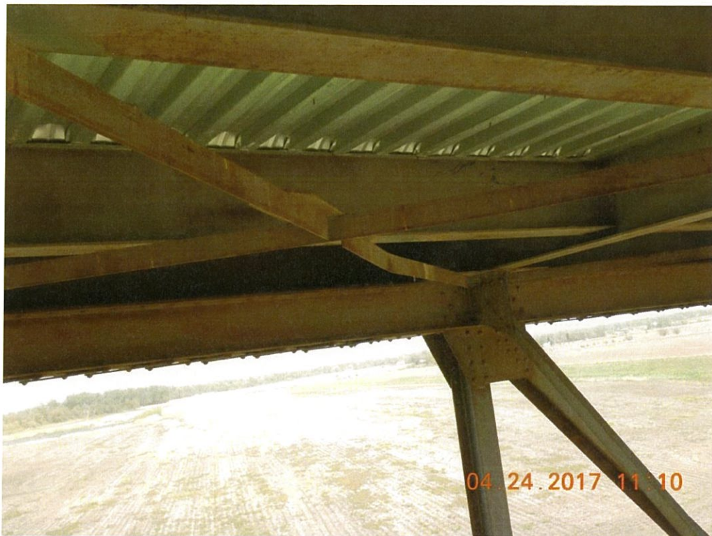
Photo 68: Deck truss upper lateral bracing is bent at Span 7 Bay 3.
