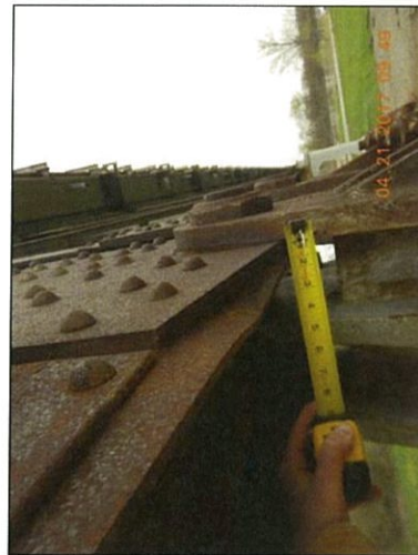
Span 1 L10 Rt bottom exterior packrust
