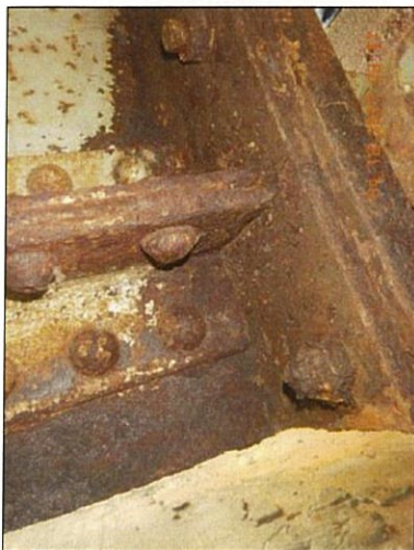
Span 11 Abutment 2 Girder 4 interior face deterioration
