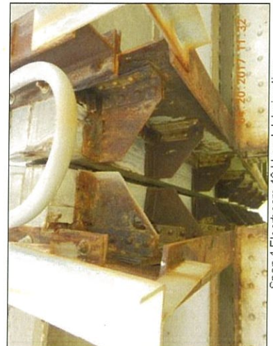
Span 1 Floorbeam 10 Lt end deterioration
