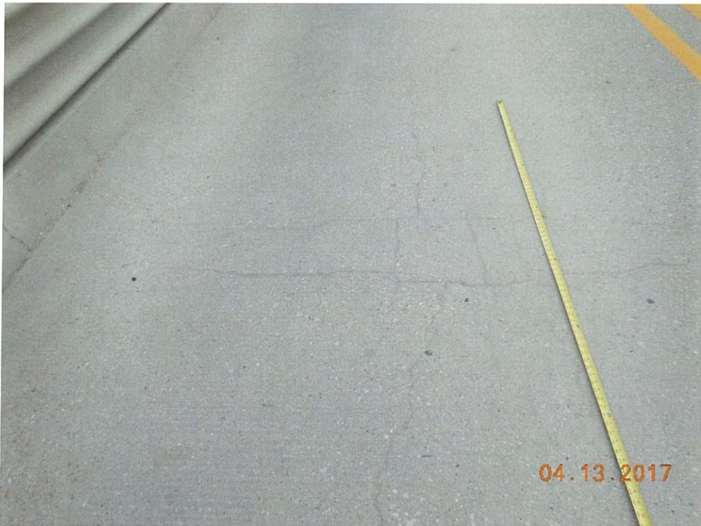
Photo 7: Where the deck is continuous over a floorbeam there is transverse cracking.
