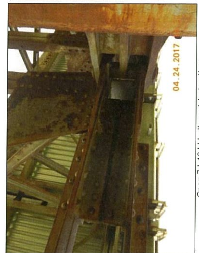
Span 7 L10 Lt bottom deterioration
