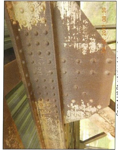
Span 4 U6 Rt exterior deterioration
