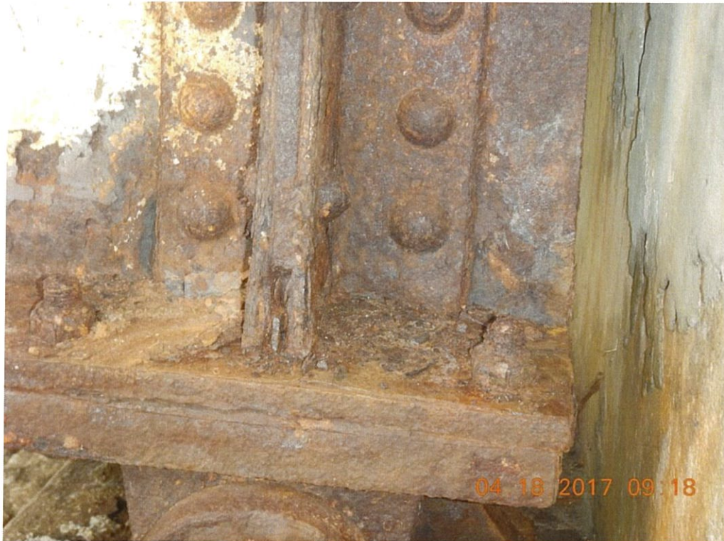
Photo 103: The leaking joints at above the ends of the girders have caused heavy rust with some section loss in the girder webs. Girder 4 exterior face at Abutment 2 shown.
