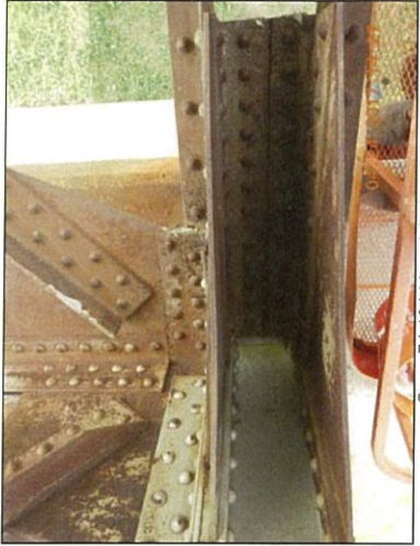
Span 7 L10 Lt top deterioration
