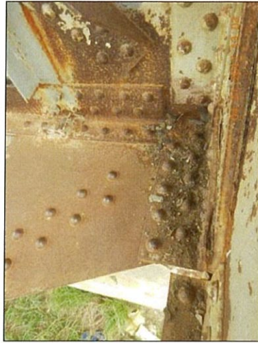
Span 1 L0 Lt top interior packrust
