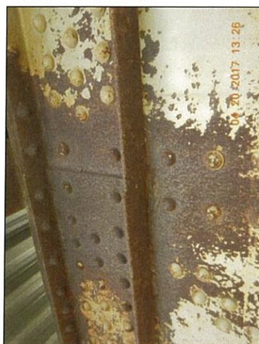
Span 3 U8 Rt exterior channels not lined up
