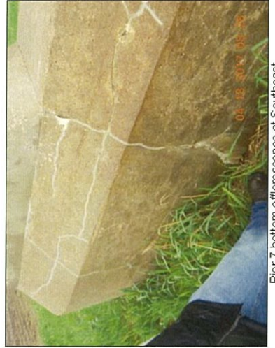
Pier 7 bottom efflorescence at Southeast
