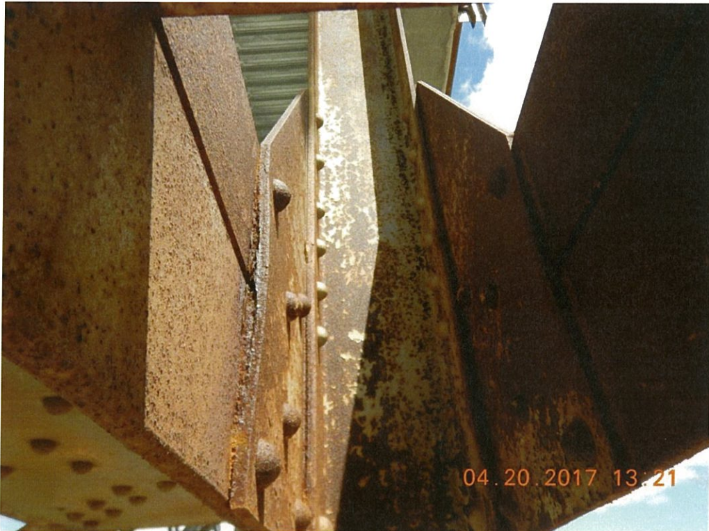
Photo 31: Minor packrust up to 1/4" is typical at the members coming into the deck truss lower connection gusset plates, excluding the end connections. Span 3 L8 Rt. west inside shown.
