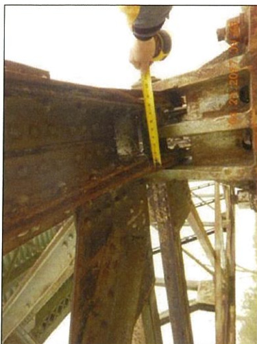
Span 1 L10 Rt gussets bent inward
