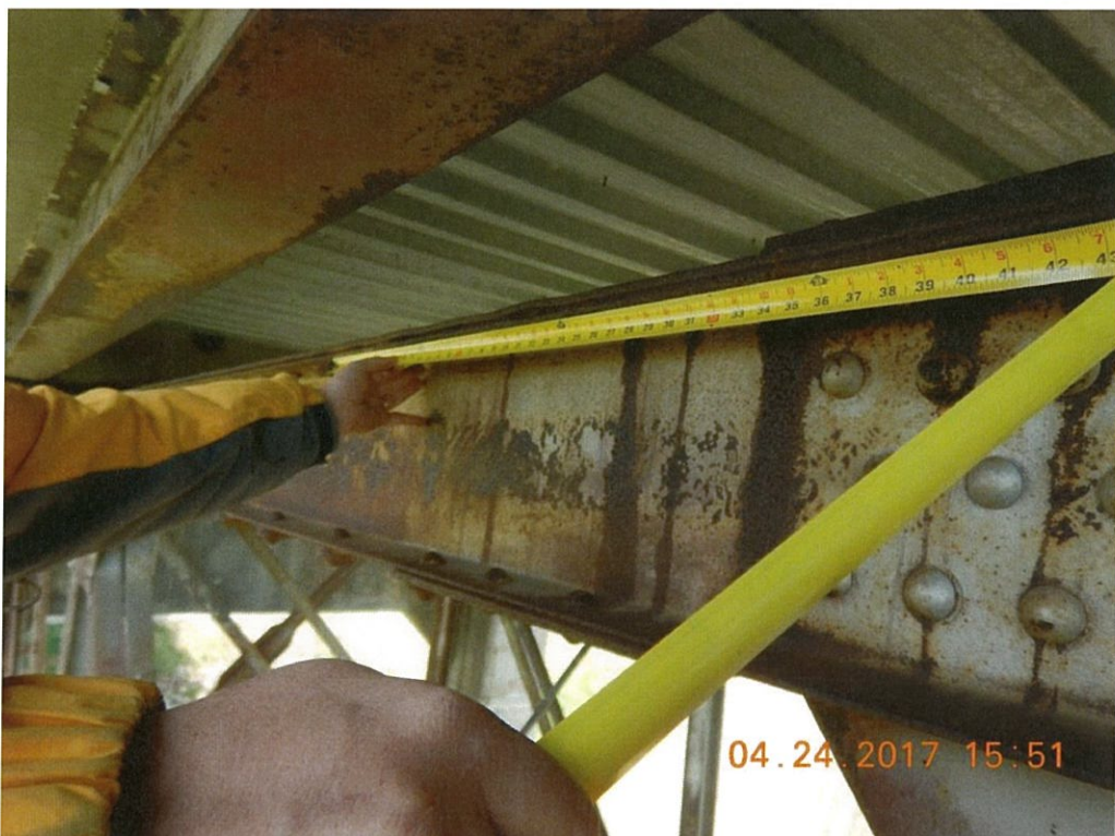
Photo 33: Minor packrust up to 1/4" is typical at the cover plate of the deck truss upper chords which produces a ripple distortion along the rivets. Span 8 U8U9 Lt. shown.
