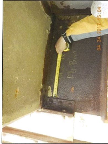
Span 8 Floorbeam 2 Lt hole
