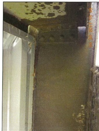
Span 3 Floorbeam 4 Stringer 4 deterioration
