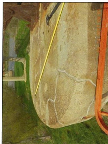
Pier 7 South top deterioration
