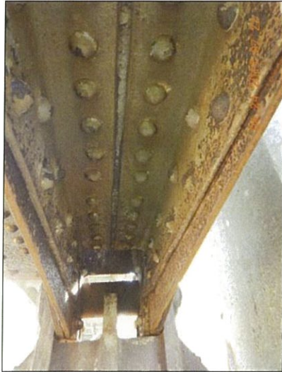
Span 8 L10 Rt bottom deterioration
