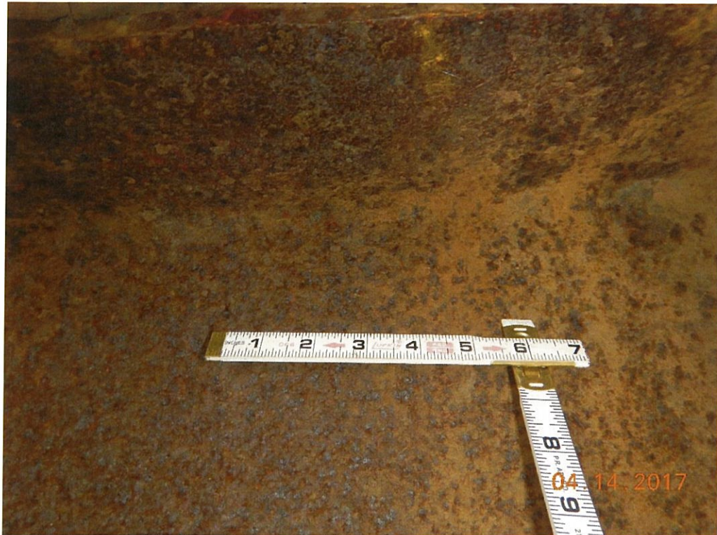
Photo 91: The thru truss floorbeam corrosion showing web to top flange.
