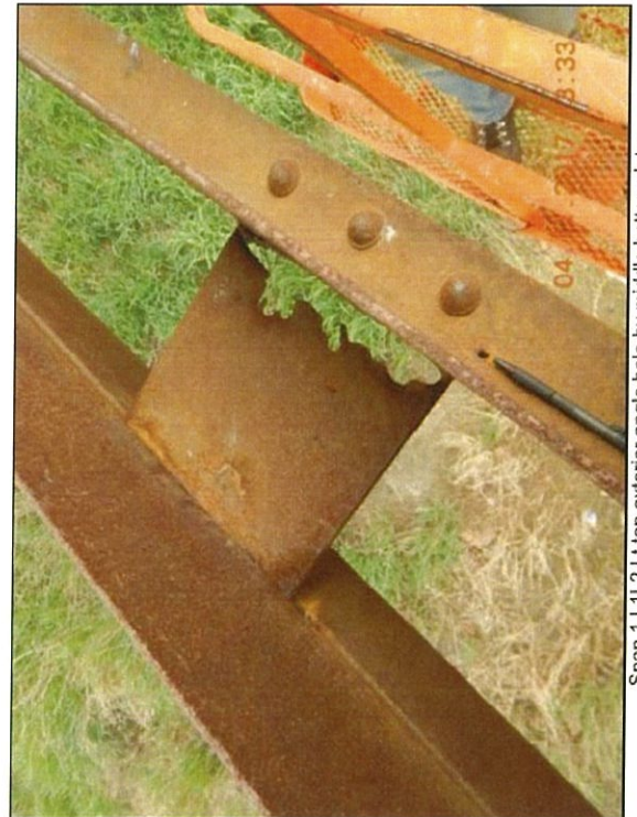
Span 1 L1L2 Lt bottom interior angle hole below middle batten plate
