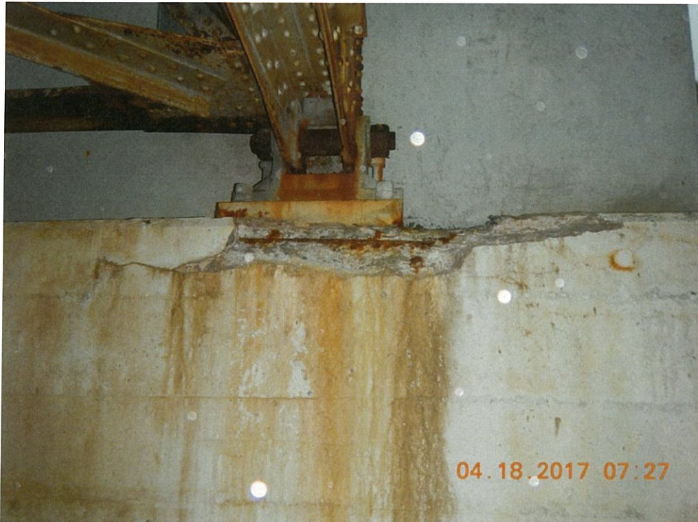
Photo 115: The front edge of Abutment 1 under the north bearing is spalled approximately 6" by 6" for nearly 3' – back edge of spall is at front edge of the bearing.
