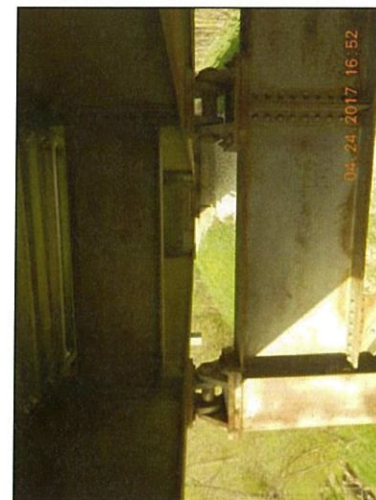
Bearings Pier 10 Girders 1 and 2
