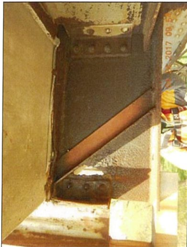
Span 7 Floorbeam 8 Rt stiffened and hole
