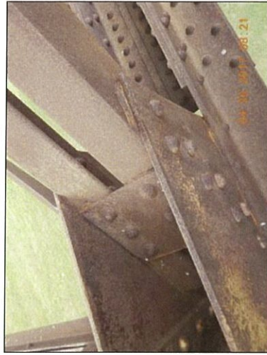
Span 3 L4 Lt packrust
