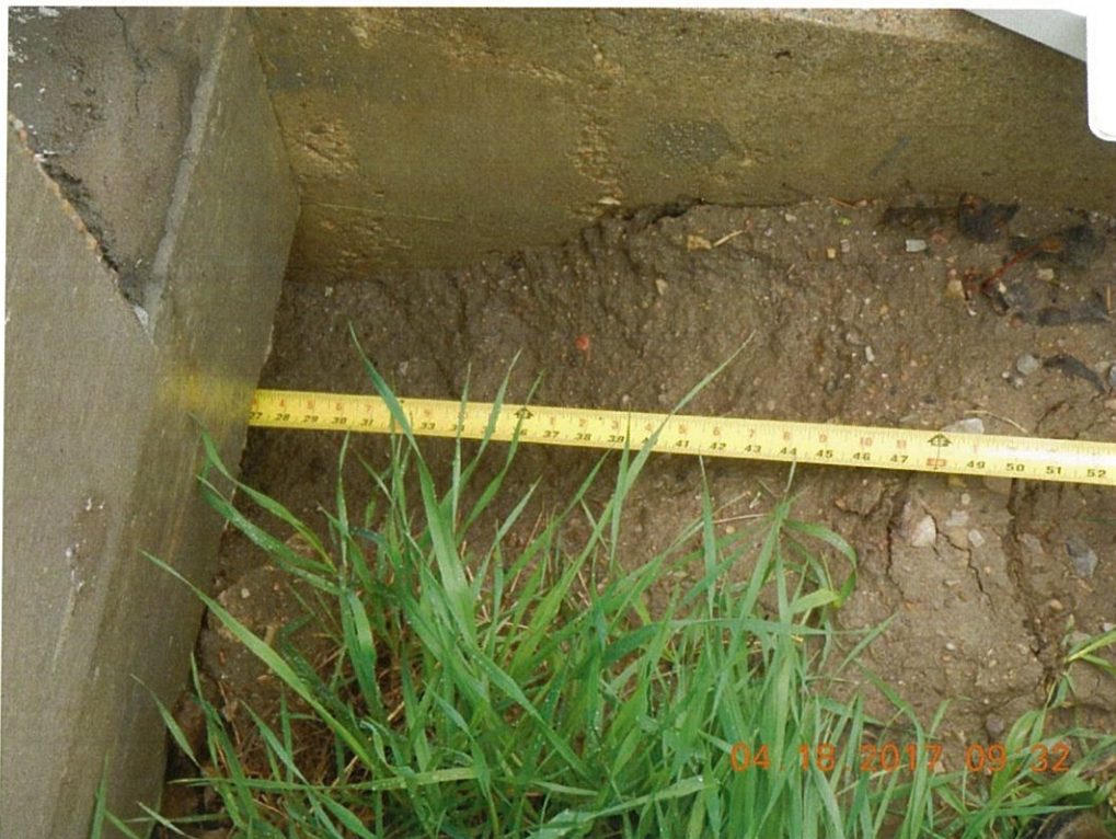
Photo 12: The east approach slab is undermined adjacent to the north barrier wall in two spots. Shown is at the abutment the penetration is approximately 6" tall by 4' wide x 3' below the slab.
