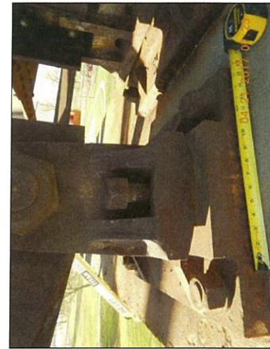
Span 3 L0 Lt exterior anchor bolt bent
