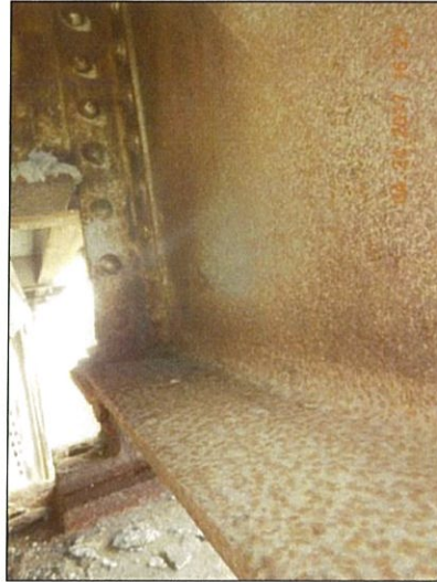
Span 9 Girder 1 interior deterioration at Pier 8
