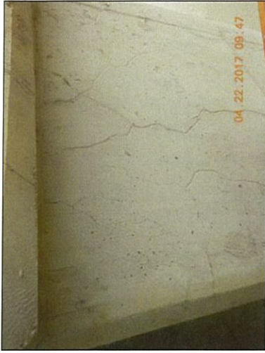
Pier 4 south west face cracking
