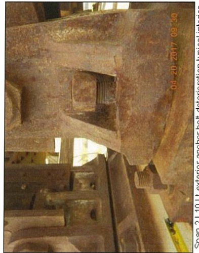
Span 2 L10 Lt exterior anchor bolt deterioration typical interior
