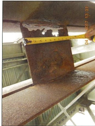
Span 1 L1L2 Lt middle batten plate hole
