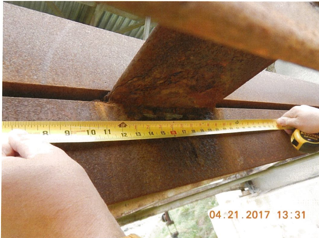
Photo 27: The worst case of the deck truss lower chord loss is at the middle batten plate of Span 1 L1L2 Lt. Complete section loss in the interior angle for approx. 5" in length and 1" in depth.
