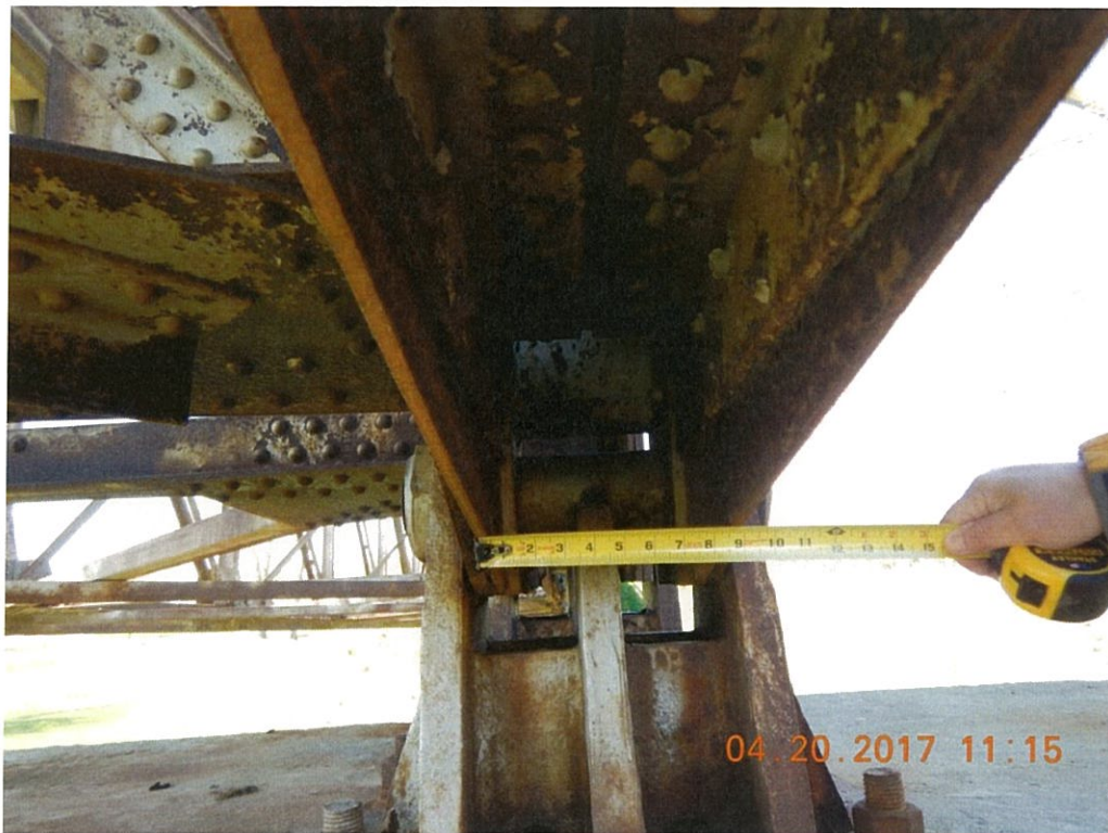
Photo 44: The lower chord gusset plates at the deck truss bearings are typically bowed inward at the bottom. Span 2 L0 Lt. shown.
