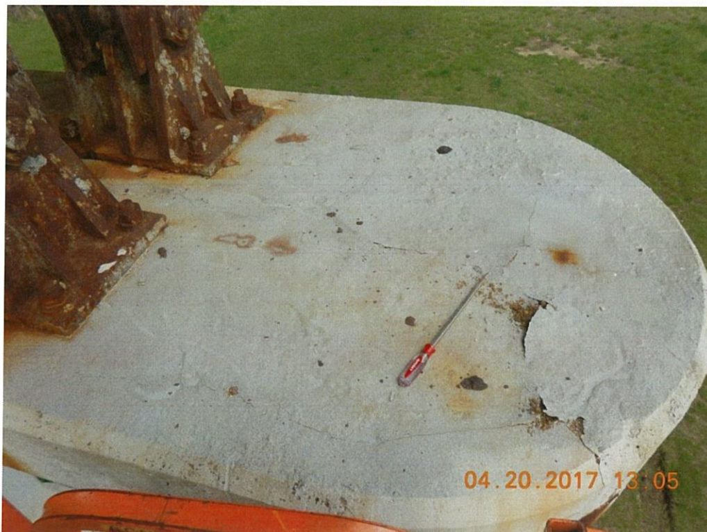
Photo 122: The top of the Pier 3 cap has minor sealant coat deterioration with plain sand and aggregate underneath it at the south end.
