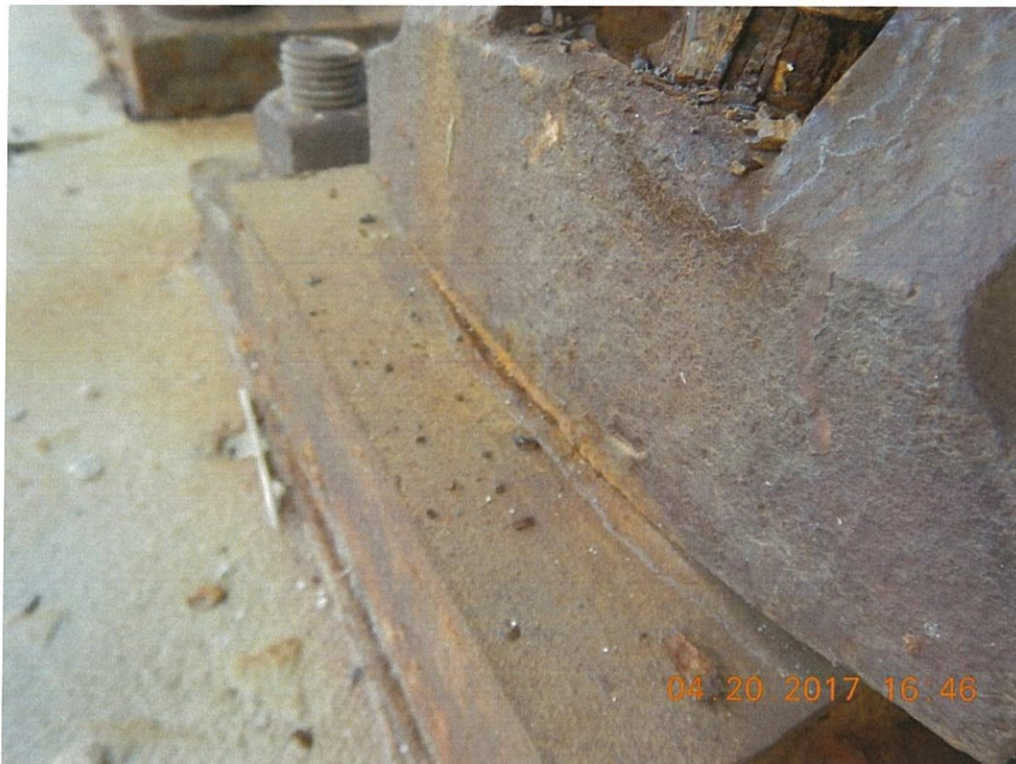
Photo 104: All the expansion bearings have wearing marks indicating movement through the temperature range. Span 3 L0 Rt. shown.
