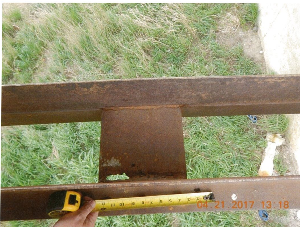
Photo 23: The loss shown in Photos 21 and 22 does also go into some batten plates with holes having formed in the middle batten plates of Span 1 L0L1 Lt.
