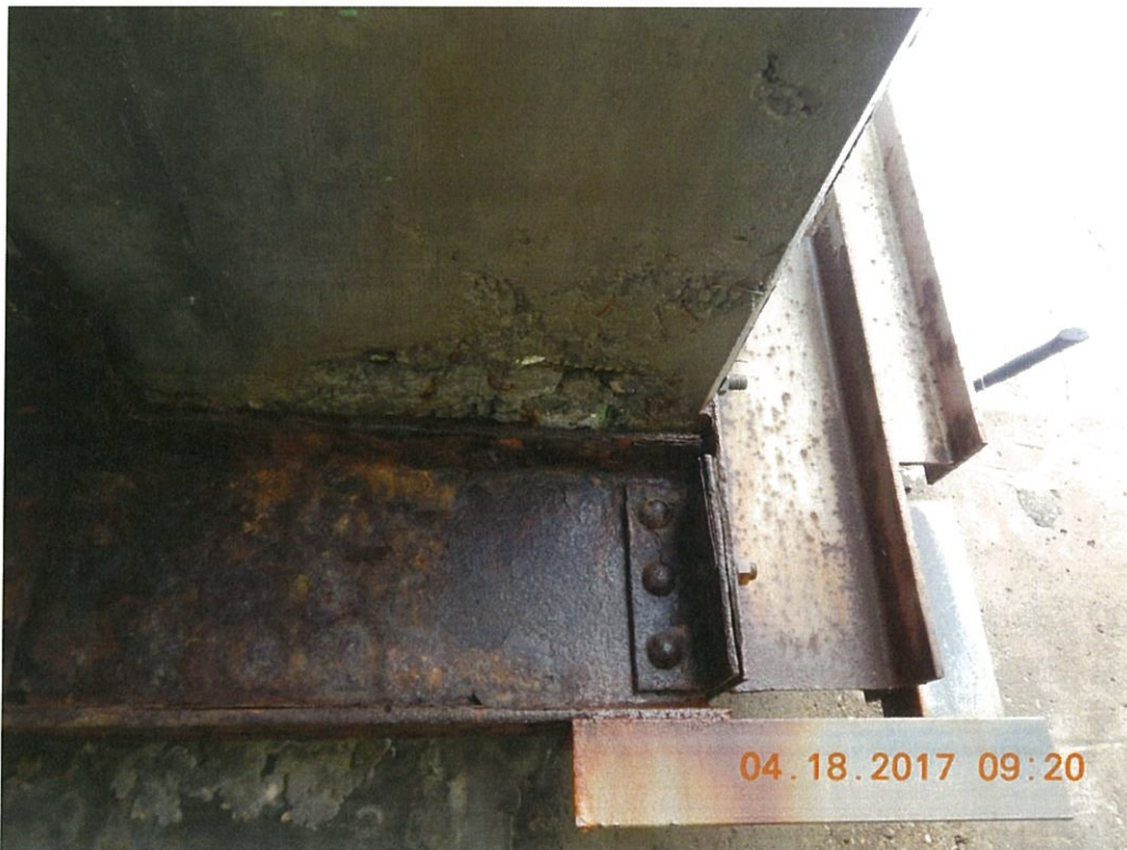
Photo 8: Poor consolidation of the concrete during construction has left exposed rebar at the bottom of the deck overhang at both corners of the East Abutment. South corner shown.
