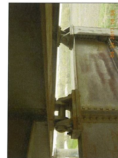
Bearings Pier 9 Girders 1 and 2
