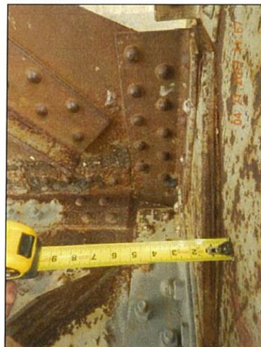
Span 1 L0 Rt top interior packrust
