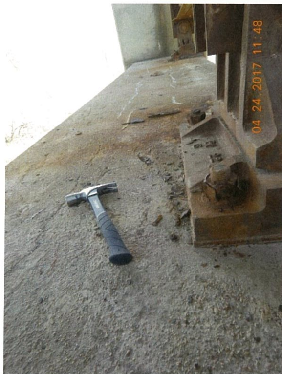
Photo 124: There is delamination of the Pier 6 cap behind the Span 7 south bearing.
