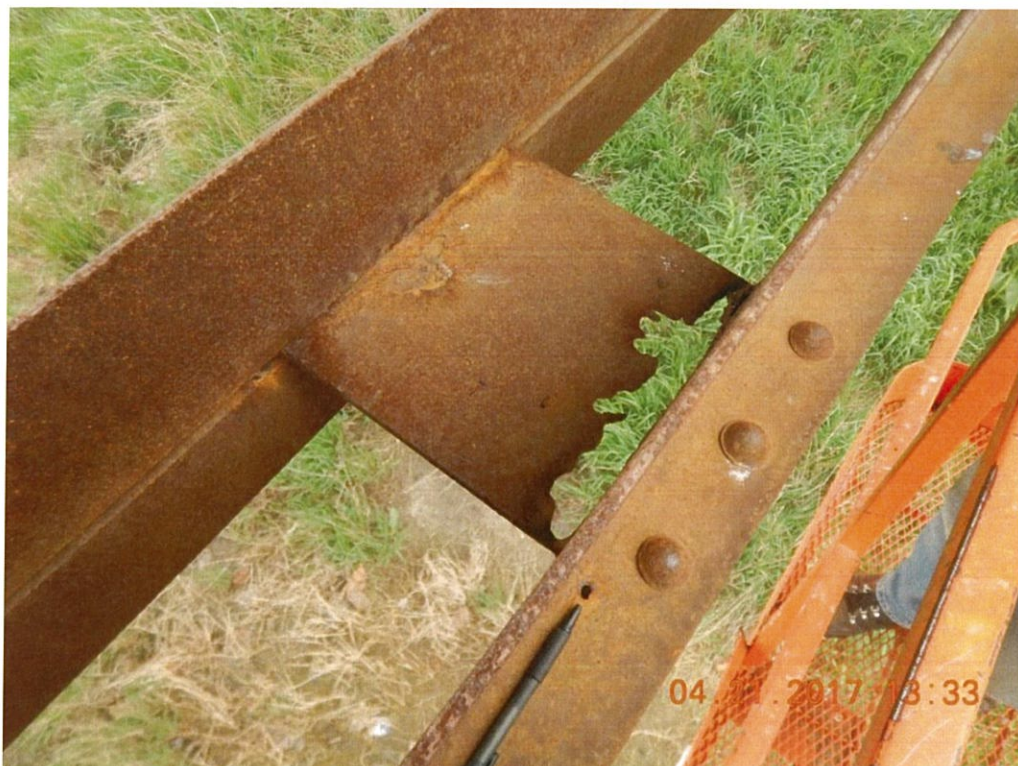
Photo 24: Similar loss in Span 1 L1L2 Lt. middle batten plate as shown in Photo 23. There is also a small \frac{1}{4} " diameter hole in the horizontal leg of the top exterior angle of this member.
