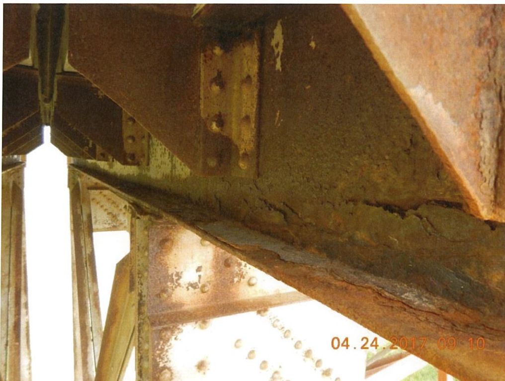
Photo 57: There are areas of delamination in the deck truss floorbeam faces below the deck joints. Span 8 Floorbeam 0 Rt. end shown.
