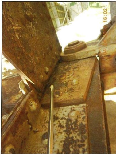
Span 8 L10 Lt bottom interior deterioration
