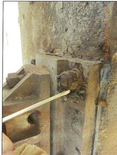
Span 7 L0 Rt bearing nut deterioration
