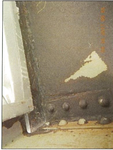
Span 7 Stringer 4 at U8 connection loss on East
