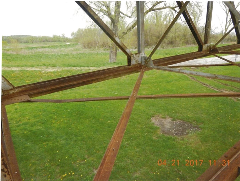
Photo 64: Deck truss lower lateral bracing is bent at Span 1 Bay 3 and 4; note Bay 3 is the closest bay shown in the photo.
