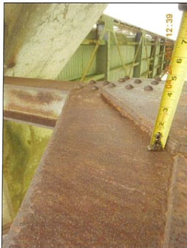
Span 7 L0 Lt top exterior packrust
