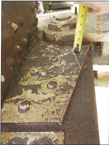
Span 2 L0 Rt interior pin packrust
