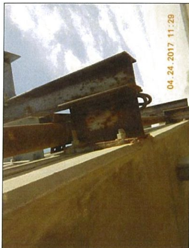
Span 7 Rail post near U0 bracket was loose - removed at ...
