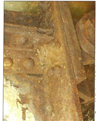
Span 11 Abutment 2 Girder 4 exterior face deterioration
