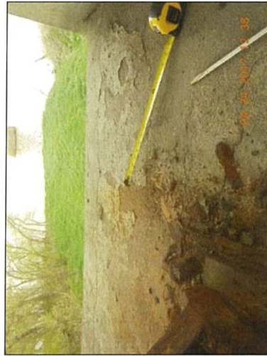
Pier 6 cap deterioration near Span 7 L0 Lt
