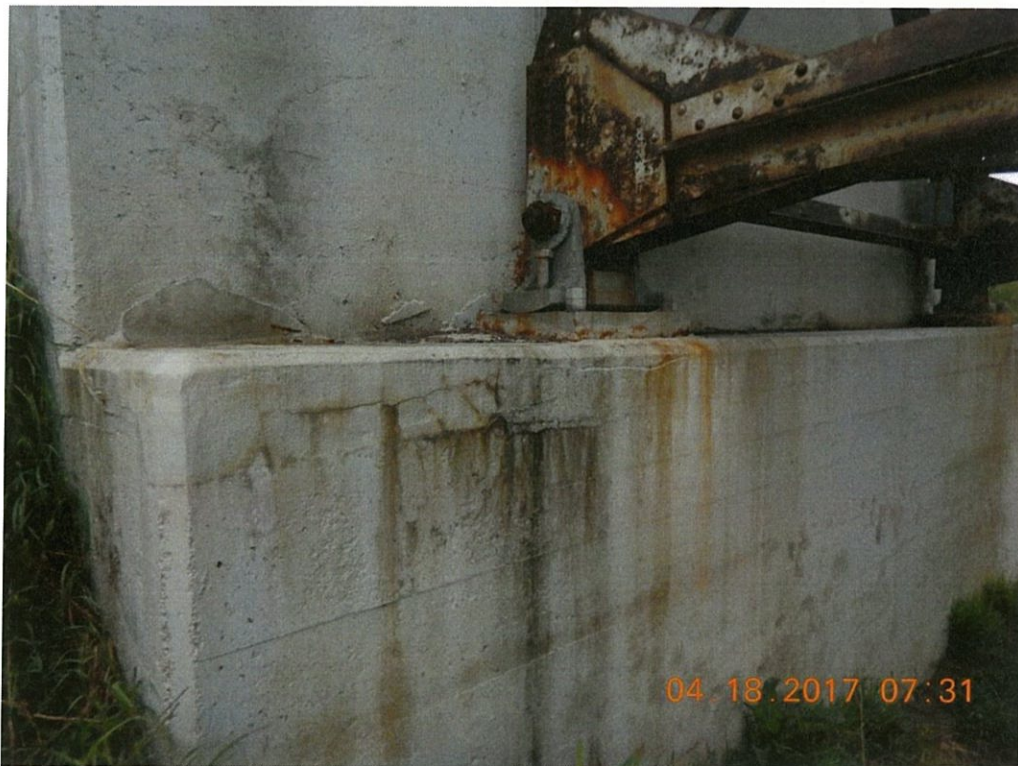
Photo 116: The front edge of Abutment 1 under the south bearing is delaminating from the south corner to the bearing 2.
