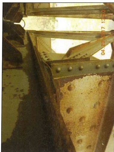
Span 3 U10 Rt end packrust
