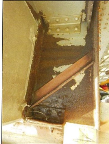
Span 7 Floorbeam 4 Rt stiffened and hole
