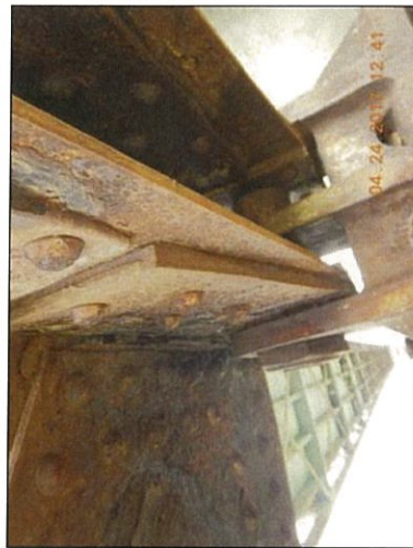
Span 7 L0 Lt bottom interior packrust
