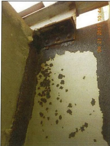
Span 1 Floorbeam 5 Rt heavy deterioration
