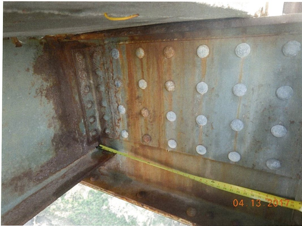
Photo 89: Typical thru truss floorbeam web repair.
