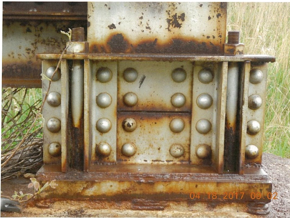
Photo 133: Heavy packrust has developed between the steel column anchor bolts and their stiffeners; there is section loss on some bolts. East bolts at the north column shown.
