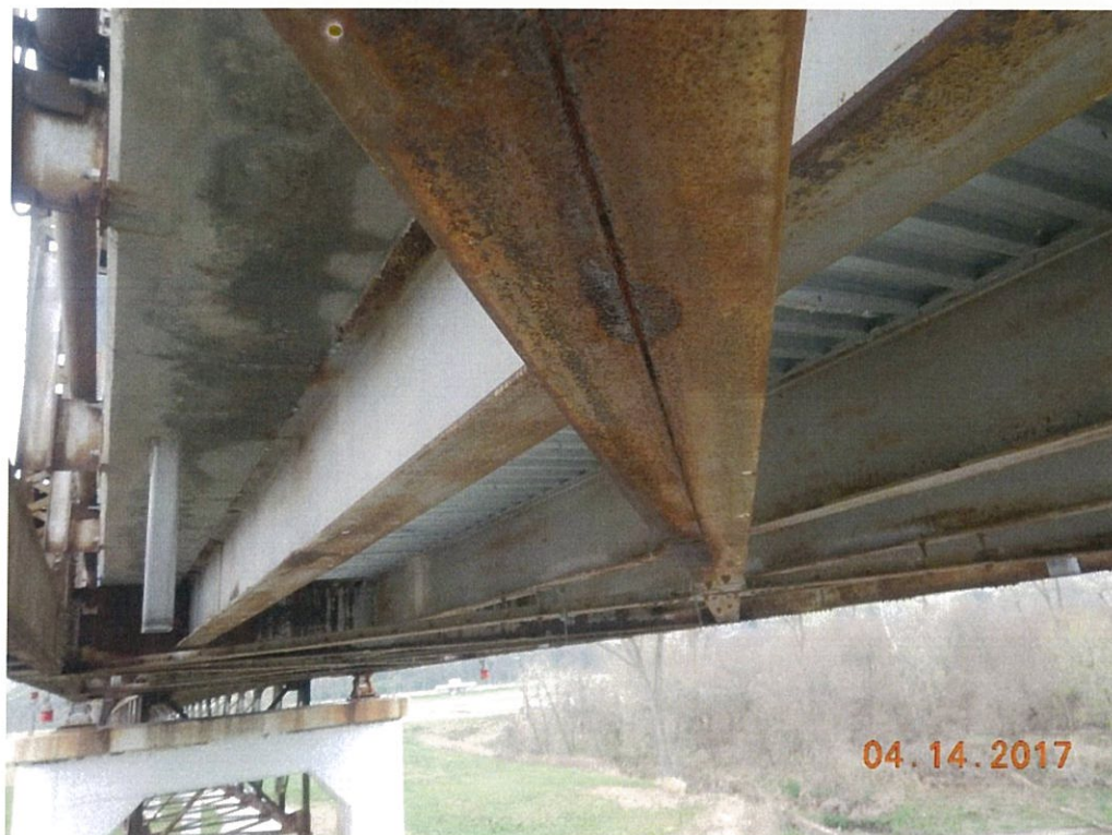
Photo 84: Span 5 lower lateral bracing from L2 Lt. to L3 Rt. is bent.
