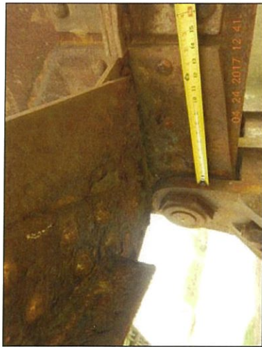
Span 7 L0 Lt bottom interior deterioration
