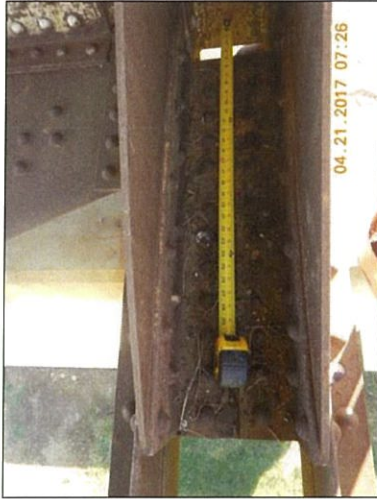
Span 2 L 10 Rt inside deterioration
