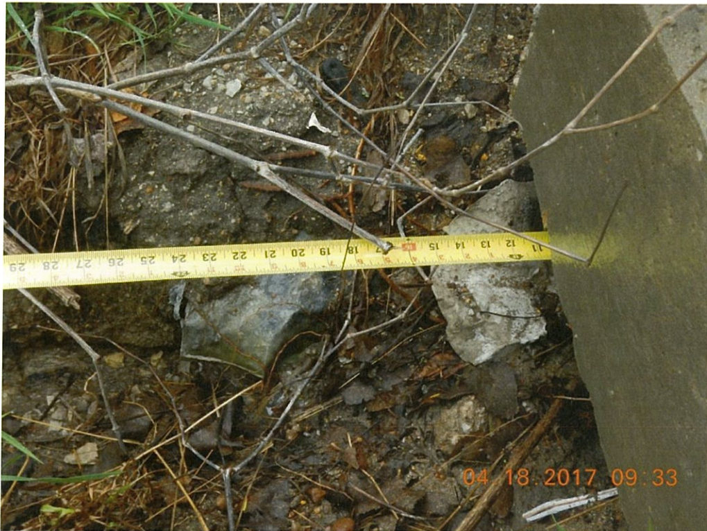
Photo 13: The east approach slab is undermined adjacent to the north barrier wall in two spots. Shown is at the end of the slab where the ditch is eroding is the penetration is approximately 6" tall by 2' wide by 2' below the slab.
