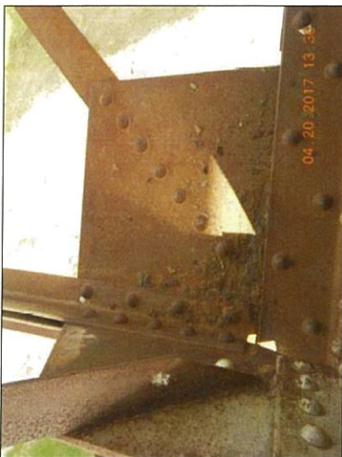
Span 3 L7 Rt horizontal gusset plate deterioration
