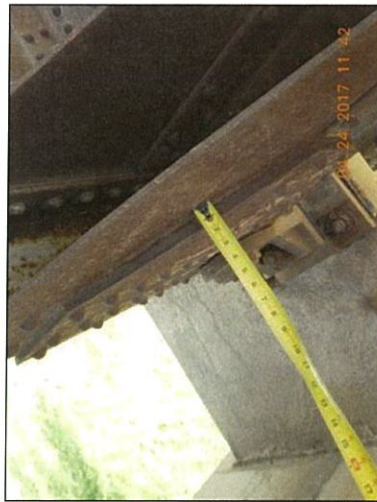
Span 7 L0 Rt top exterior packrust
