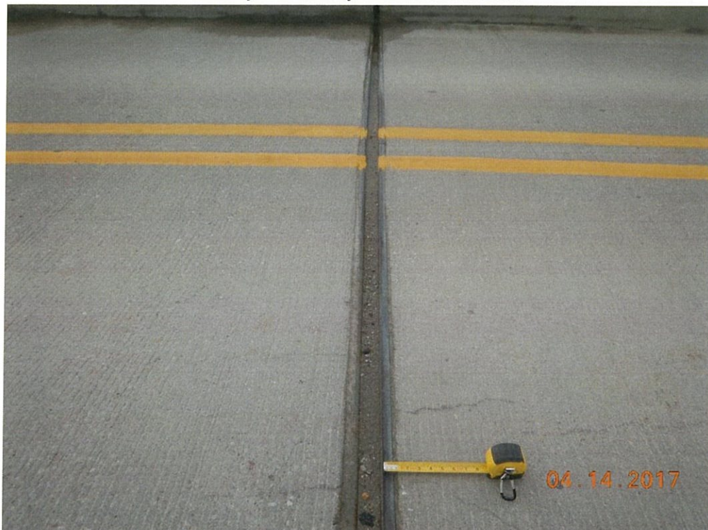
Photo 14: All of the strip seal joints are full of debris.
