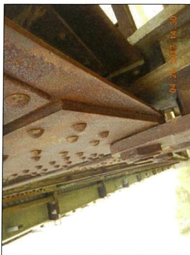
Span 7 L10 Lt bottom exterior packrust
