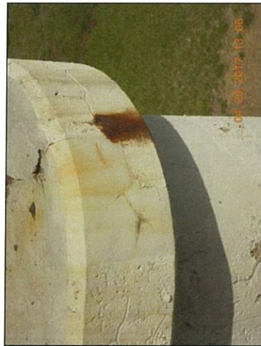
Pier 3 South cap cracking on West
