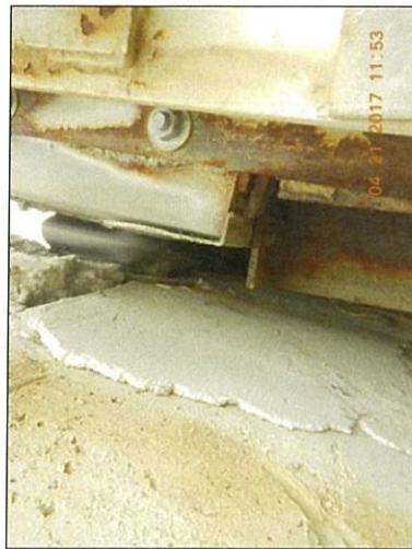
Abutment 1 South deck joint holes
