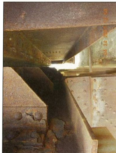
Span 7 Floorbeam 0 Lt deterioration below deck joint
