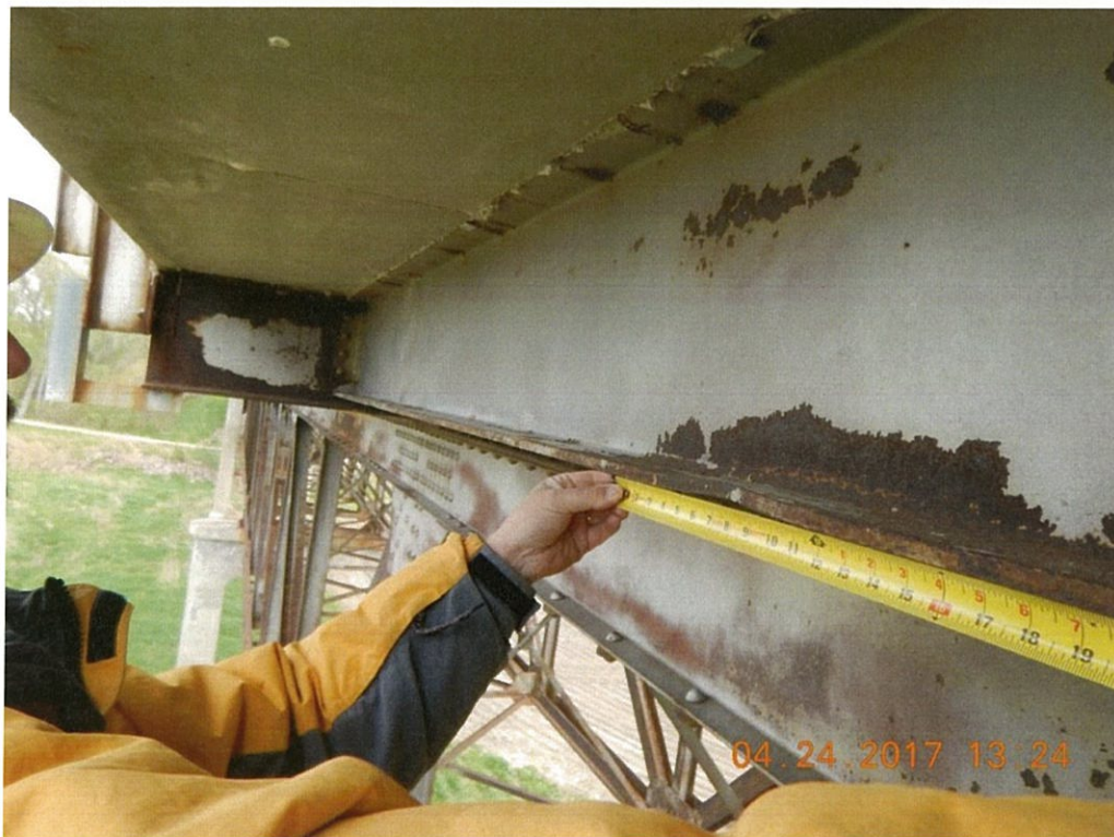
Photo 62: There are a few locations with minor bent flanges in the deck truss stringers. Span 7 Stringer 1 dent east of U3.
