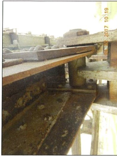
Span 4 L0 Lt bottom exterior packrust
