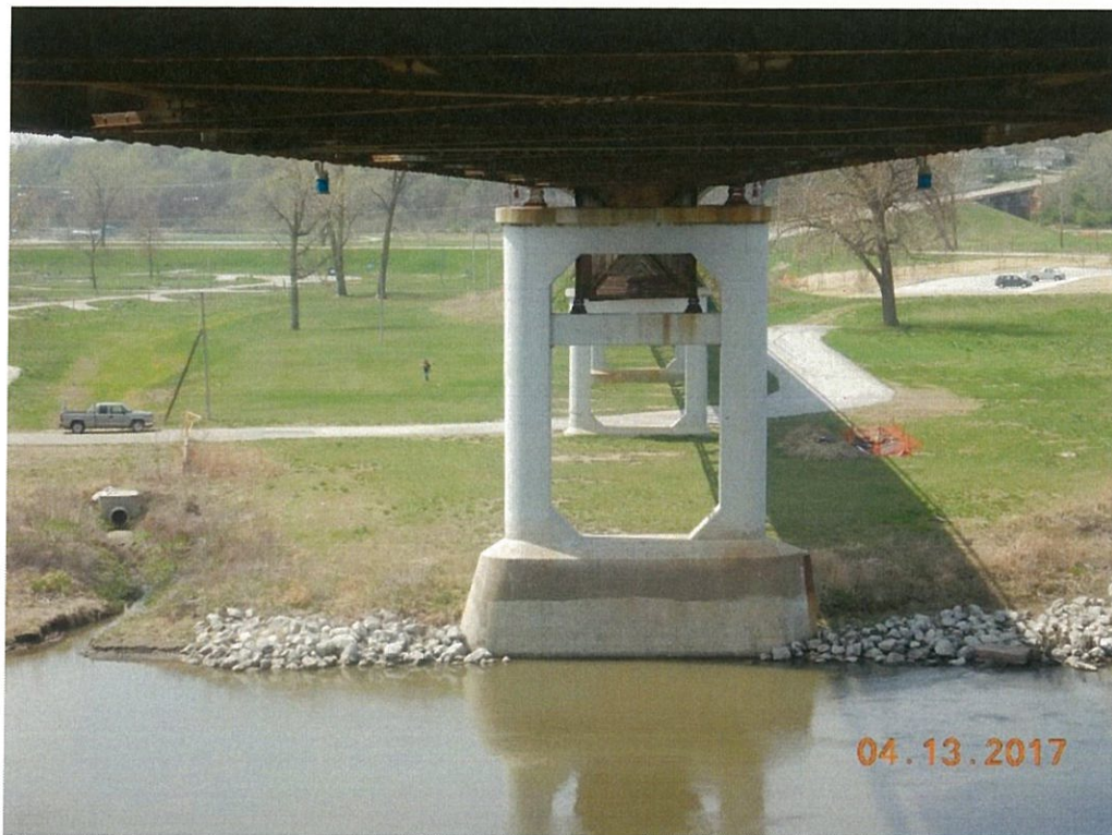
Photo 136: Riprap is sparse along the east face of Pier 4.
