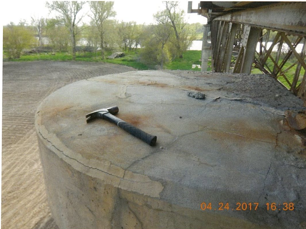
Photo 131: The concrete patch and south end of the Pier 8 cap by the south girder bearing is delaminating.
