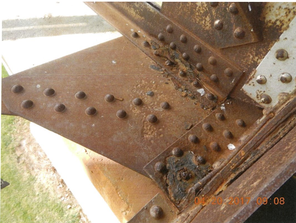
Photo 28: Section loss has occurred in several of the deck truss horizontal gusset plates from water previously sitting on the plates. Span 3 L0 Lt. shown.
