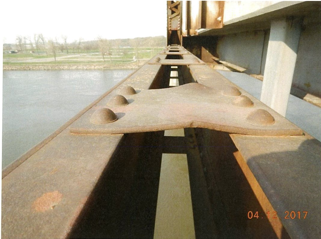
Photo 77: A few of the baton plates on the thru truss lower chords are slightly bent.
