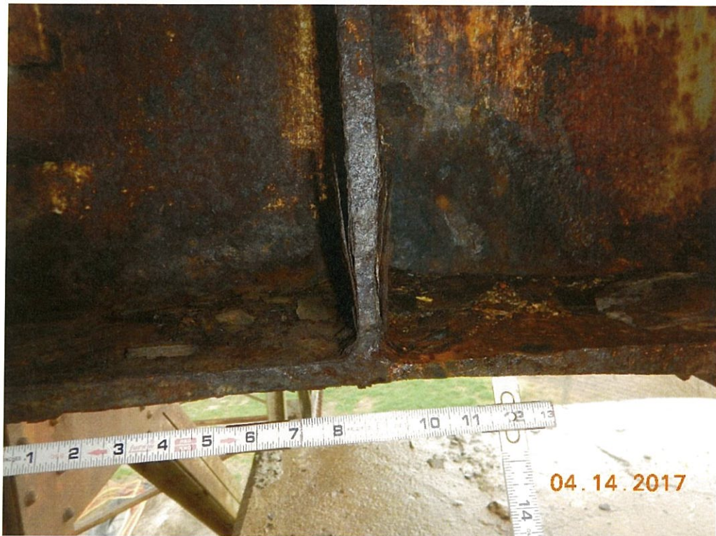
Photo 95: Thru truss floorbeam corrosion show at Span 6 Floorbeam L0' with section loss, below the joint.
