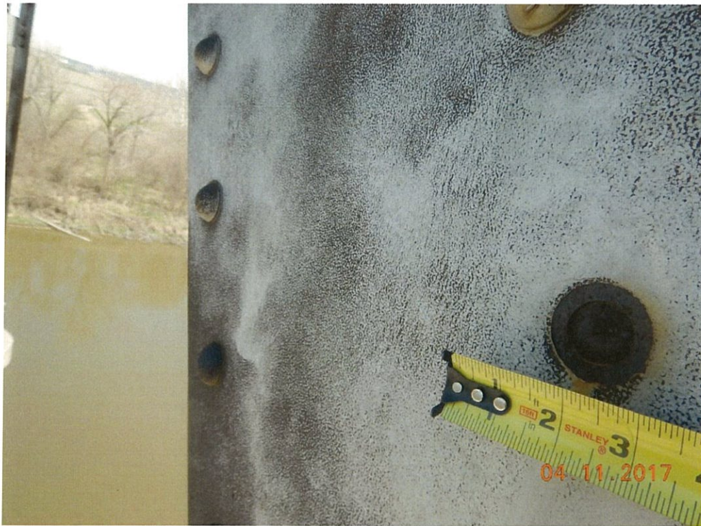
Photo 79: Span 6 U13L12 Rt. has 2 broken rivets on the interior face, only one shown.
