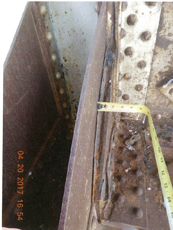
Photo 38: Heavier packrust up to 1" is typical at the deck truss gusset plates and plate connections to the bearings at the ends of the spans. Span 3 L0 Rt. interior top edge shown.
