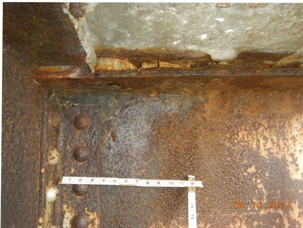
Photo 92: Typical thru truss floorbeam corrosion with packrust at stringers.
