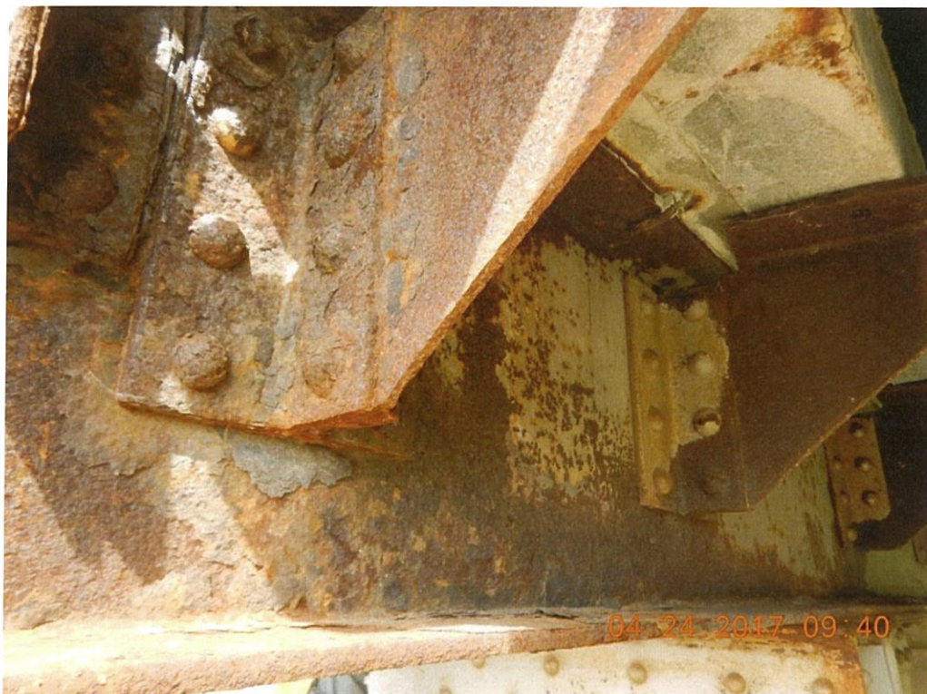
Photo 55: There are areas of delamination in the deck truss floorbeam faces below the deck joints. Span 7 Floorbeam 10 Rt. end shown.
