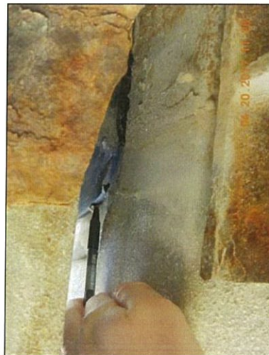
Pier 1 North deck joint torn
