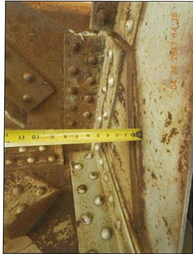
Span 7 L10 Lt top interior packrust
