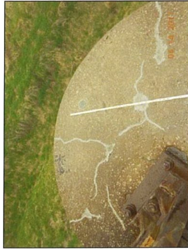
Pier 6 top cracking
