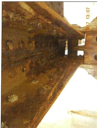
Span 4 L10 Lt bottom interior deterioration
