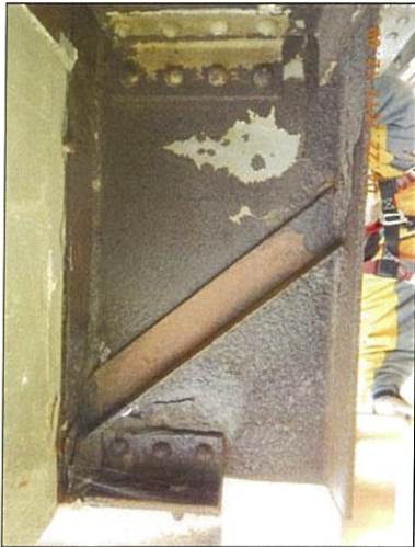
Span 4 Floorbeam 6 Lt stiffened and hole
