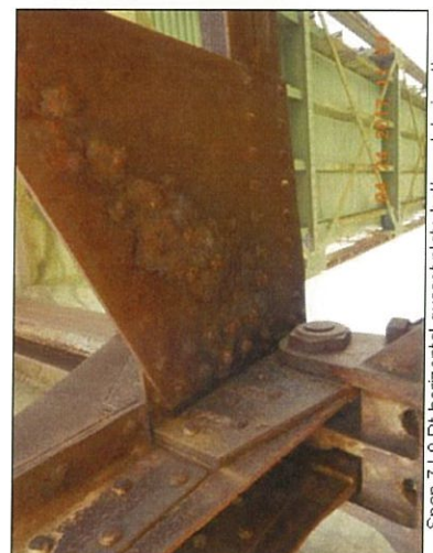
Span 7 L0 Rt horizontal gusset plate bottom deterioration
