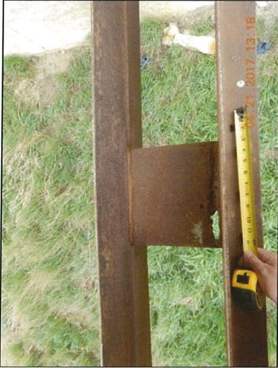
Span 1 L0L1 Lt exterior top angle hole at middle batten plate
