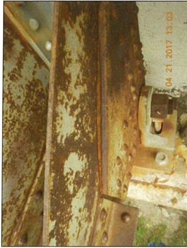
Span 1 L0 Lt top exterior packrust
