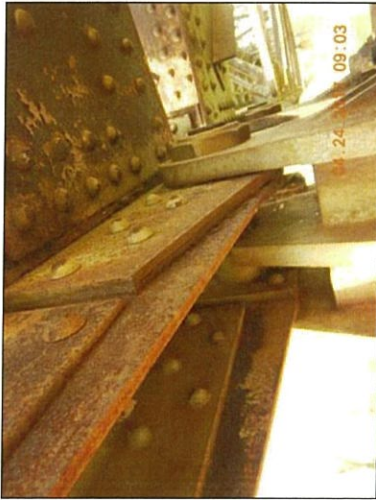
Span 8 L0 Rt bottom interior packrust
