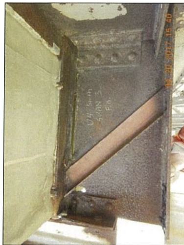
Span 3 Floorbeam 4 Rt stiffened and web deterioration...
