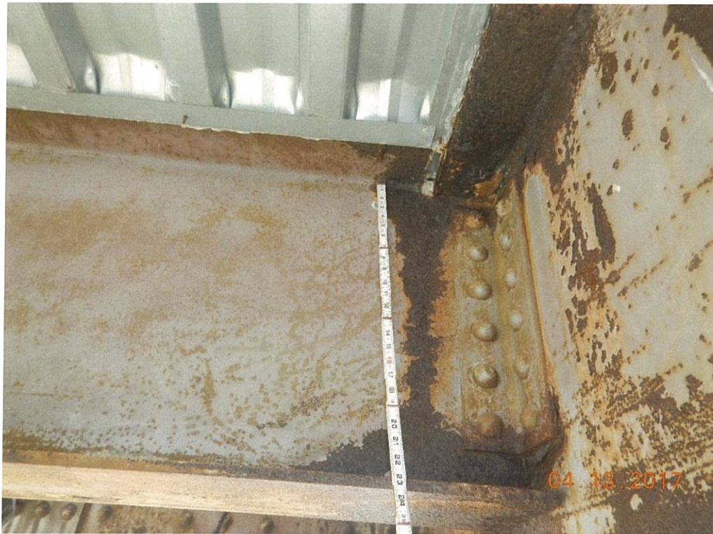
Photo 97: The thru truss stringers are in fair condition with corrosion typically occurring at their end support connections to floorbeams.
