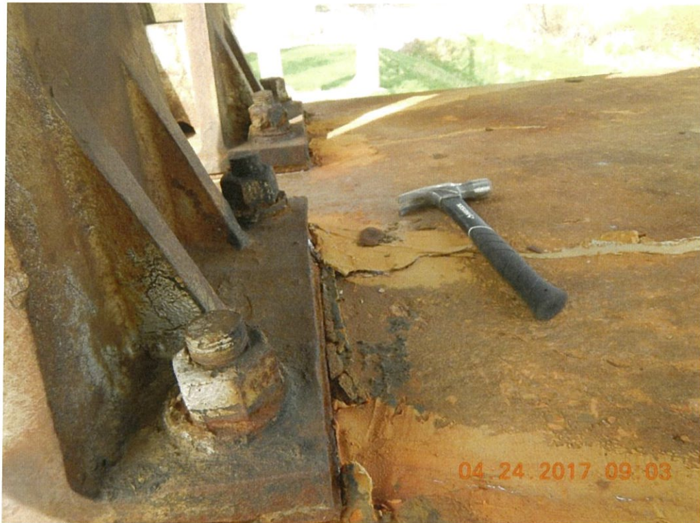
Photo 127: The patched concrete in Pier 7 around the Span 8 south bearing is delaminating.
