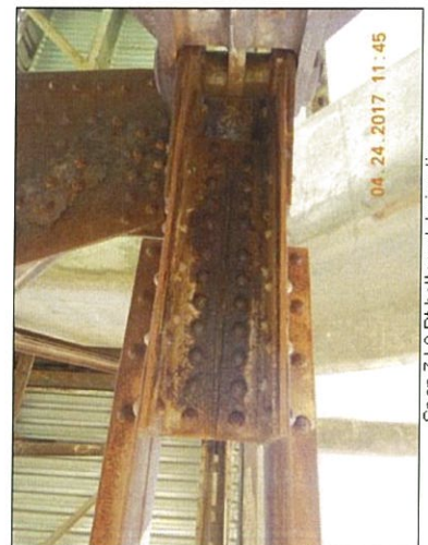
Span 7 L0 Rt bottom deterioration
