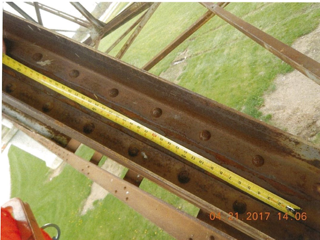
Photo 35: Minor packrust up to 1/4" is typical at the continuous plates of the deck truss diagonals consisting of four angles. Span 1 U6L5 Lt. shown.
