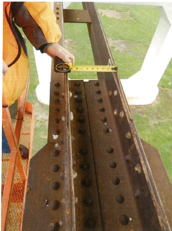
Photo 32: Minor packrust up to 1/4" is typical at the deck truss lower chord splices. Span 2 L8L9 Lt. shown – note this splice has more packrust than typical.
