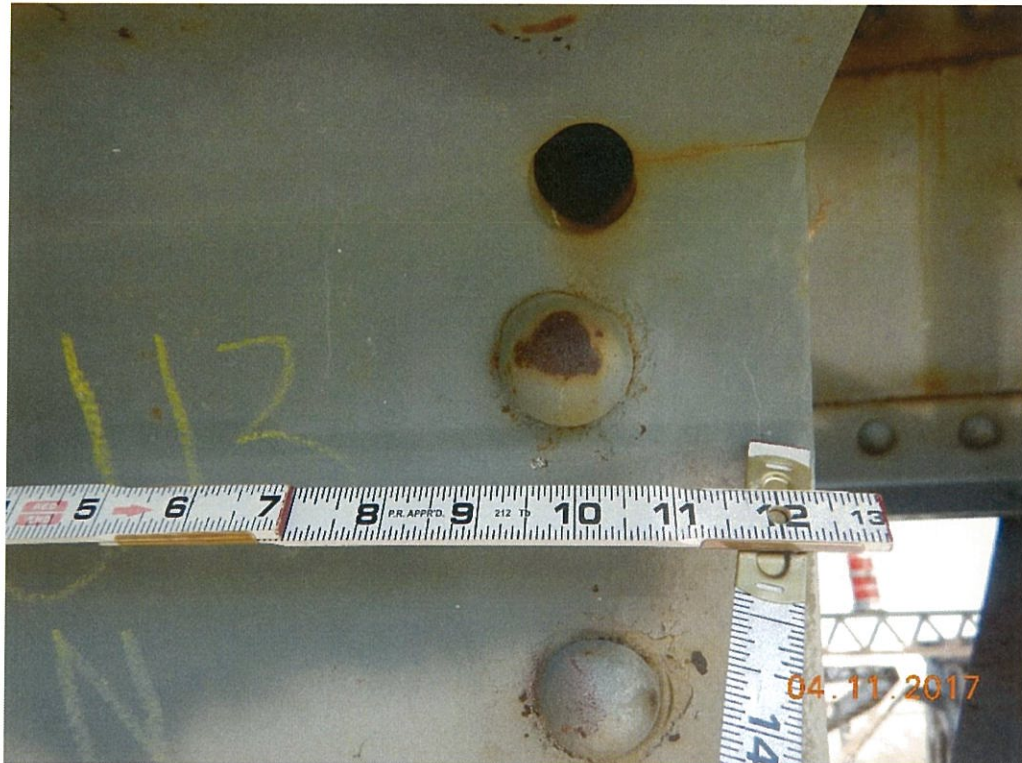
Photo 81: There is a crack with a previously installed arrest hole located in the sway bracing gusset plate at Span 5 U13 Lt.; the crack has not propagated beyond the hole.
