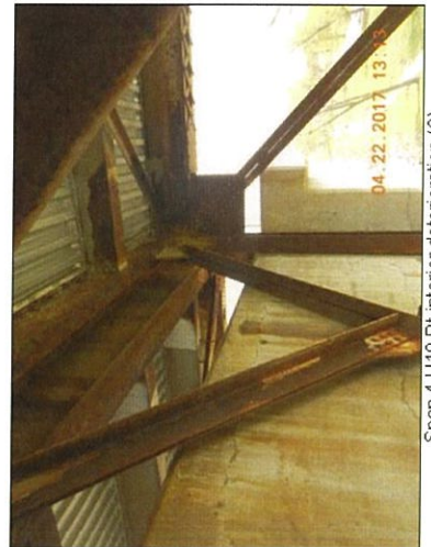
Span 4 U10 Rt interior deterioration (2)
