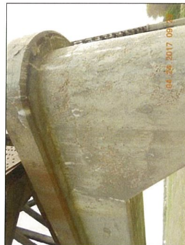
Pier 7 South end west face deterioration
