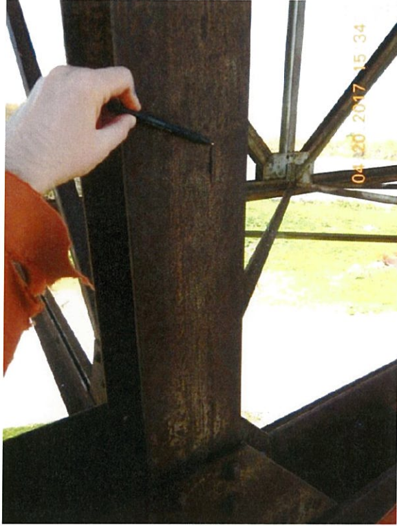
Photo 51: The exterior face of Span 3 U4L4 Rt. has a small rolling defect above L4.
