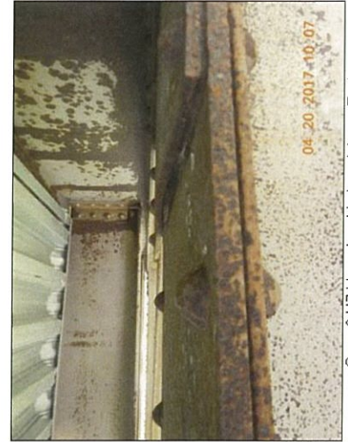
Span 2 U7 Lt packrust in top plate on East
