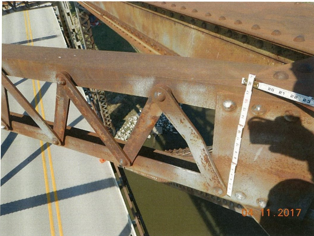
Photo 80: A few of the thru truss upper lateral bracing lattice bars of are slightly bent at random areas throughout.
