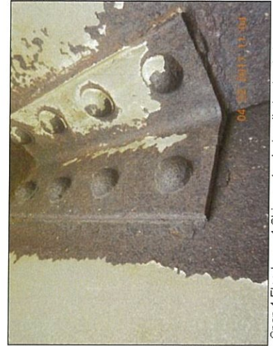
Span 4 Floorbeam 4 Stringer 1 exterior clip bent out at corner
