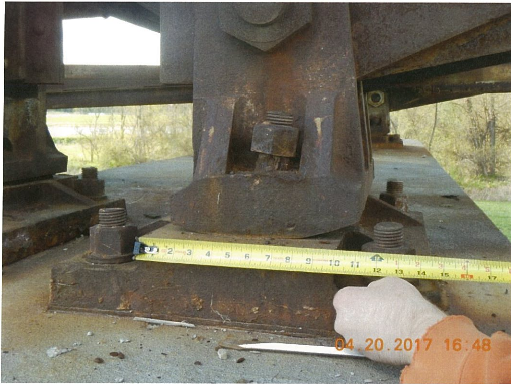
Photo 105: The Span 3 bearings at Pier 2 are no longer centered on the bearing plate and have slide in towards the span approximately \frac{3}{4} ". L0 Rt. shown.
