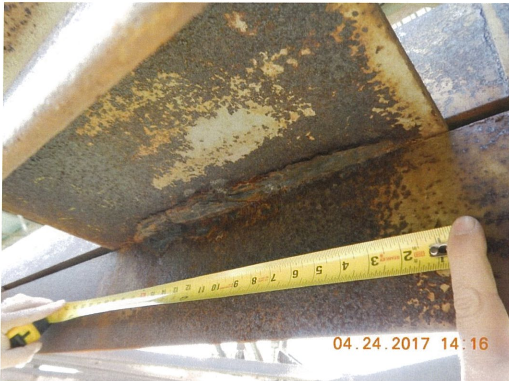
Photo 21: The section loss at the batten plates of the deck truss lower chords is typically on the inside of the lower chord angle above and below the batten plate. Span 7 L0L10 Lt. shown.
