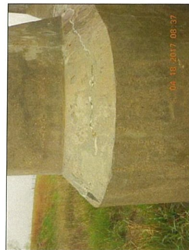
Pier 8 deterioration on Northwest
