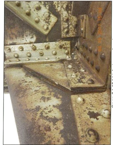
Span 3 L10 Lt interior packrust
