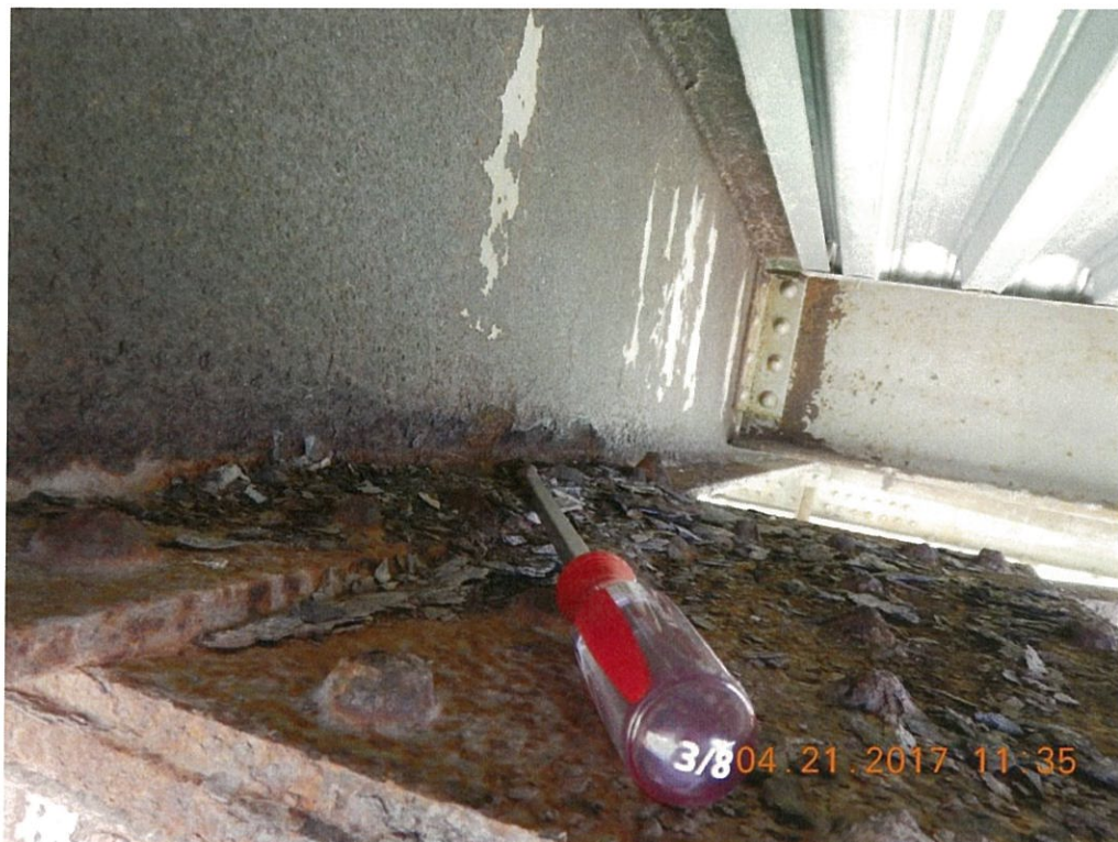
Photo 53: The deck truss floorbeams have minor surface rust throughout; heavier rust typically at the floorbeam ends overhanging the truss. Span 1 Floorbeam 2 Rt. shown.
