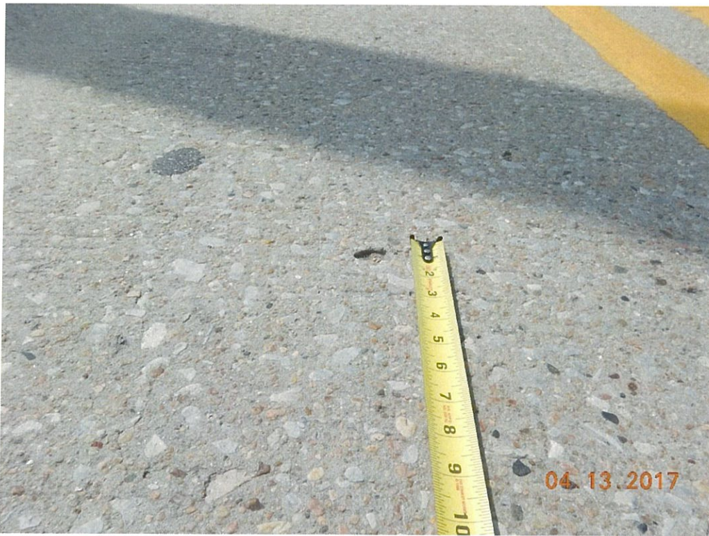
Photo 5: There are several small aggregate popouts, ¼" to 1", scattered throughout the deck surface.
