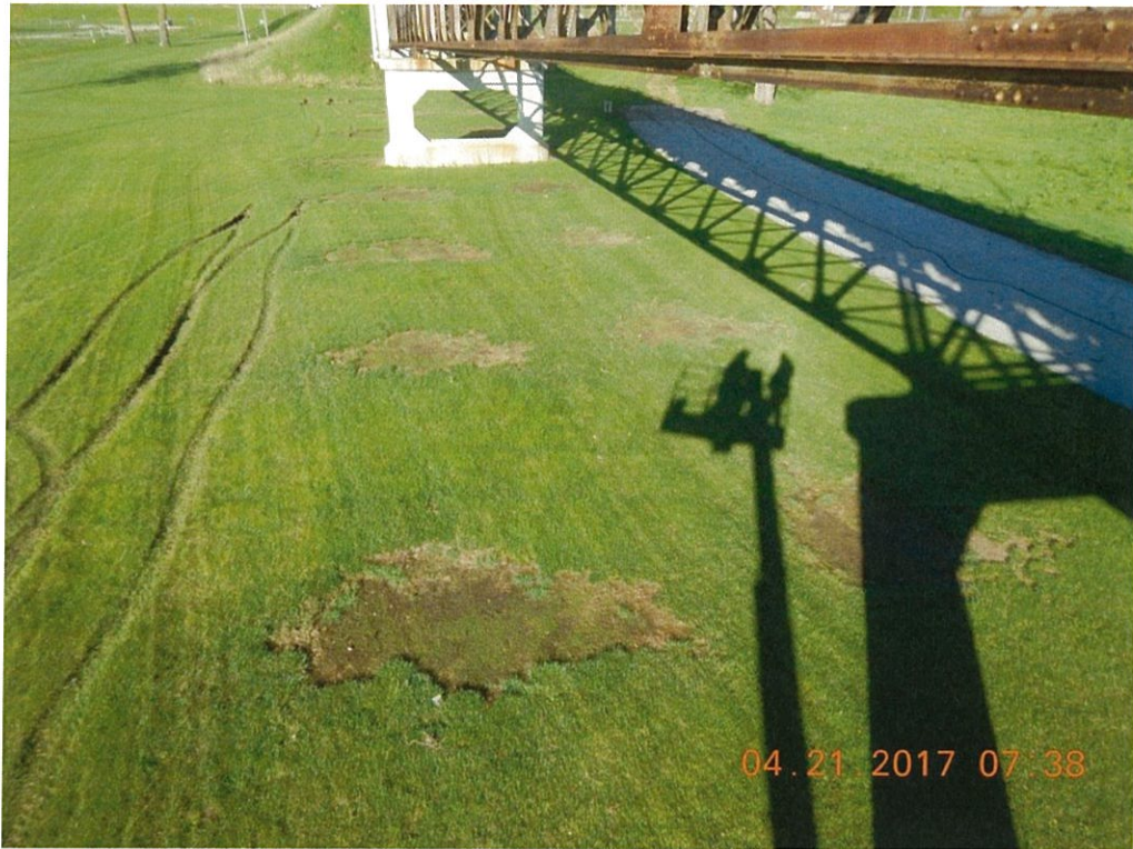
Photo 135: There is erosion of the grass and soil below the deck drains of Spans 1 through 4.
