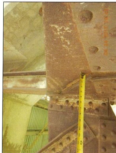
Span 7 L0 Lt top interior packrust
