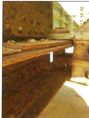
Span 8 L10 Lt bottom interior packrust
