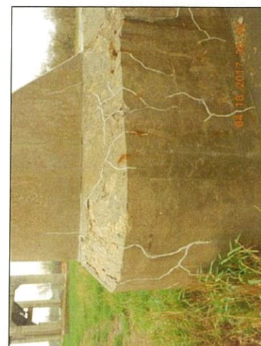
Pier 8 South cracking and scaling
