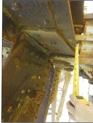
Span 2 bottom interior packrust
