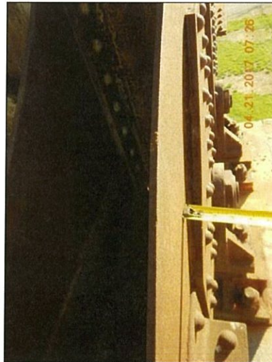
Span 3 L10 Rt top exterior packrust (2)
