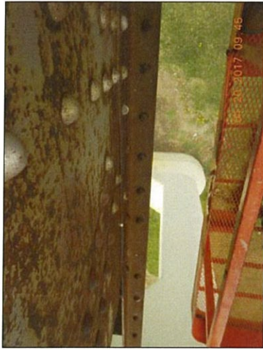
Span 2 L9 Lt exterior packrust at top of lower chords
