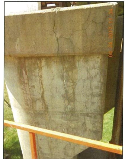
Pier 6 South end top deterioration on west face
