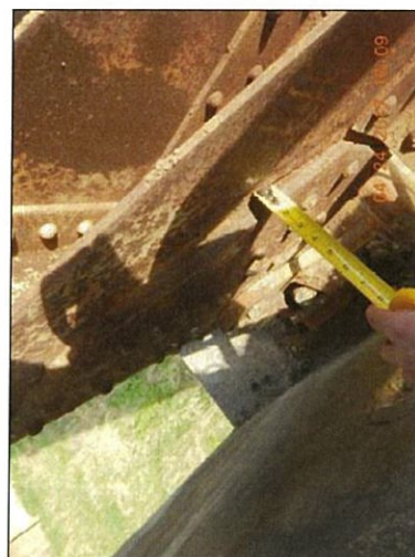
Span 8 L10 Lt top exterior packrust
