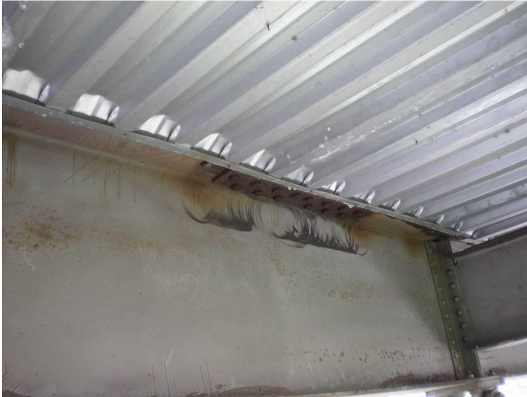
Photograph 29 – Repair Plate on Beam Top Flange
