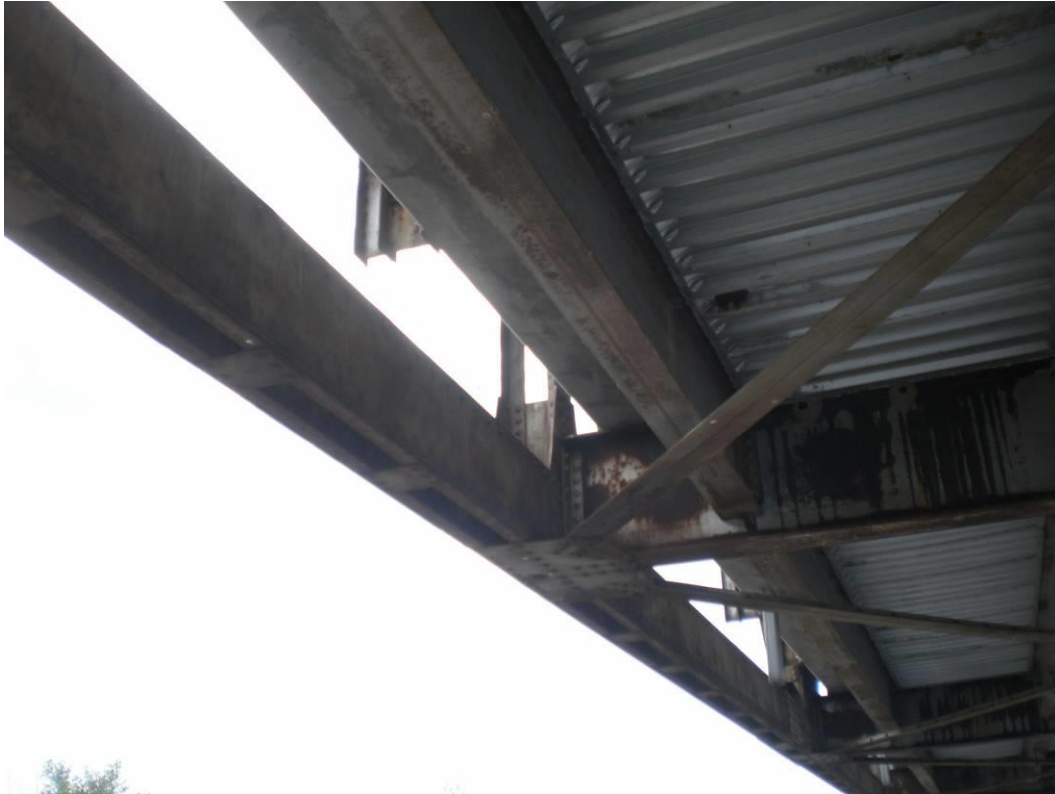
Photograph 44 – Typical Corrosion at Floorbeam Extension to Truss Vertical Connection
