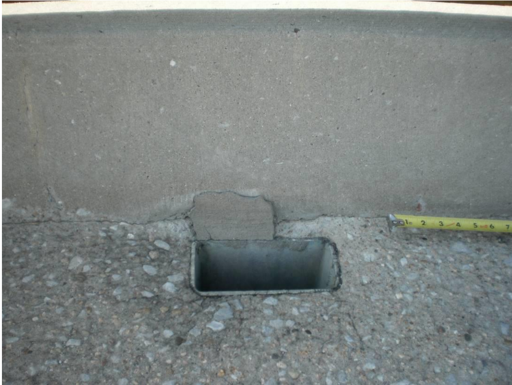
Photograph 81 – Chipped Area and Exposed Aggregate at a Deck Drain
