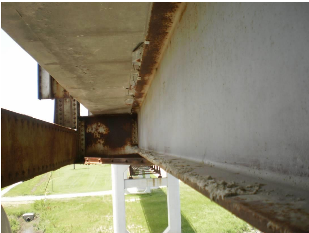
Photograph 45 – Corrosion on Floorbeam Extension and Bottom Chord
