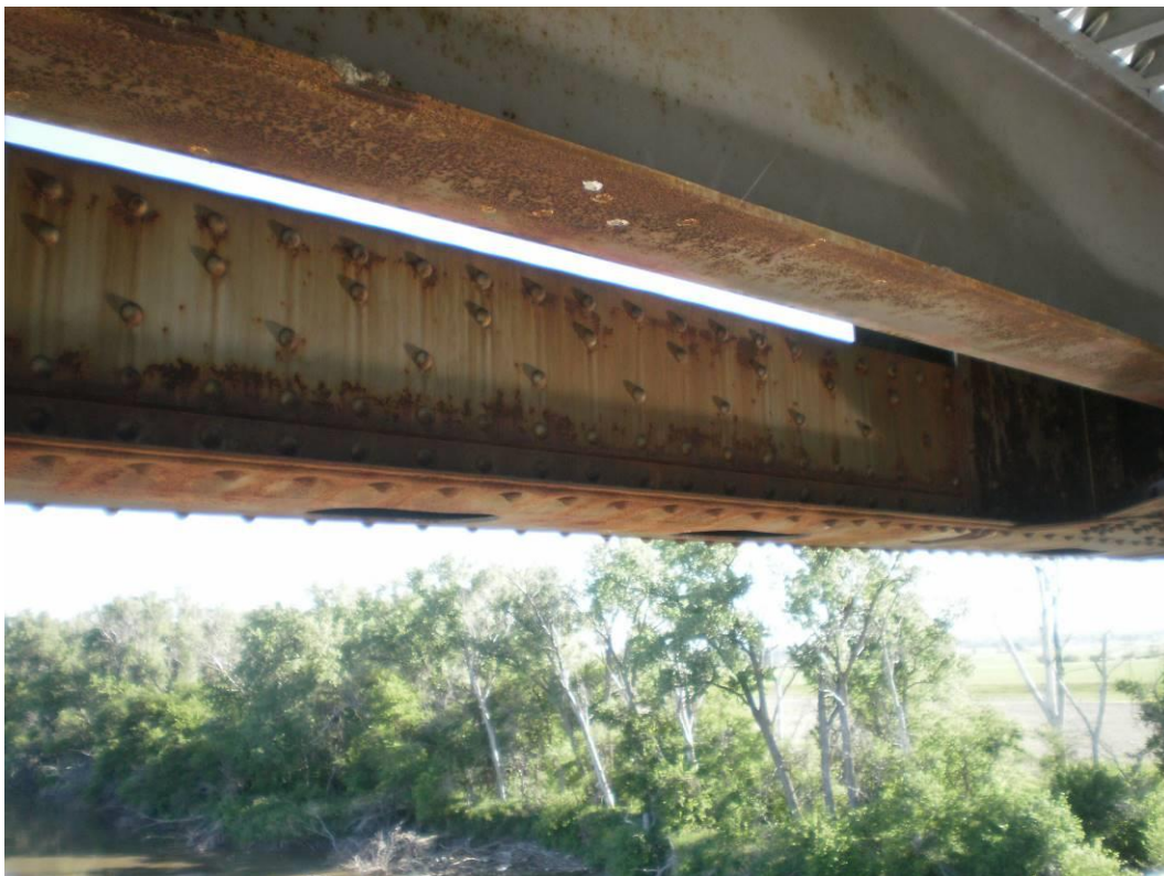
Photograph 49 – Distended Bottom Chord Cover Plate
