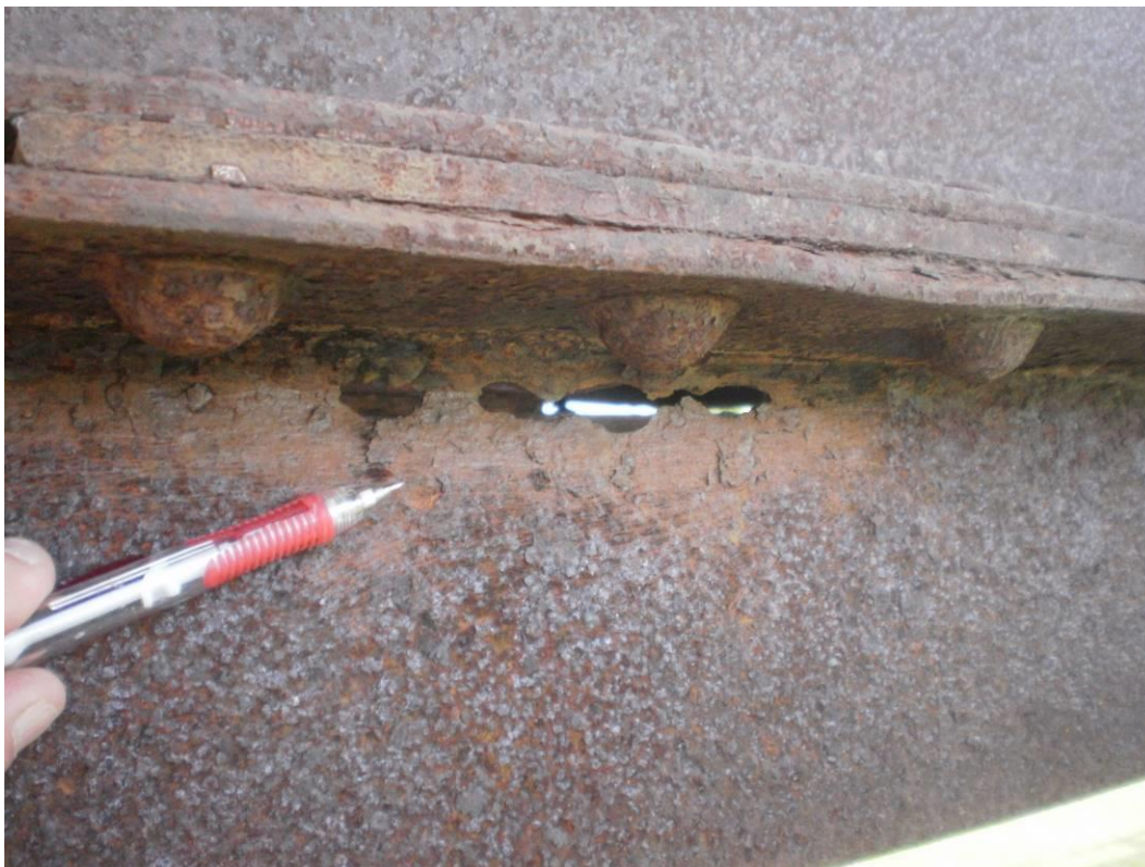
Photograph 10 – Corrosion Perforation in Bottom Chord in Span 1 – Note No Paint Remaining
