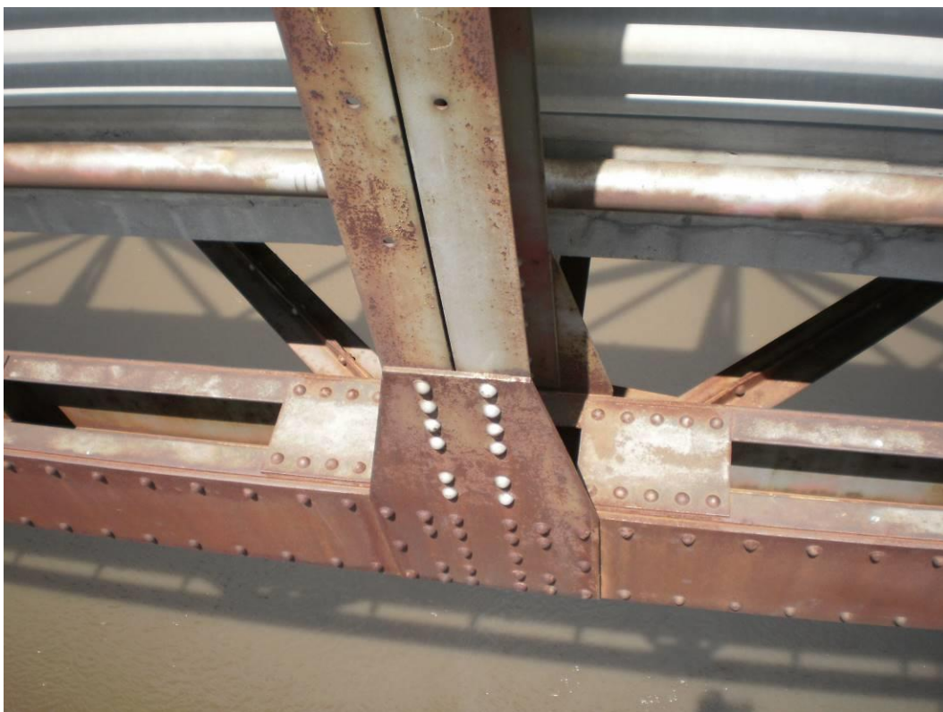
Photograph 39 – Areas on Truss Bottom Chord with Little Paint Remaining
