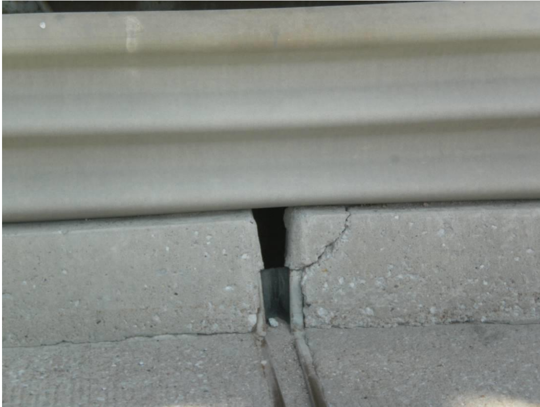
Photograph 85 – Cracked Curb at Strip Seal Joint Extrusion at Pier 5
