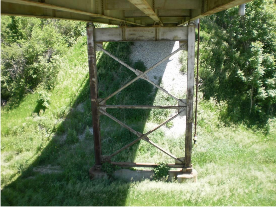
Photograph 27 – Typical Coating Condition of the Steel Bents
