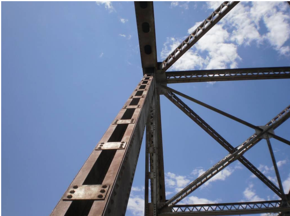
Photograph 35 – Slightly Better Coating Condition above the Splash Zone
