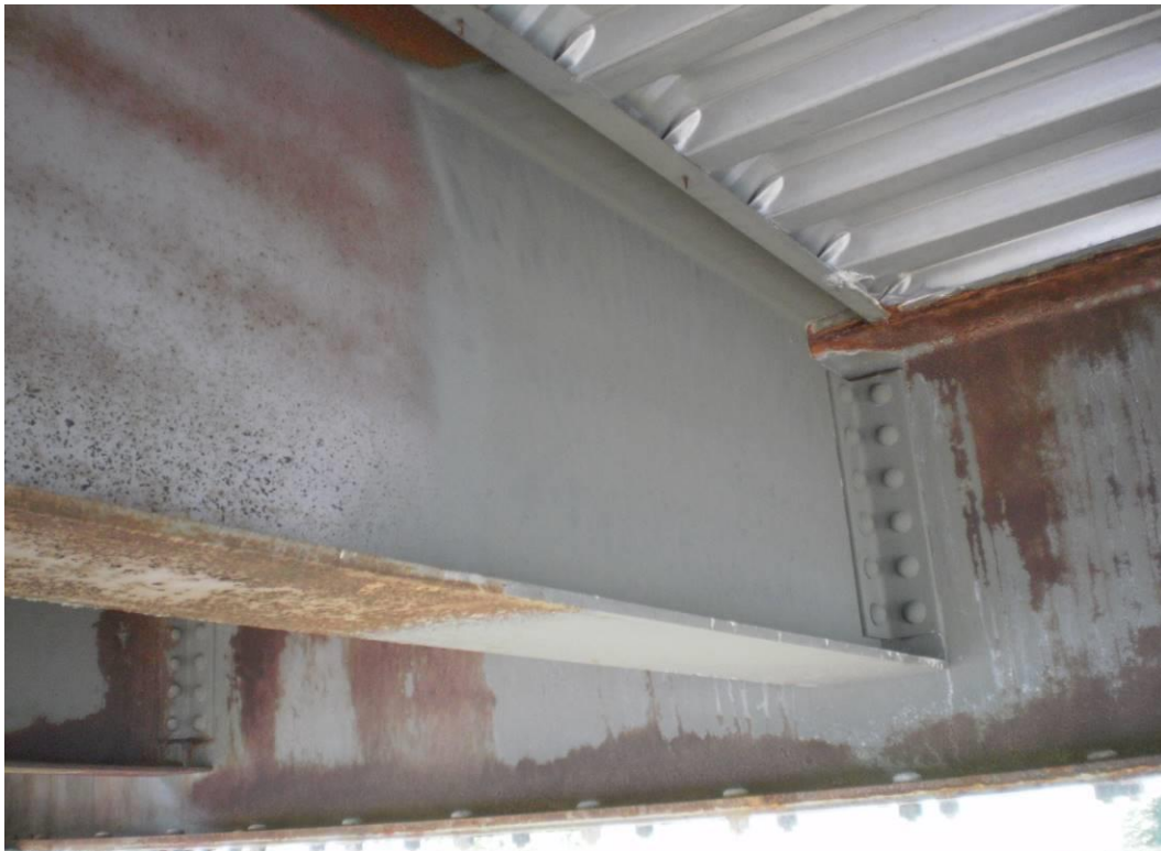
Photograph 55 – Touch-up Area on Stringer End – Note Adjacent Stringer Not Touched-up
