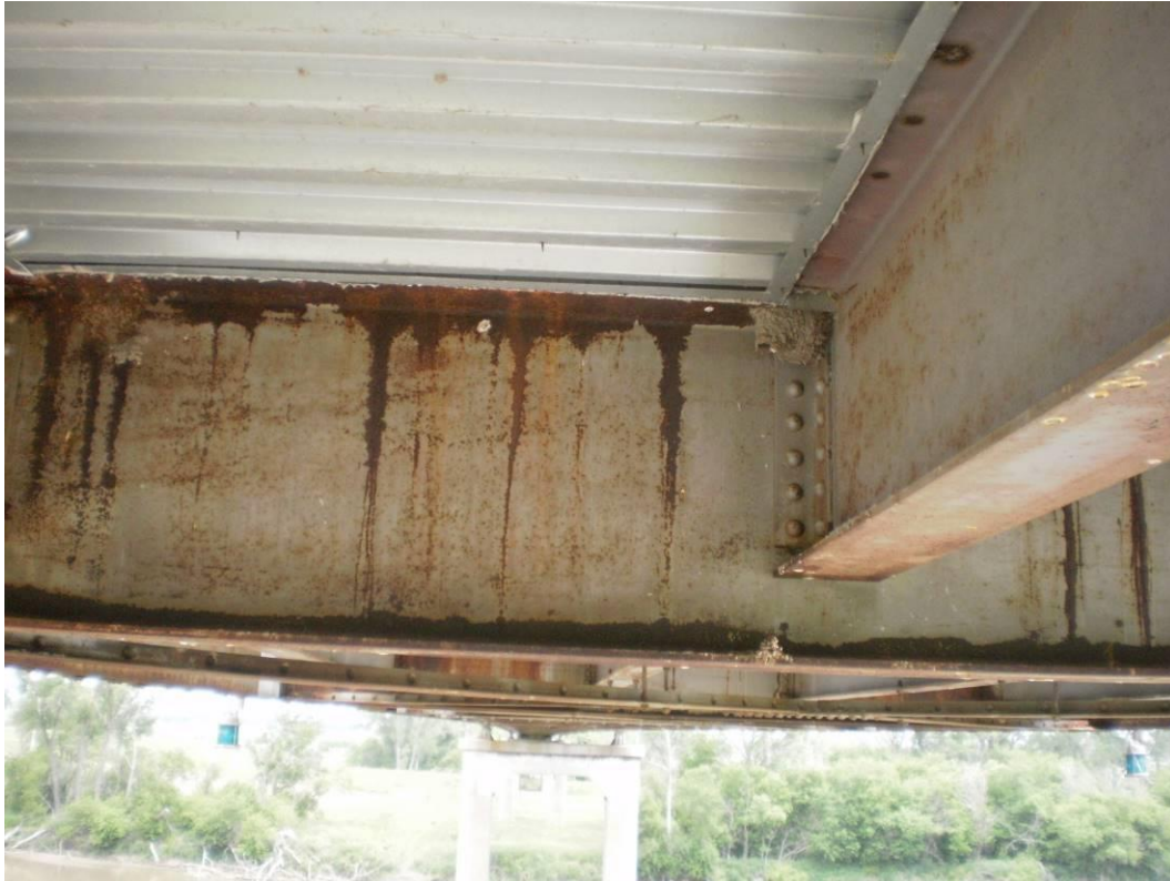
Photograph 42 – Typical Areas of Spot and Pinpoint Corrosion on Stringers and Floorbeams
