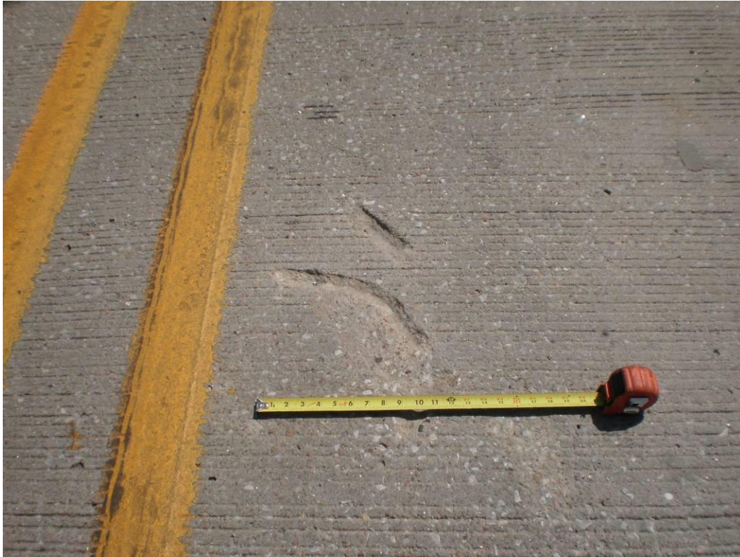
Photograph 87 – Mechanical Damage to Deck – Span 6, Downstream Lane, 4 Panels from Iowa Portal
