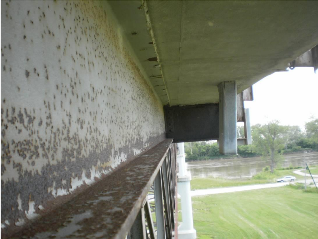
Photograph 12 – Coating Failure and Rust on the Outside Face of the Exterior Stringers
