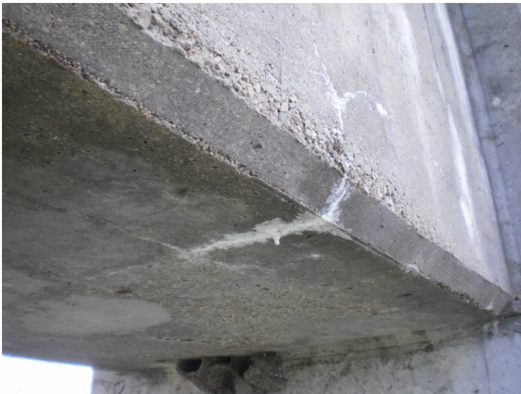
Photograph 71 – Cracks exuding Efflorescence
