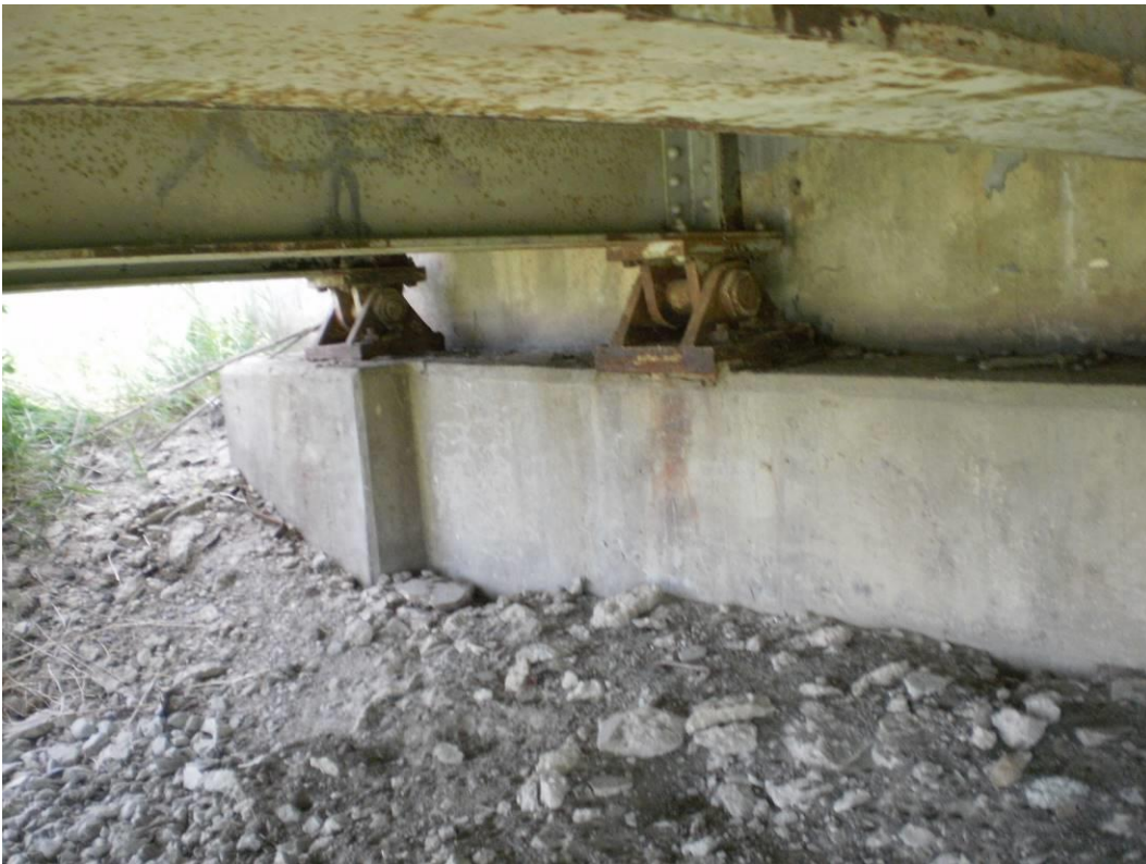
Photograph 74 – Good Condition of Concrete at Abutment No. 2
