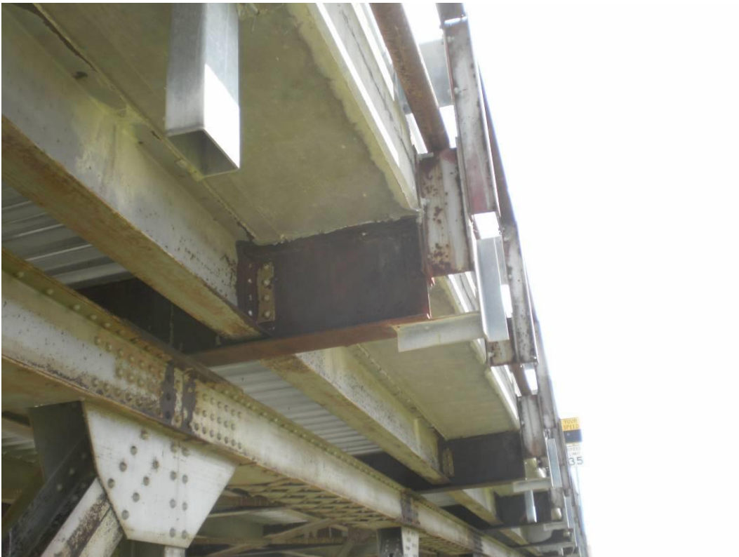
Photograph 13 – Rust on Floorbeams and Floorbeam Ends
