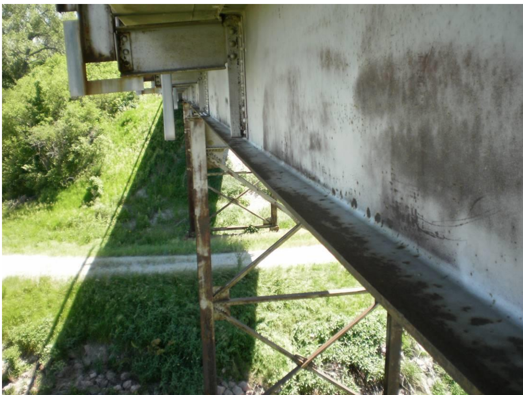
Photograph 26 – Coating Wear on Beam Web and Bottom Flange
