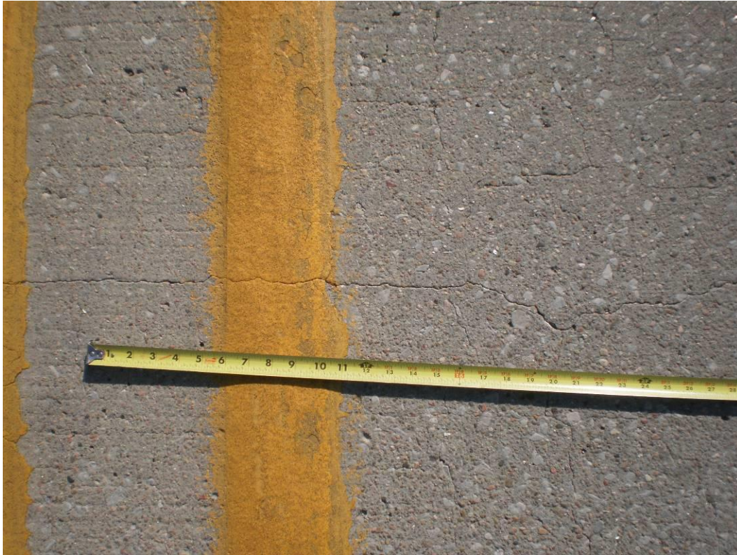
Photograph 83 – Transverse Crack at the Centerline of the Bridge
