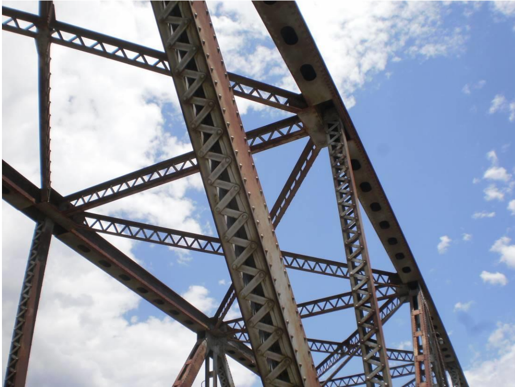
Photograph 40 – Areas of Exposed Primer on Outside Face of Truss Members
