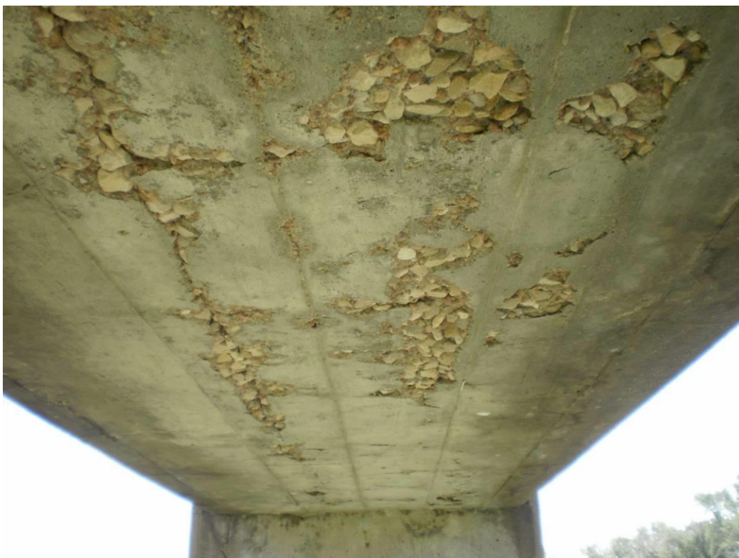
Photograph 72 – Exposed Aggregate at the Underside of the Pier Cap at Pier 7
