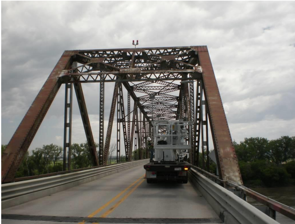
Photograph 34 – Typical Coating Condition at Truss Portals
