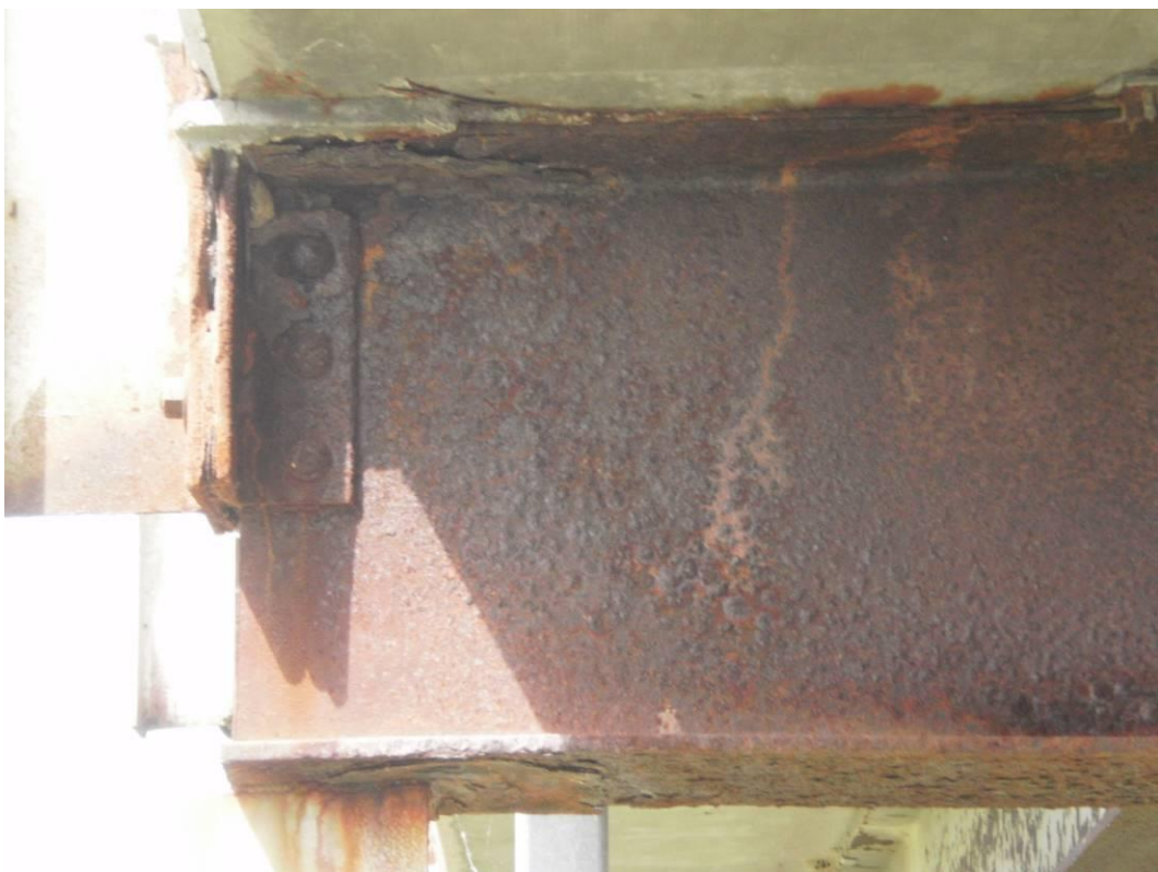
Photograph 17 – Section Loss at Floorbeam Ends
