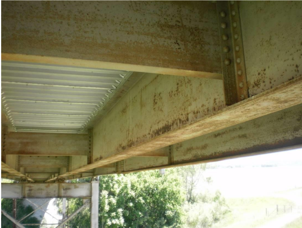
Photograph 21 – Typical Condition of the Interior Beams and Diaphragms
