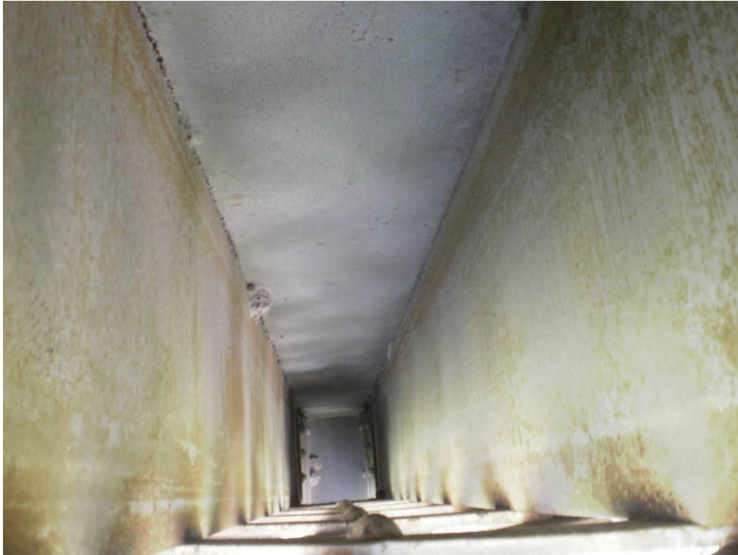
Photograph 6 – Pinpoint Rusting on the Interior Surface of the Top Chord
