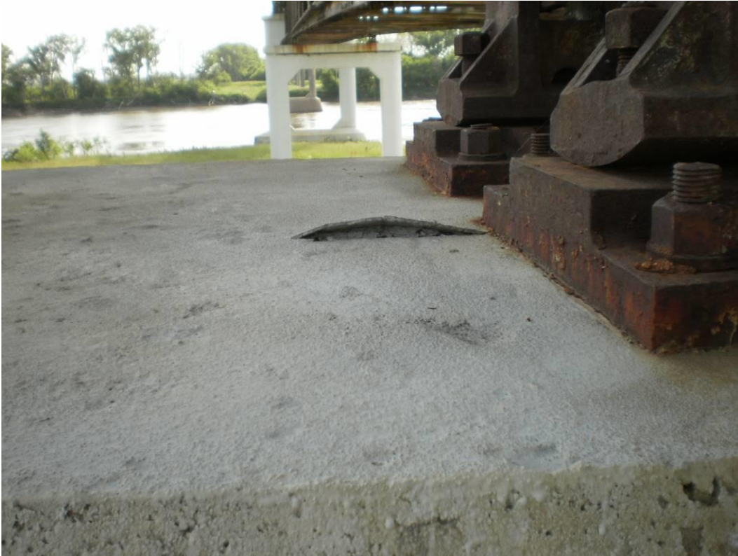
Photograph 65 – Area of Lifting Coating on a Pier Cap
