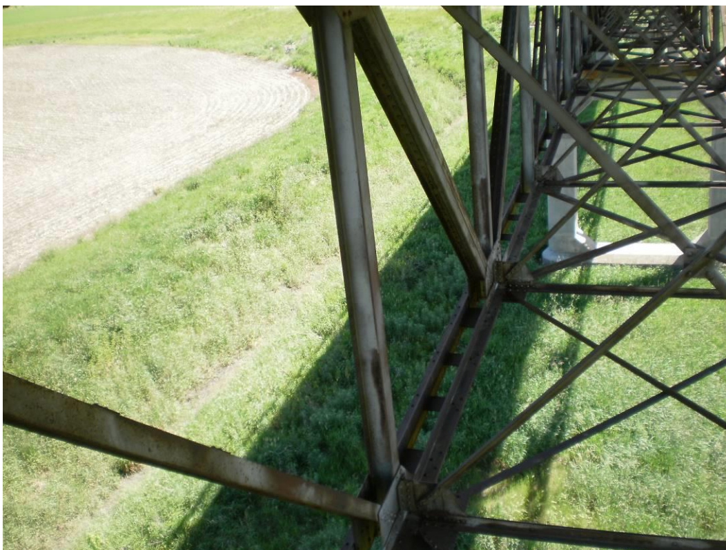
Photograph 20 – Areas where the Paint is Worn Thin or No Paint Remains
