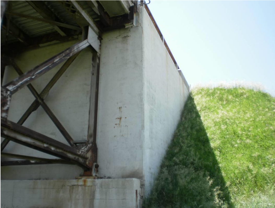
Photograph 75 – Good Condition of Abutment No. 1 Backwall
