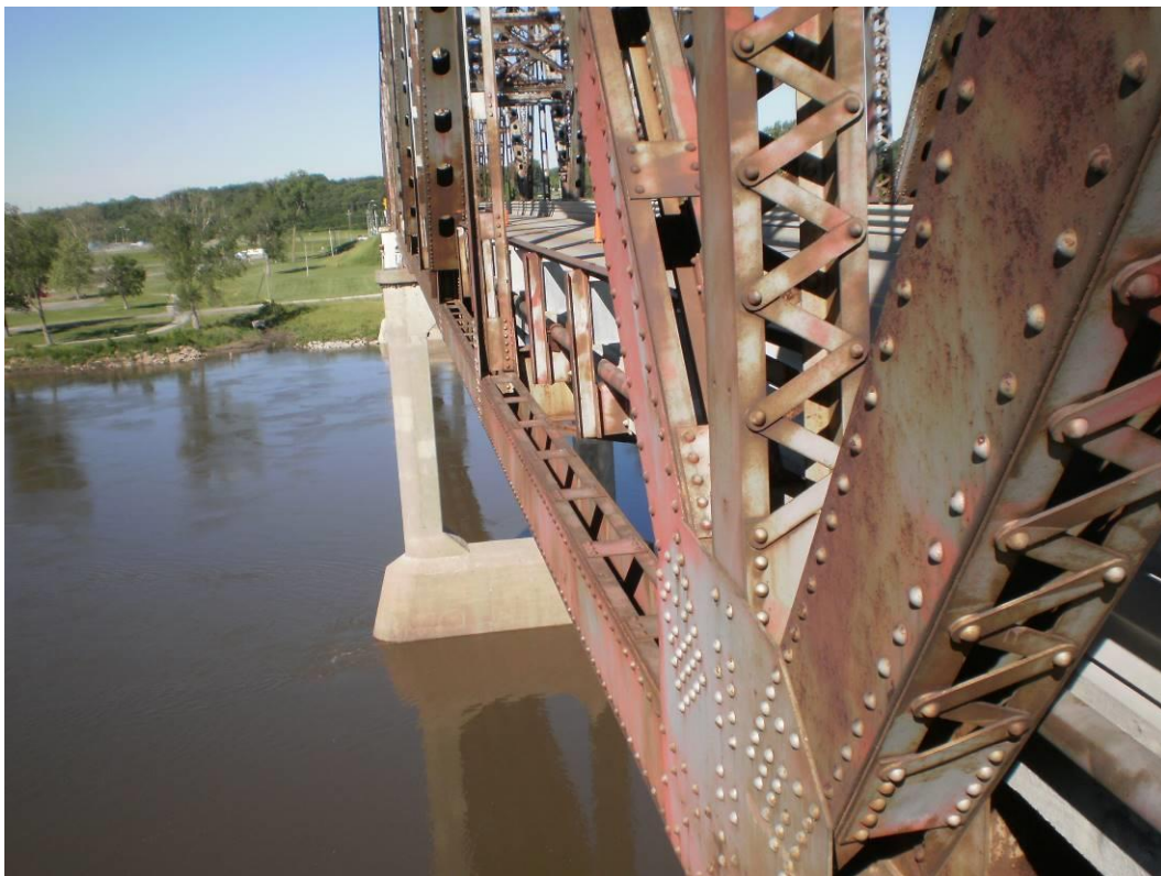
Photograph 41 – Exposed Primer on Truss Members
