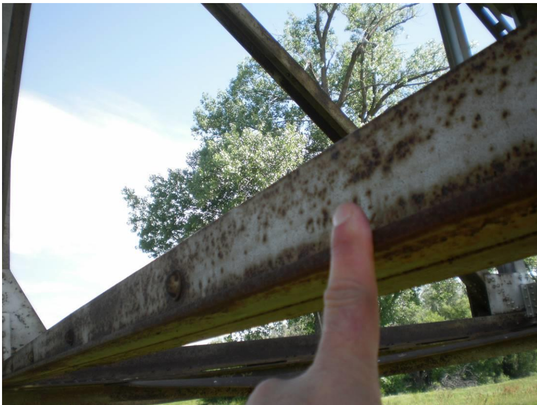
Photograph 9 – Edge Corrosion and Pinpoint Rust on Sway Frame Struts
