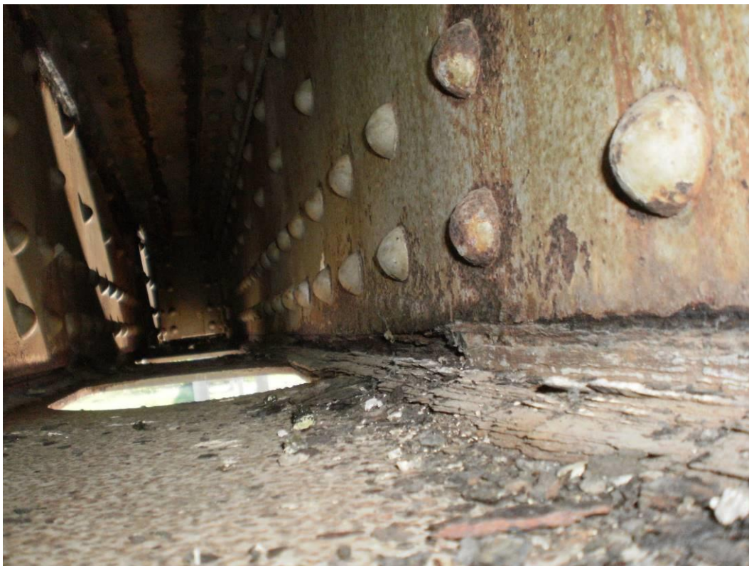
Photograph 52 – Section Loss along Web of Truss Bottom Chord
