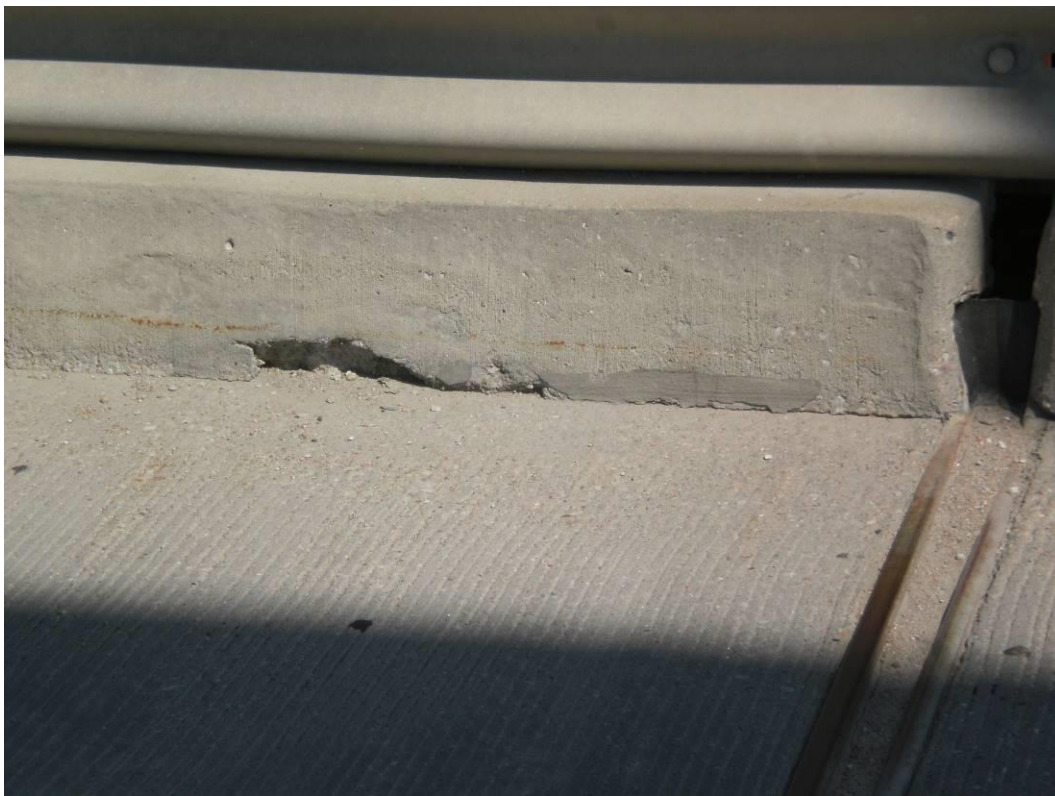
Photograph 86 – Chipped Area of Curb in Span 5 Near Midspan, Upstream Side of Bridge
