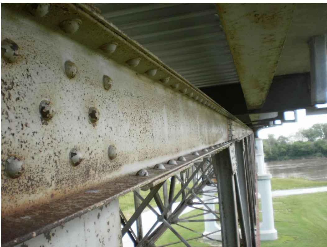
Photograph 11 – Typical Condition of Outside Face of the Top Chord
