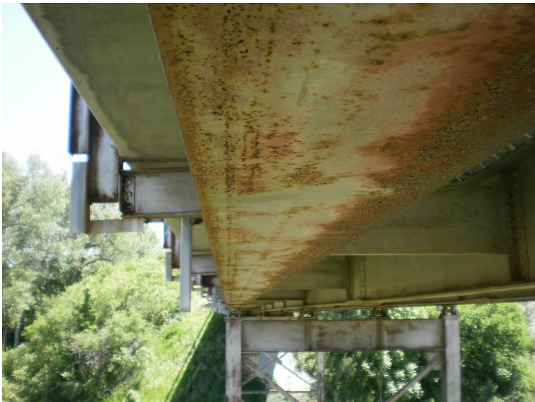
Photograph 22 – Edge Rusting and Small Spot Corrosion on the Exterior Beam Bottom Flange
