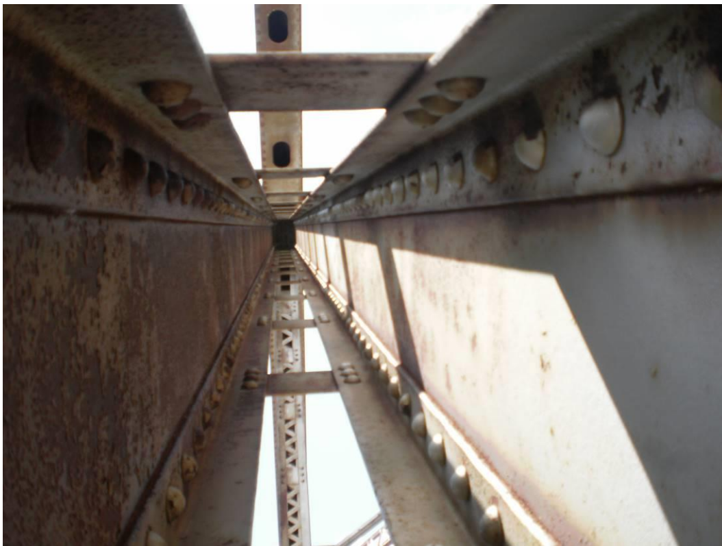
Photograph 36 – Typical Coating Failure and Rust on the Interior of Box Members
