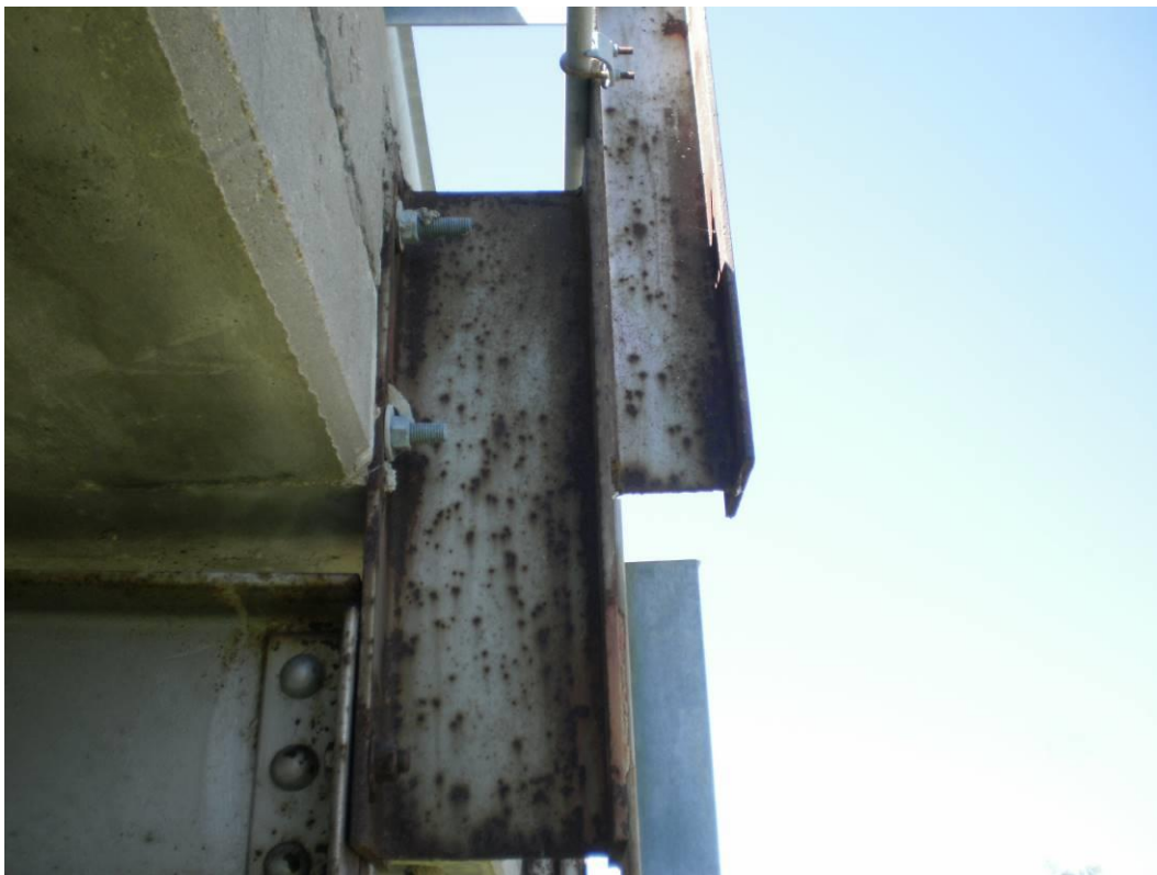
Photograph 25 – Corrosion on the Guardrail Posts
