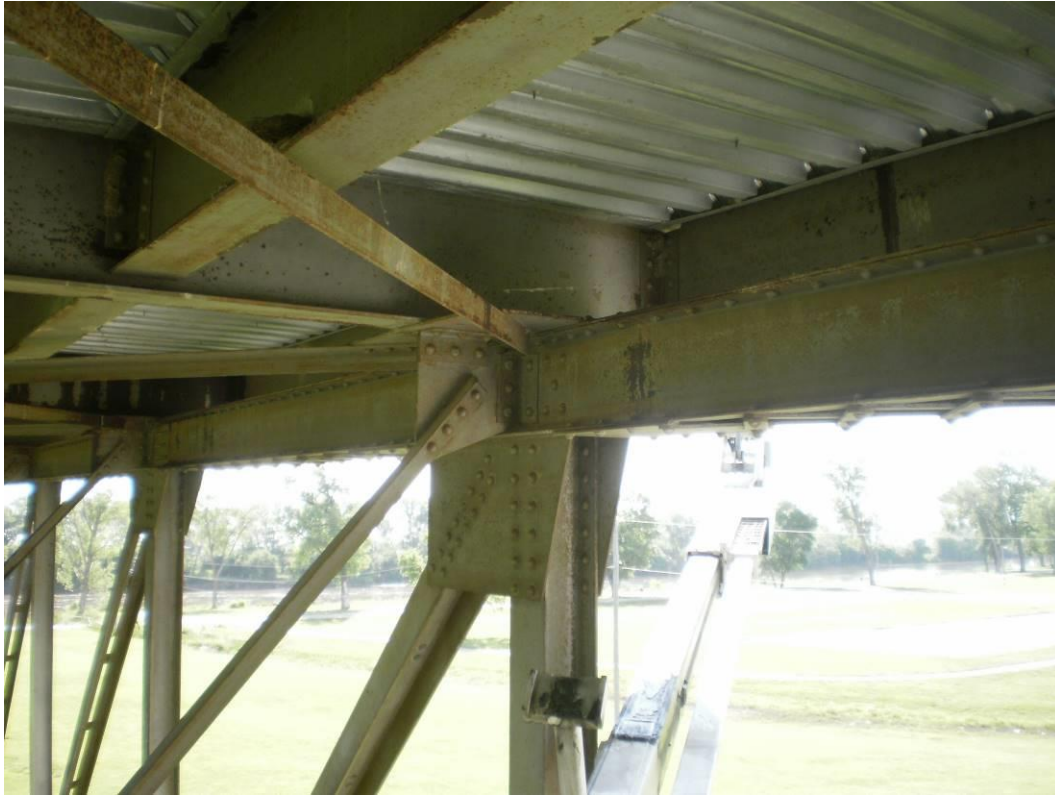
Photograph 4 – Typical Coating Condition of Inside Face of the Top Chord
