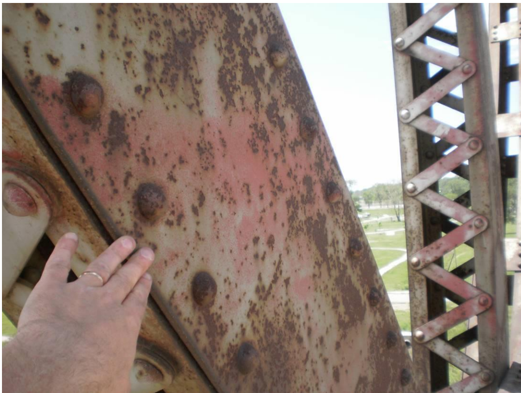
Photograph 38 – Areas of Corrosion and Exposed Primer on Truss Members
