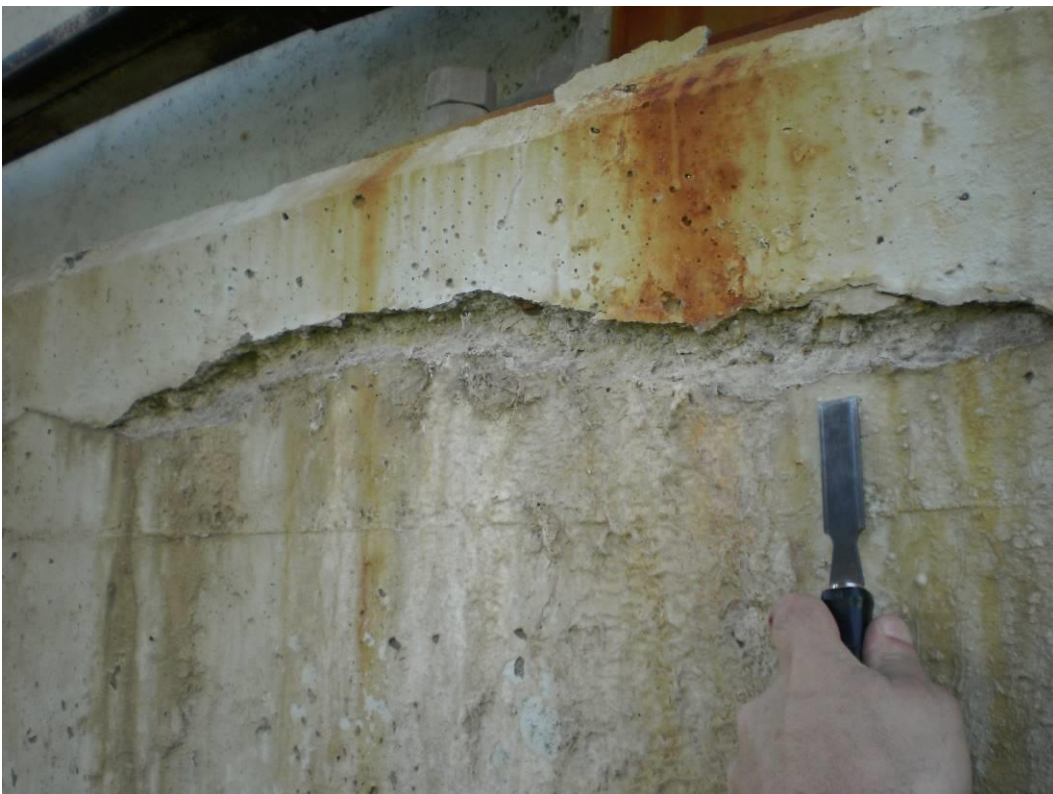
Photograph 76 – Crack and Chipped/Spalled Area on Abutment No. 1 Pedestal
