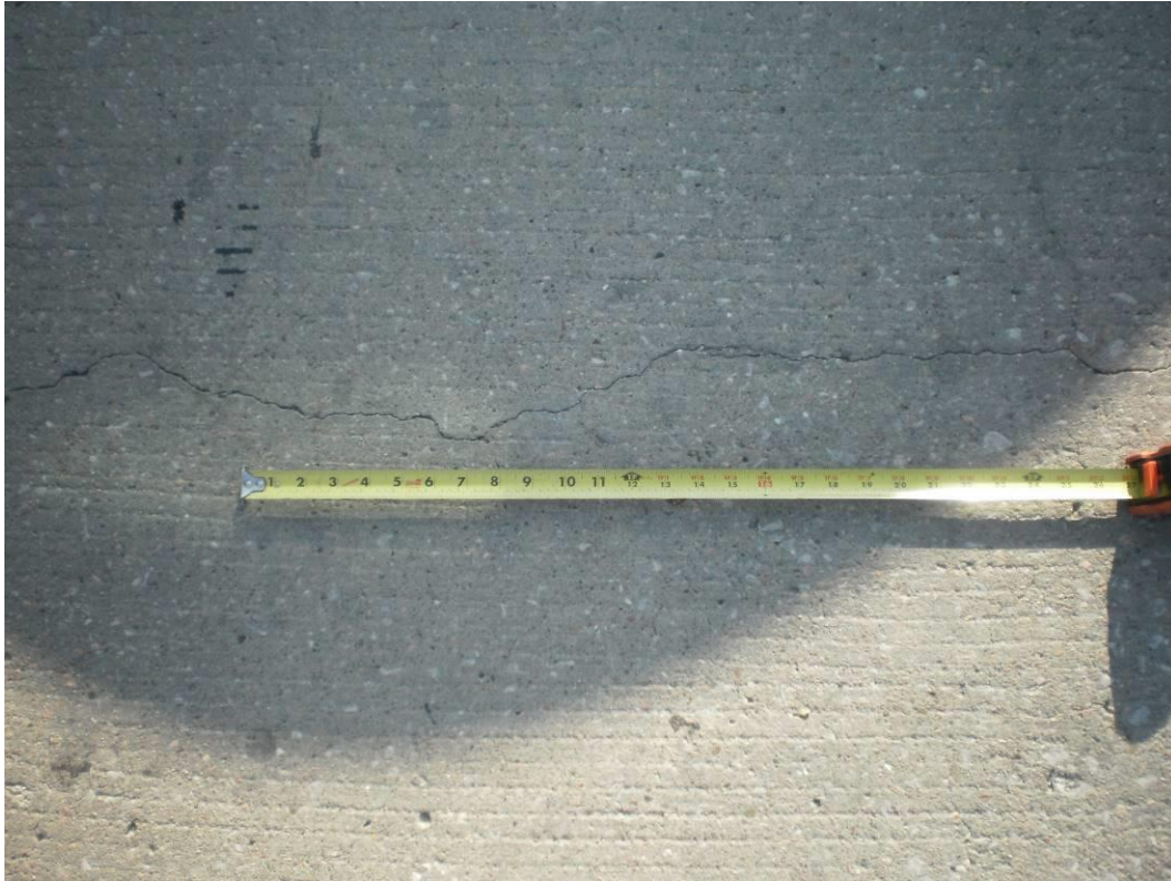
Photograph 79 – Typical Transverse Crack in the Bridge Deck
