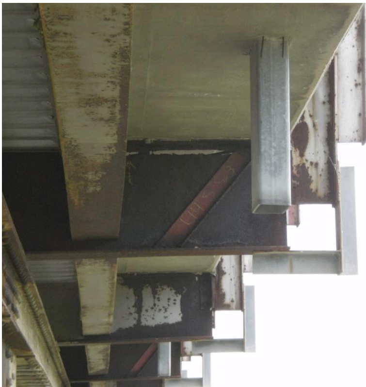
Photograph 16 – Floorbeam End with Perforation and Strengthening Channel
