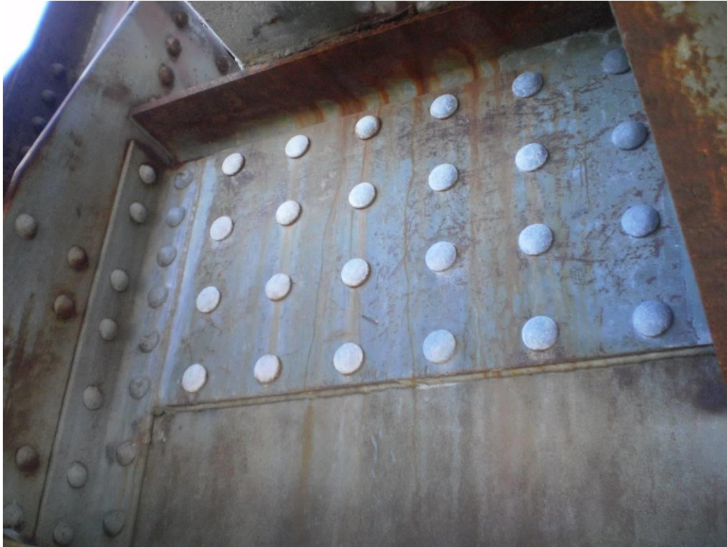
Photograph 58 – Strengthening Plate added at Floorbeam to Truss Connection
