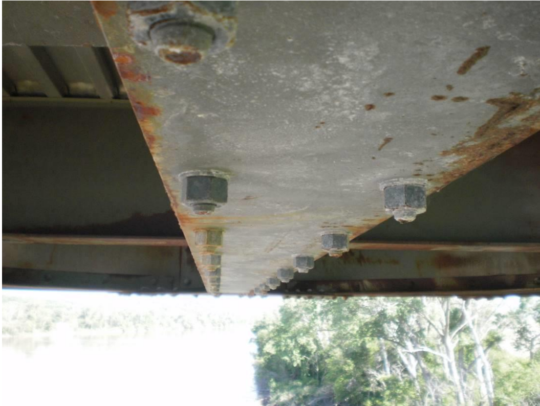
Photograph 56 – Newer Floorbeam Bottom Flange Cover Plate
