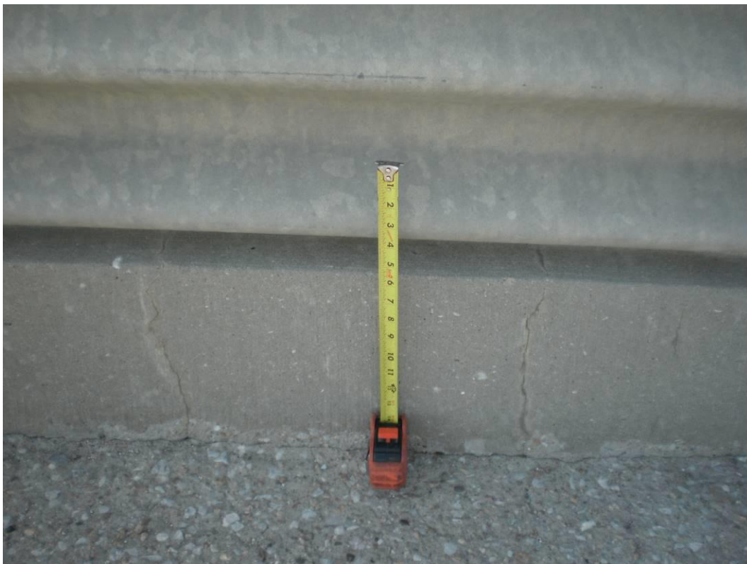
Photograph 80 – Vertical Cracks in the Curb
