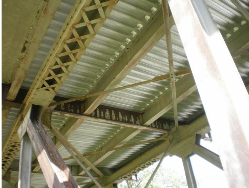
Photograph 14 – Rusted Areas on a Floorbeam
