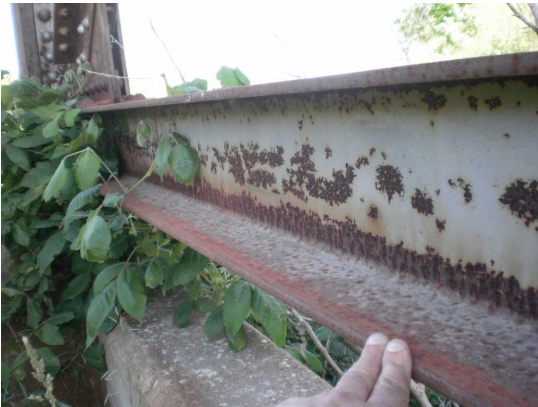
Photograph 32 – Typical Coating Condition on the Steel Bent Struts
