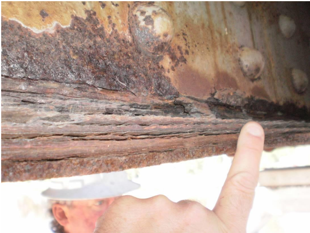
Photograph 51 – Delamination and Corrosion at Truss Bottom Chord
