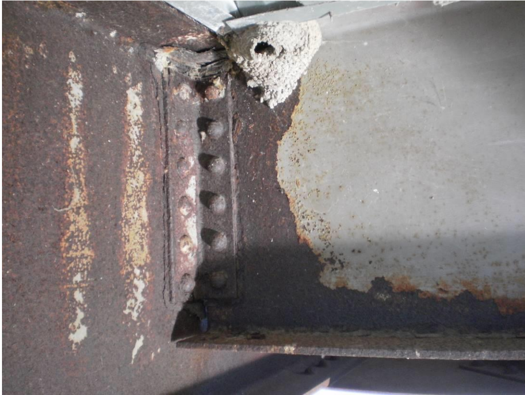
Photograph 54 – Coating Failure to Rust at Stringer to Floorbeam Connection
