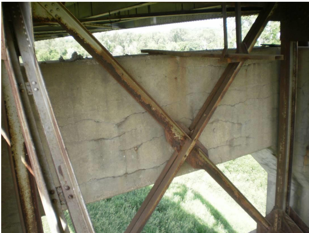
Photograph 70 – Cracks at Pier 6
