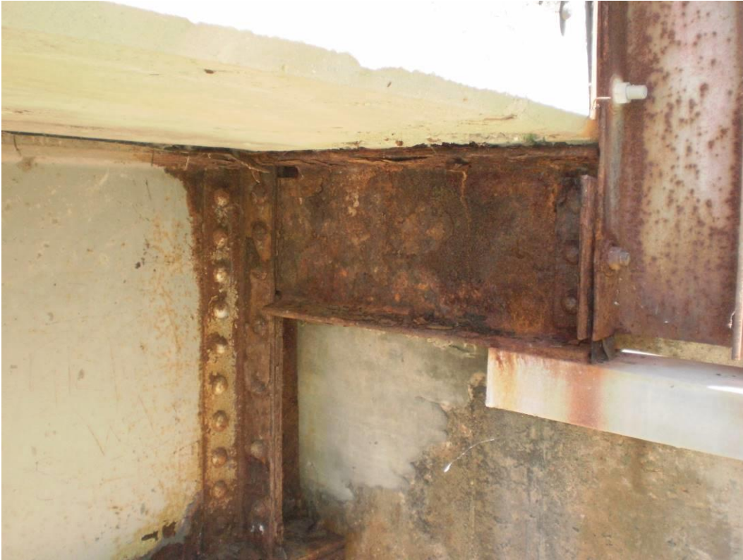
Photograph 31 – Corrosion and Section Loss on Guardrail Post Bracket at Abutment No. 2
