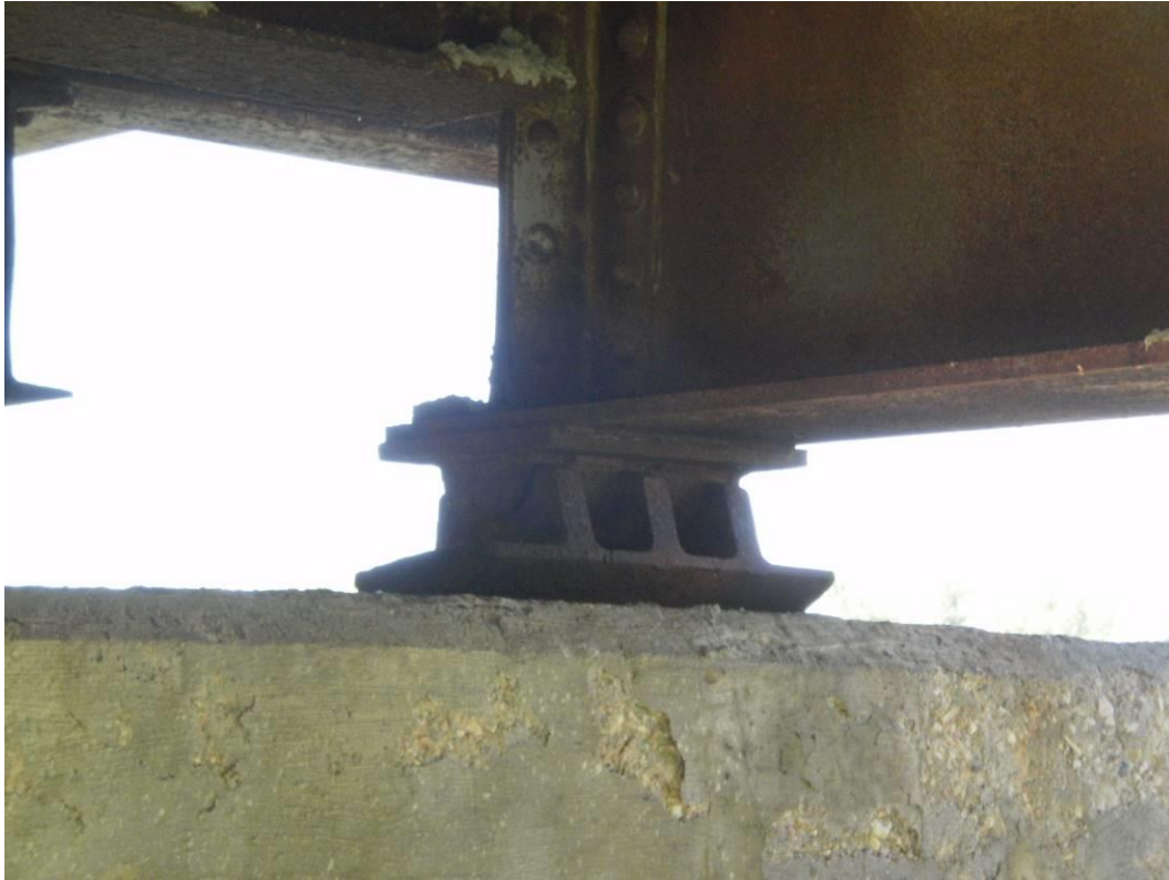
Photograph 23 – Typical Condition of the Bearings
