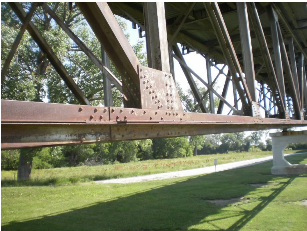
Photograph 7 – Typical Condition of More Environmentally Exposed Truss Members
