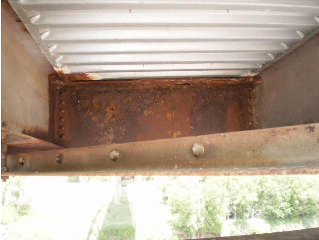
Photograph 48 – Corrosion and Section Loss on Intermediate Diaphragm
