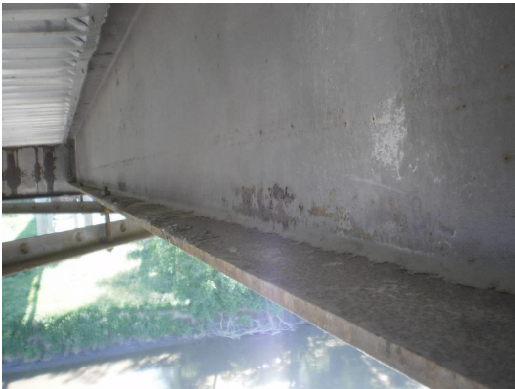
Photograph 53 – Rust along Stringer Bottom Flange
