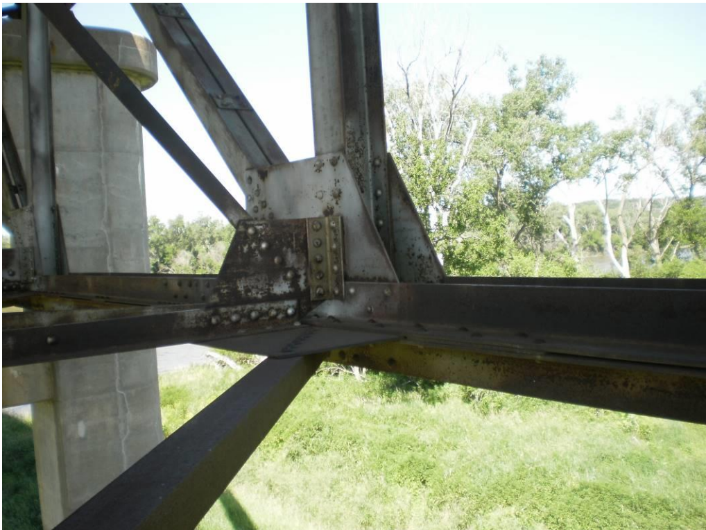
Photograph 19 – Typical Conditions at Bottom Chord Gusseted Connections
