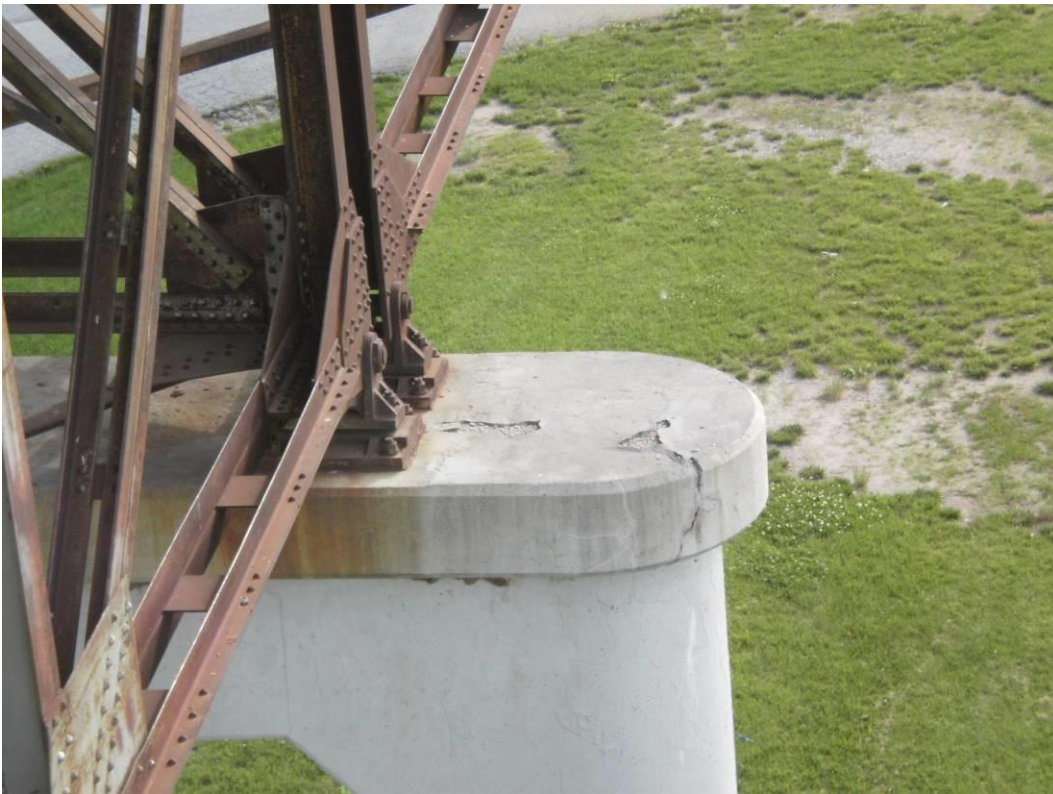
Photograph 66 – Chipped/Spalled Areas on a Pier Cap
