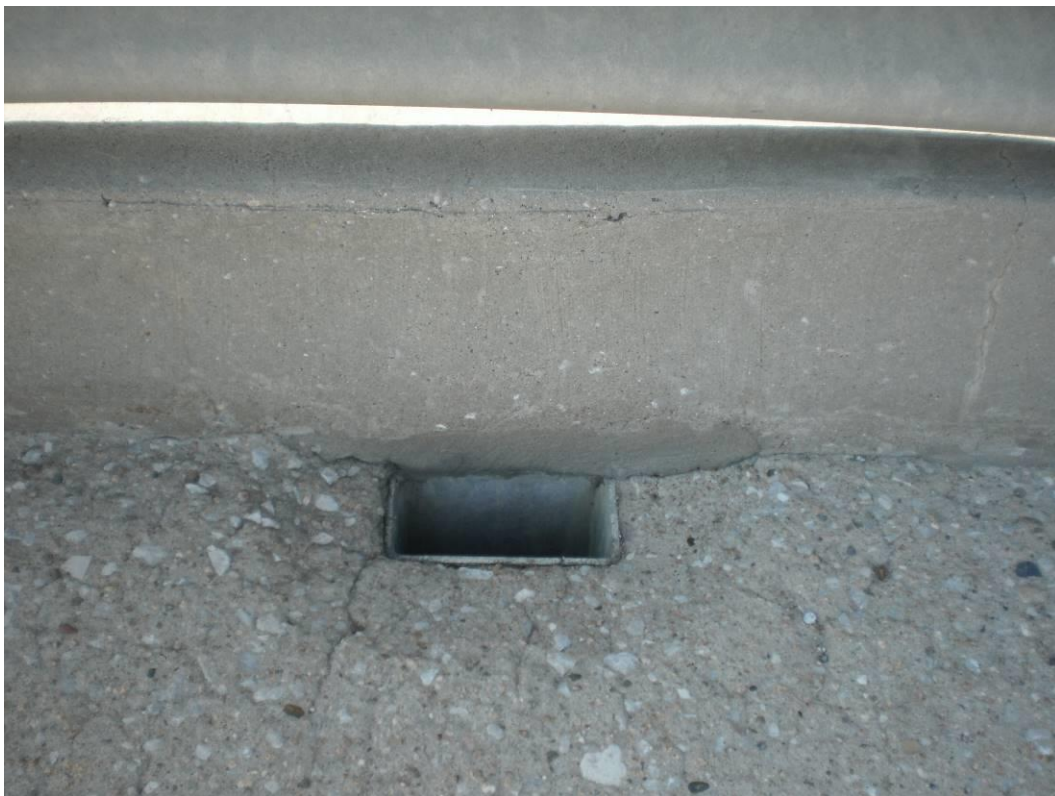
Photograph 82 – Crack in Deck at a Drain Inlet
