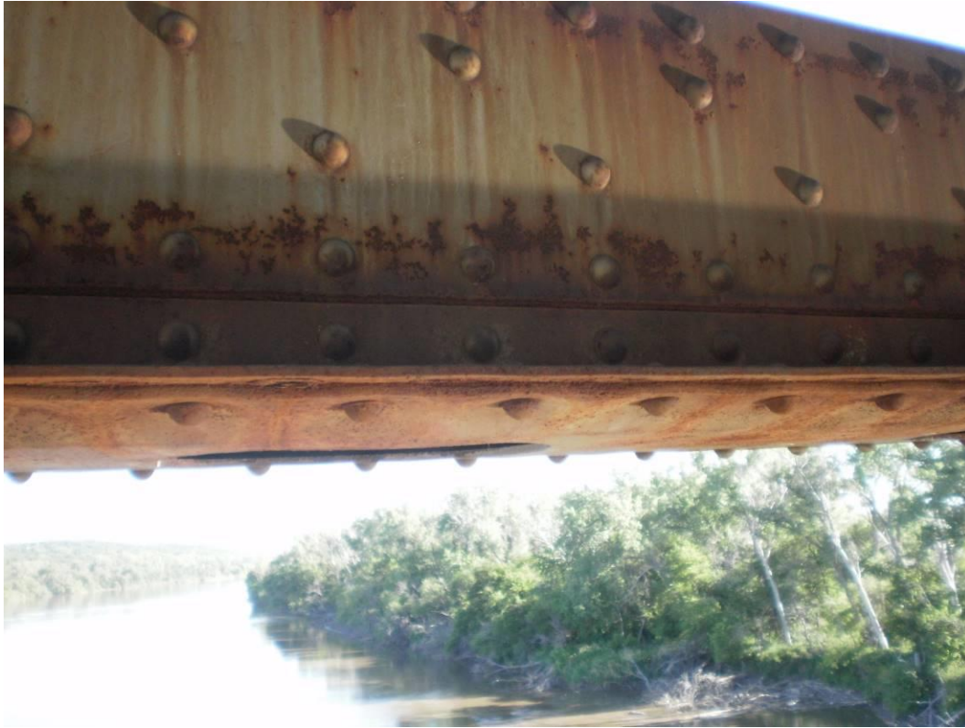
Photograph 2 – Span 6 Bottom Chord – Note Pack Rust Causing Curvature (distension) of the Bottom Cover Plate
