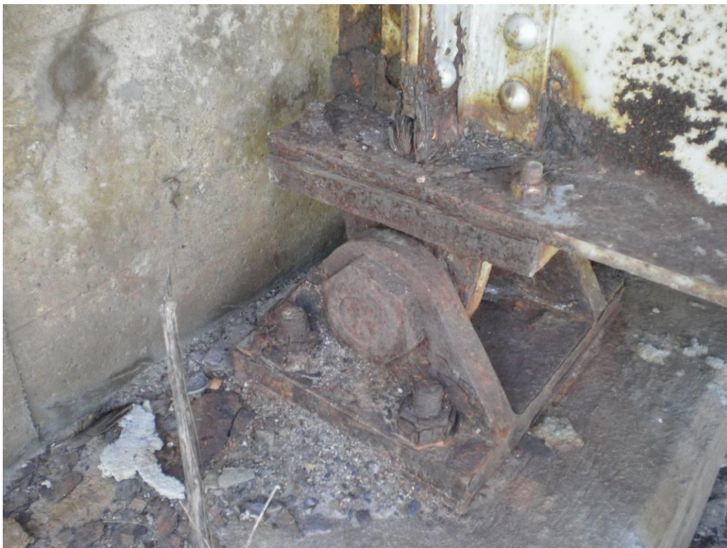
Photograph 24 – Corrosion at Abutment No. 2 Bearings – Note Section Loss on the Beam Bearing Stiffener
