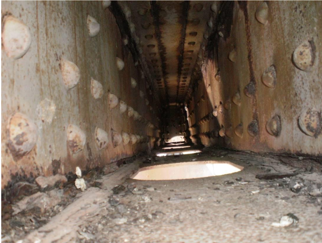
Photograph 50 – Interior of Bottom Chord in Distended Area – Note Pack Rust and Laminated Corrosion
