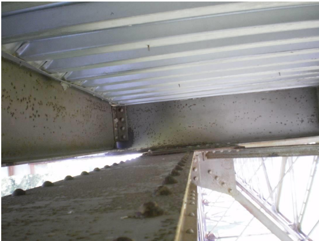
Photograph 5 – Rust Areas on Top of the Top Chord, Floorbeam, and Stringer
