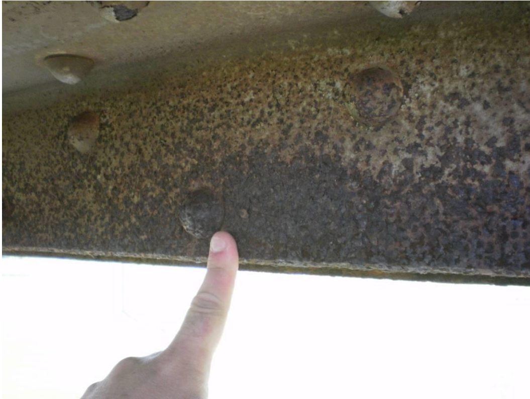
Photograph 8 – Typical Condition of the Bottom Chords
