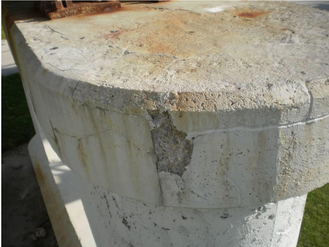
Photograph 61 – Area of Chipping at Previous Repair
