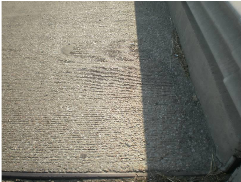
Photograph 78 – Exposed Aggregate along the Curb
