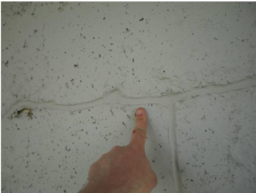
Photograph 62 – Typical Good Condition of Previous Crack Repair
