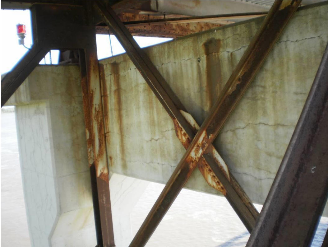
Photograph 67 – Horizontal Cracks in the Pier Cap at Pier 4
