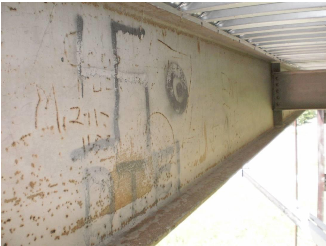
Photograph 30 – Graffiti on Beam at Abutment No. 2
