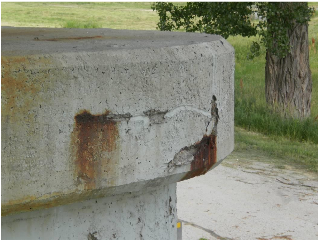
Photograph 64 – Chipped/Spalled Areas with Rust Stain (It was not determined if the stain was from reinforcing or form ties)
