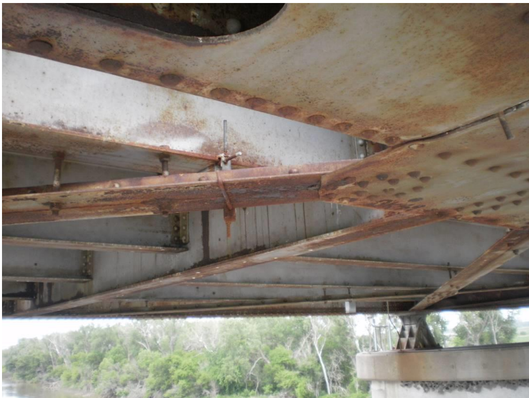
Photograph 47 – Corrosion on Lower Lateral Bracing
