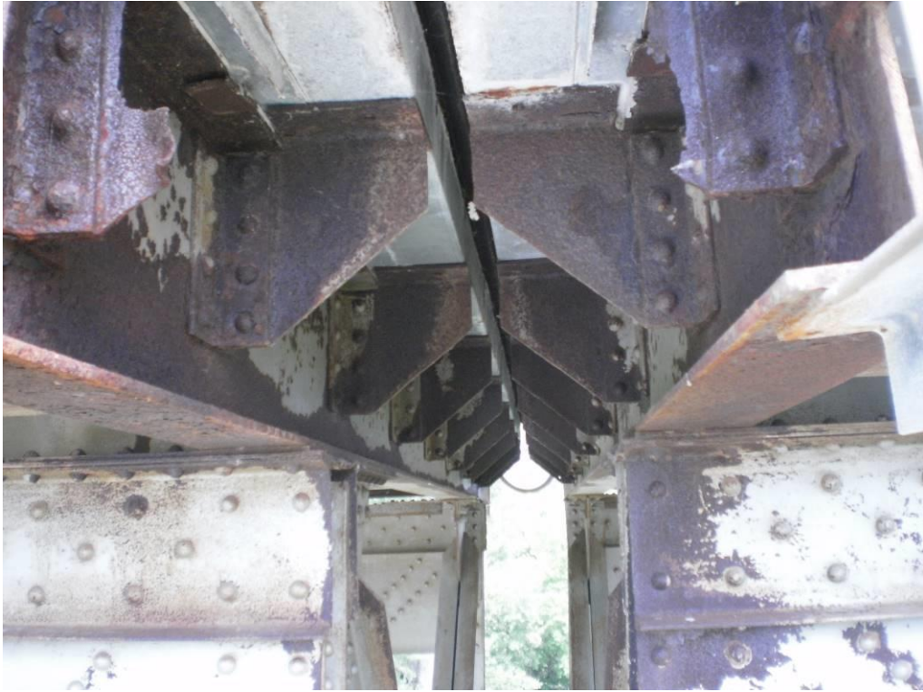
Photograph 18 – Overhanging Brackets at an Expansion Joint Note Bracket Rusted Away at the Top of the Photograph
