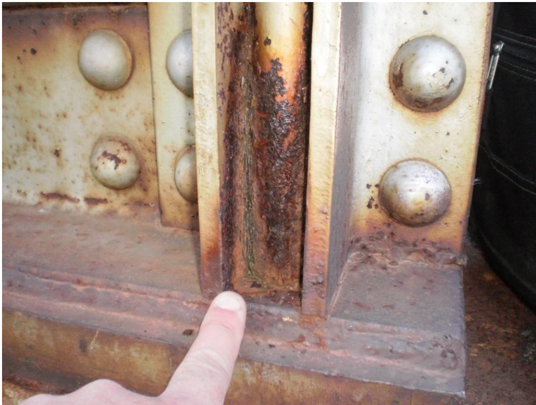
Photograph 33 – Typical Pack Rust at Bent Column Anchor Bolts
