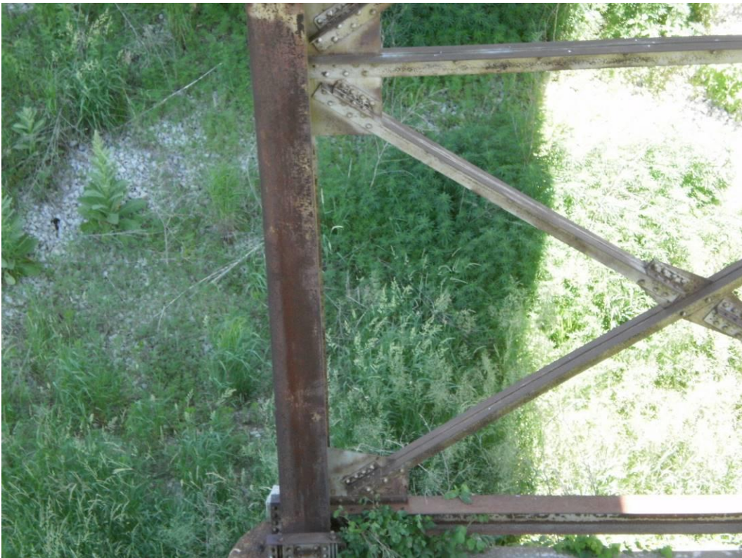
Photograph 28 – Areas where No Coating Remains on a Bent Column
