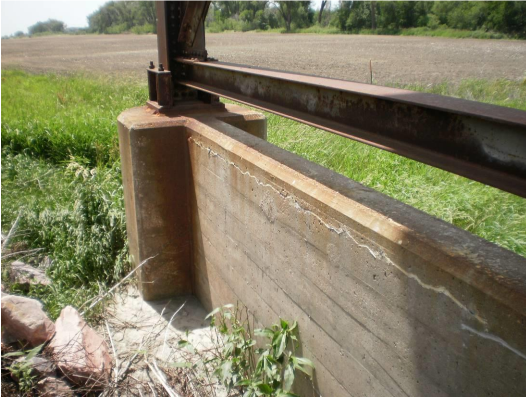
Photograph 73 – Typical Condition at Steel Bent Foundations
