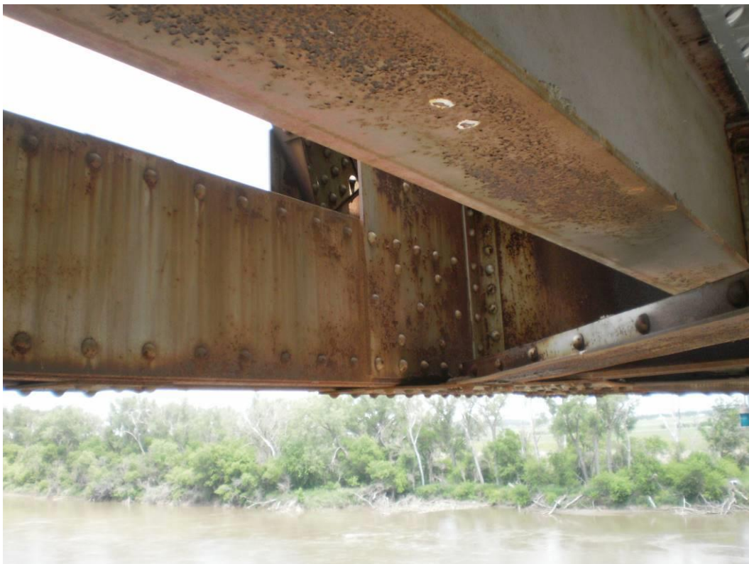
Photograph 43 – Corrosion Areas on Stringer Bottom Flange and Bottom Chord
