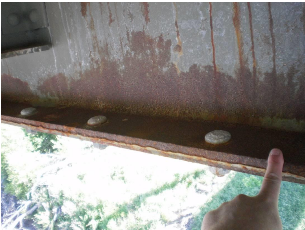
Photograph 57 – Corrosion on Upper Flange Surface at Floorbeam Cover Plate
