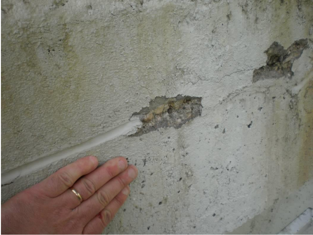
Photograph 63 – Minor Areas of Chipping/Spalling
