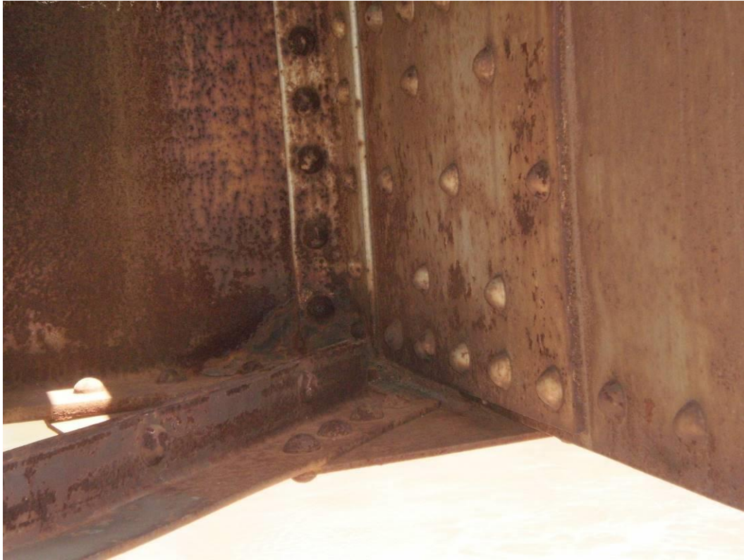
Photograph 46 – Corrosion at Lower Lateral Bracing Connection
