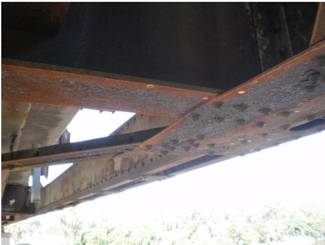
Photograph 59 – Rust on Bottom Chord Gusset Plate
