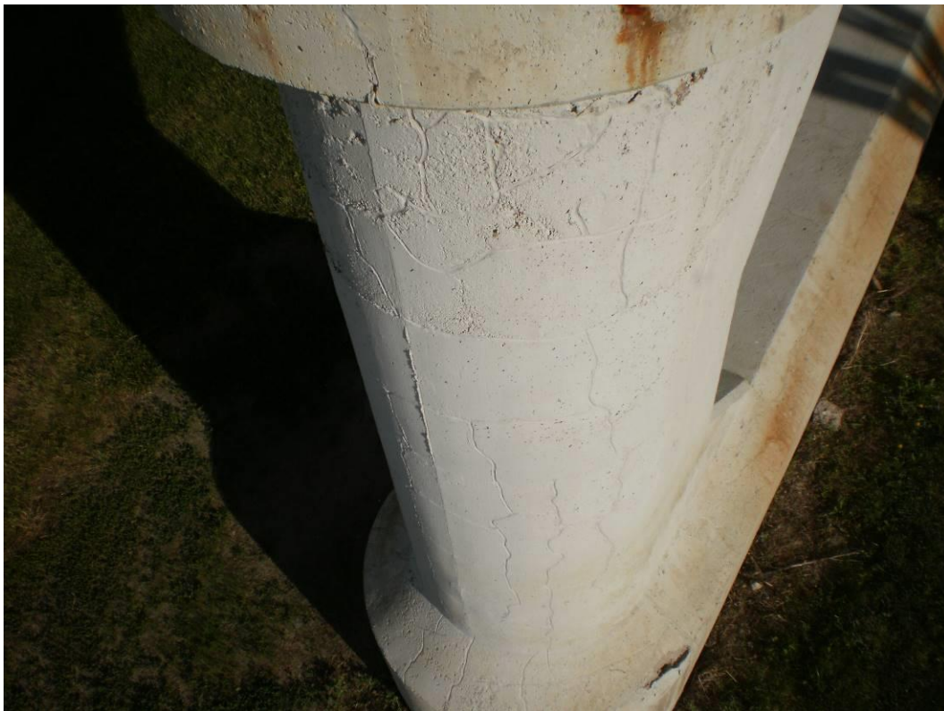
Photograph 60 – Painted Pier with Repaired Cracks – Note Chipping at Base
