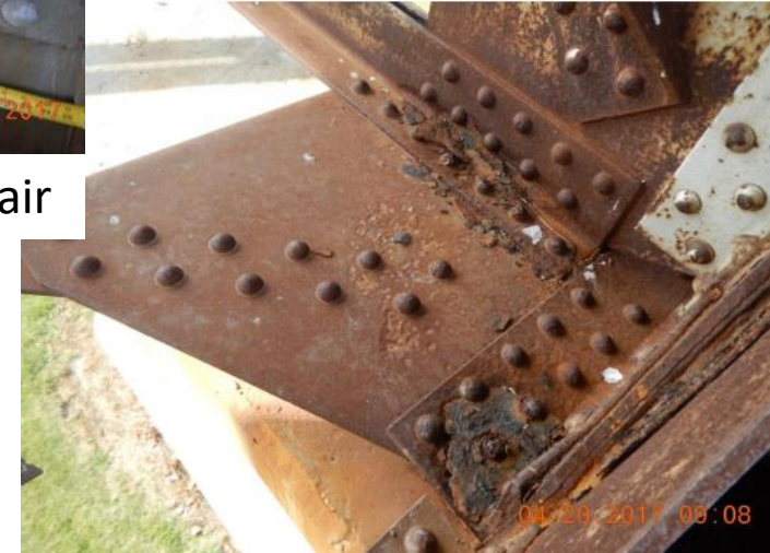
Typical Truss Gusset Plate Connection
