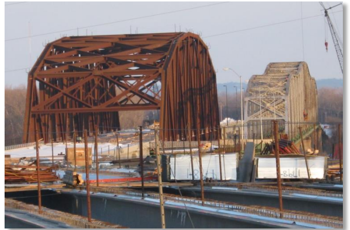
Construction of the new Veteran’s Memorial Bridge alongside the old bridge.
