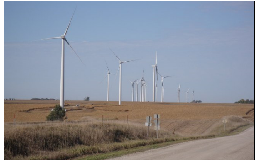
Walnut Wind Farm in Pottawattamie County, Iowa
