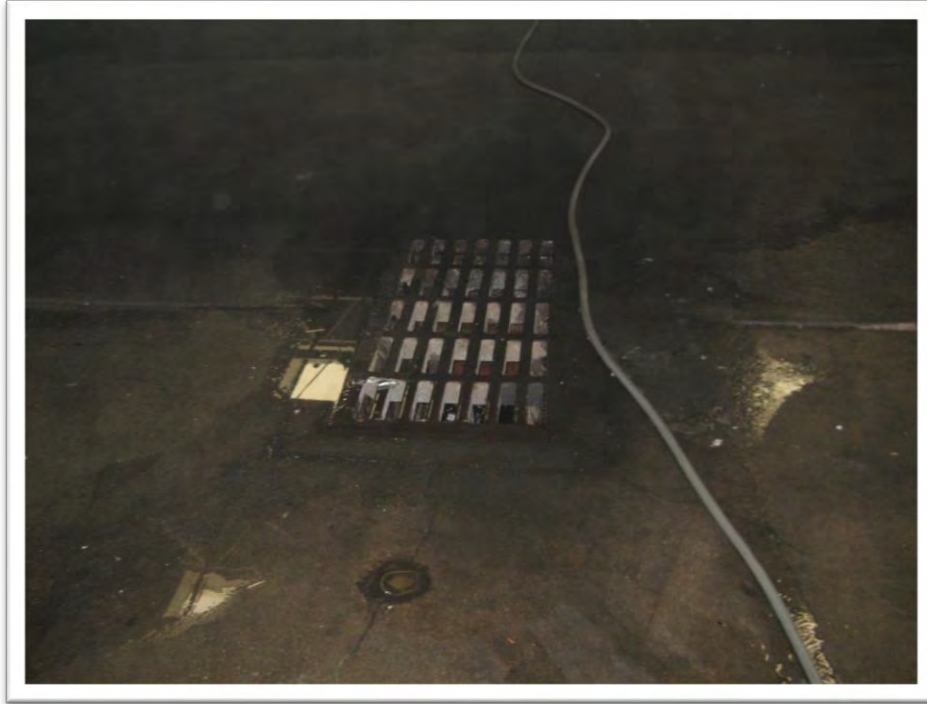
Floor drain located in center of warehouse floor.
