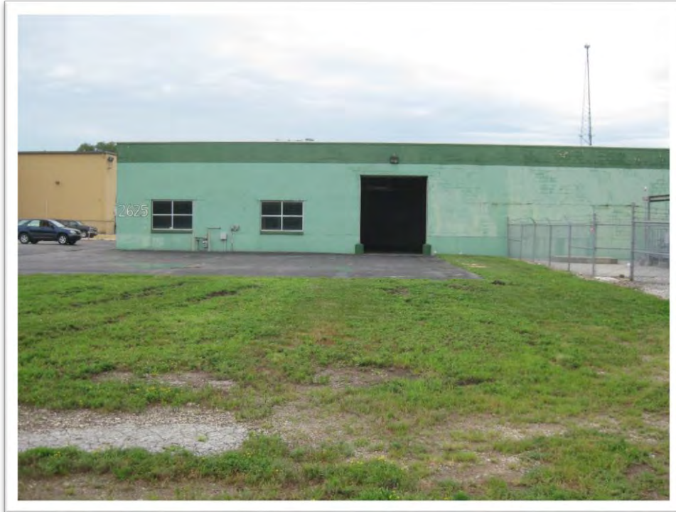
View south of building and lot east of the AT&T facility.
