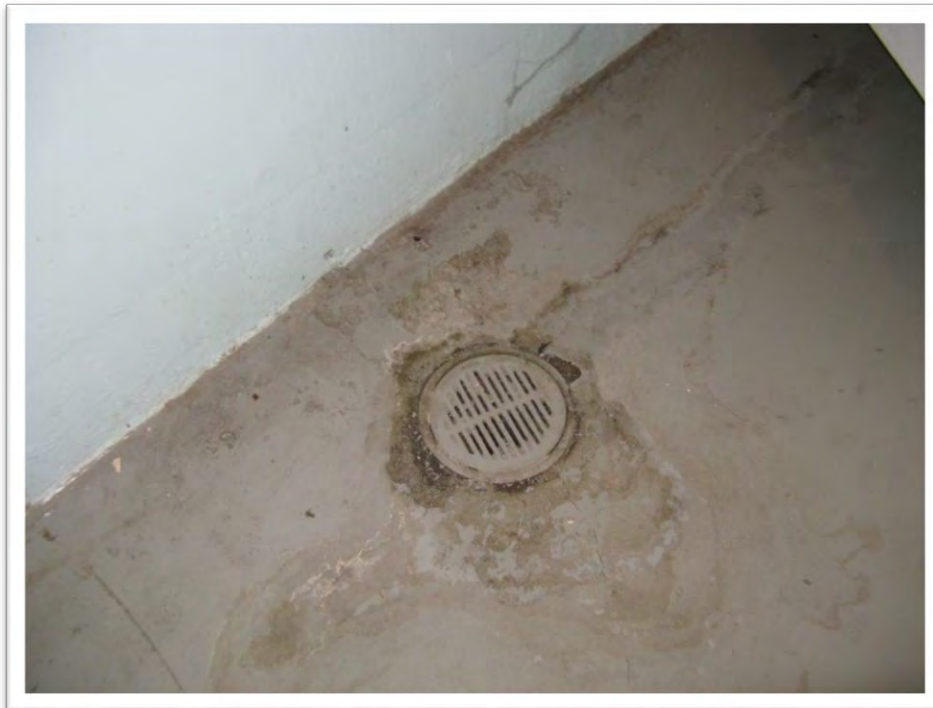
Floor drain located in the bathroom.
