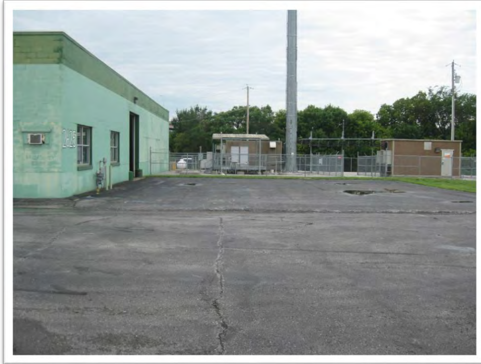
View west across Property towards AT&T facility.
