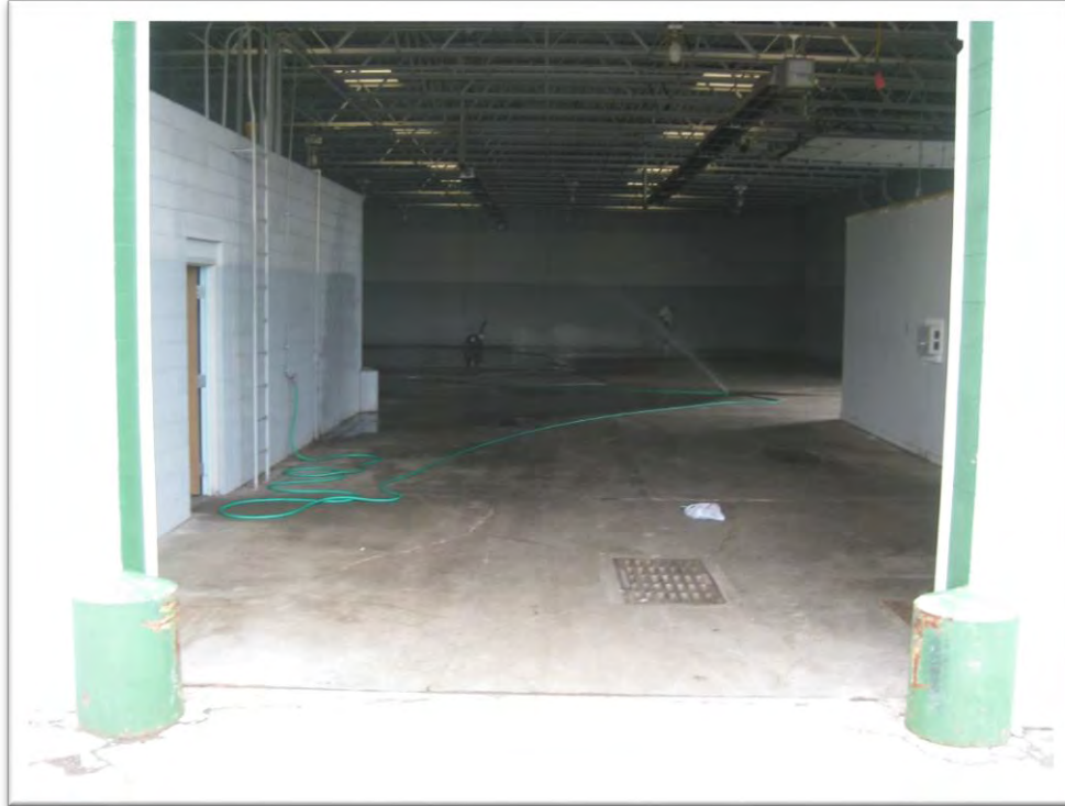
View into warehouse from east overhead entrance.
