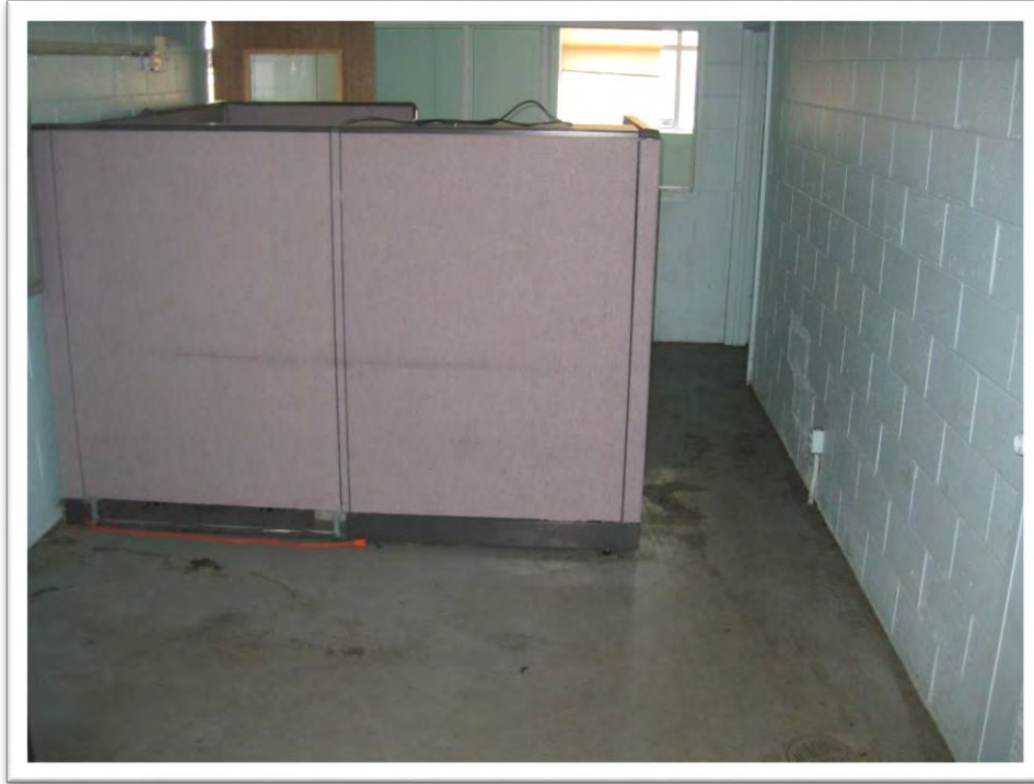
General view of office space in southeast corner of building.
