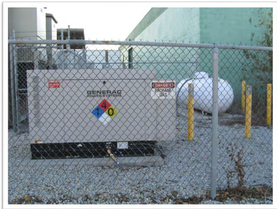
AT&T emergency generator with propane AST located near northwest corner of Property building.
