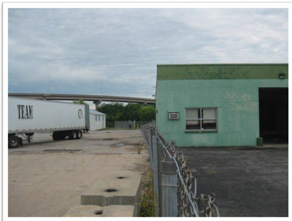
View west along south Property line.
