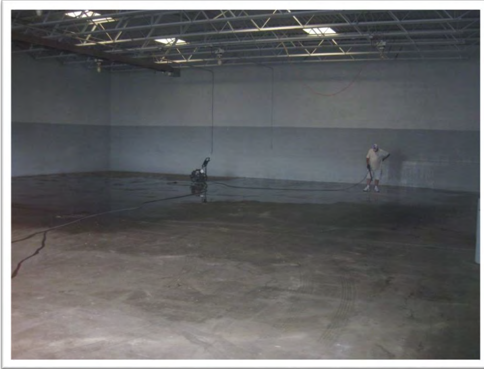
View of vacant warehouse area.
