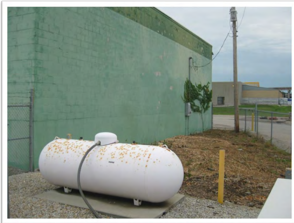
View along west side of building and propane tank.
