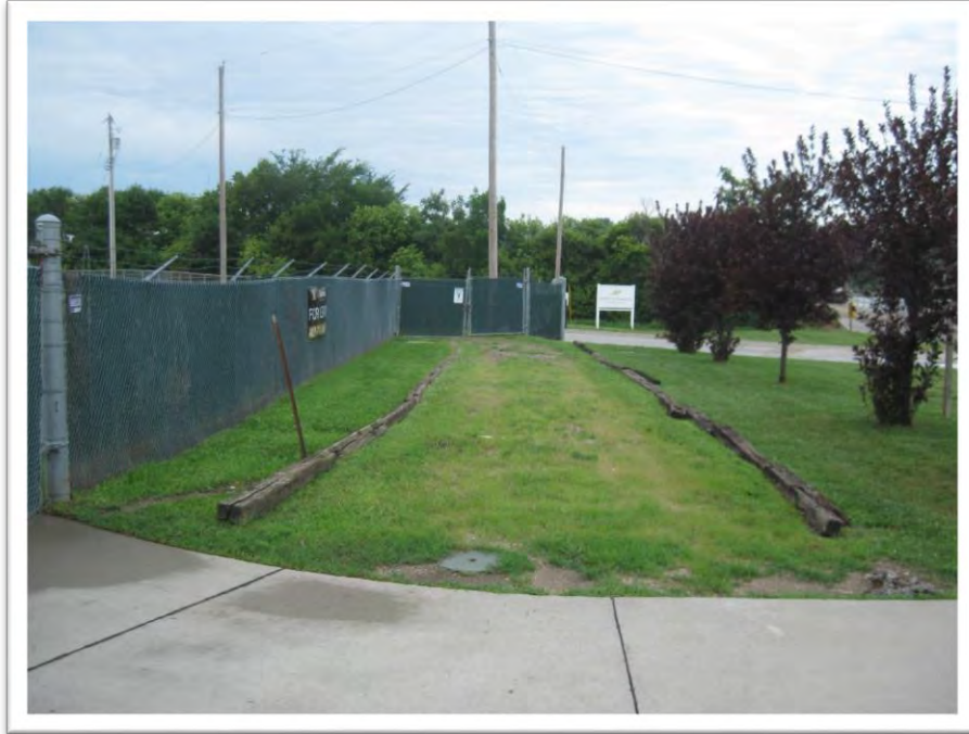
View west along cell tower access road next to fence and city right-of-way land located between the chain link fence (northern Property boundary) and Vinton Street.
