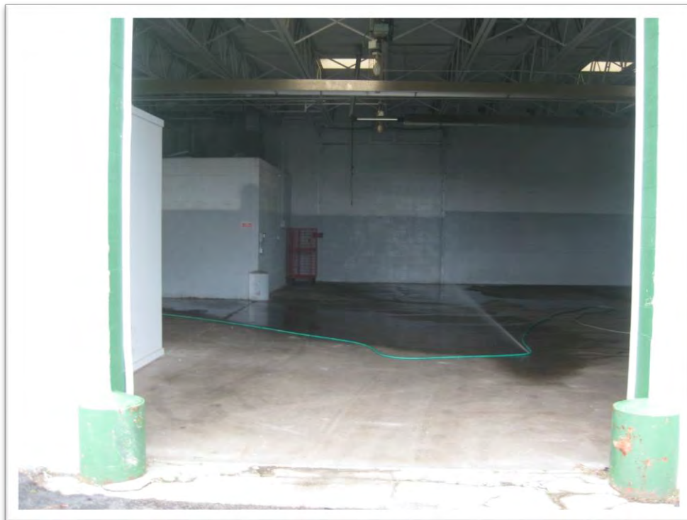
View into warehouse from north overhead entrance.
